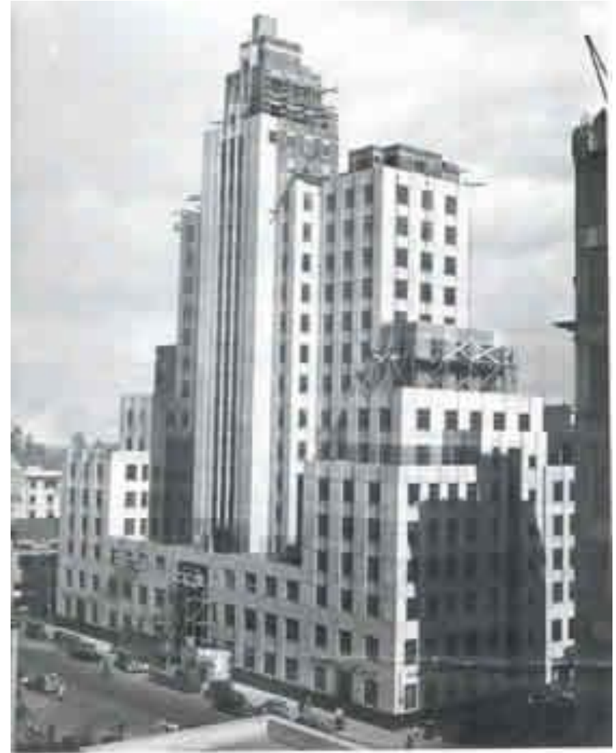
Escom House under construction
