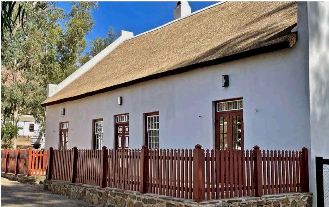
FIGURE 15B: The Winkelhuis front façade after restoration. (Image: ARCON, 9 March 2021).
