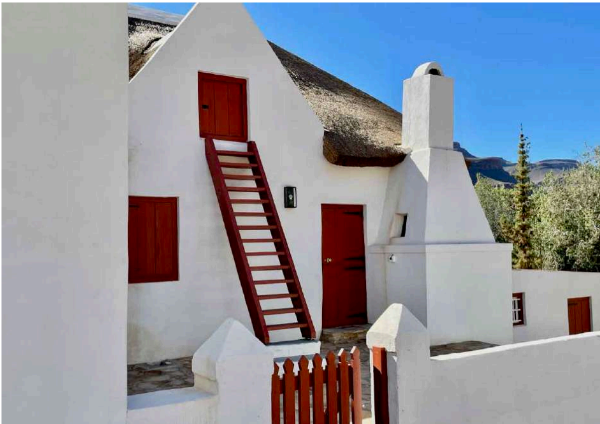
FIGURE 14F: The west side of the Parsonage after restoration. (Image: ARCON, 23 March 2021).
