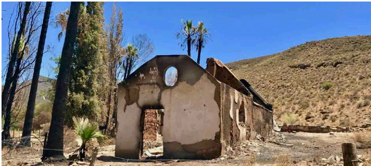
FIGURE 22A: The gutted Blacksmith's Shop after the fire. (Image: ARCON, 24 January 2019).
