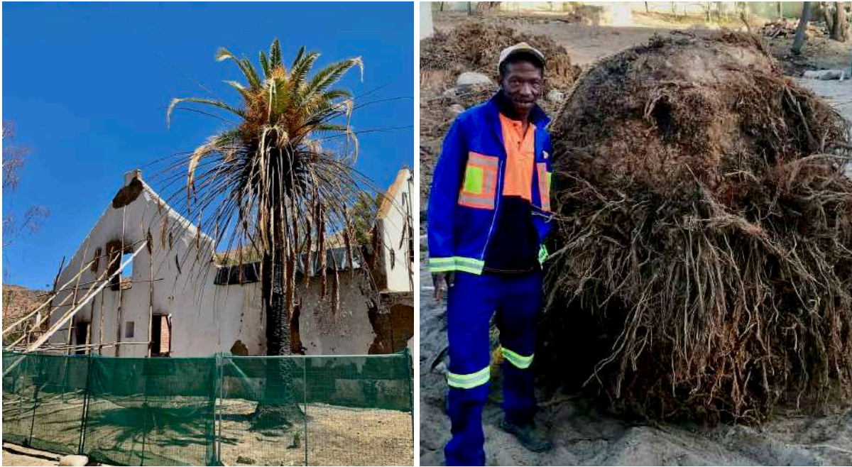
FIGURE 23C: Left: A palm next to the Winkelhuis was another example of a tree removed for fire security reasons. This image also indicates the emergency propping installed shortly after the fire using locally available timber to prevent a gable collapse. Right: the size of the root bowl of the palm after its removal. (Images: ARCON, 24 February 2019 and 11 October 2019).
