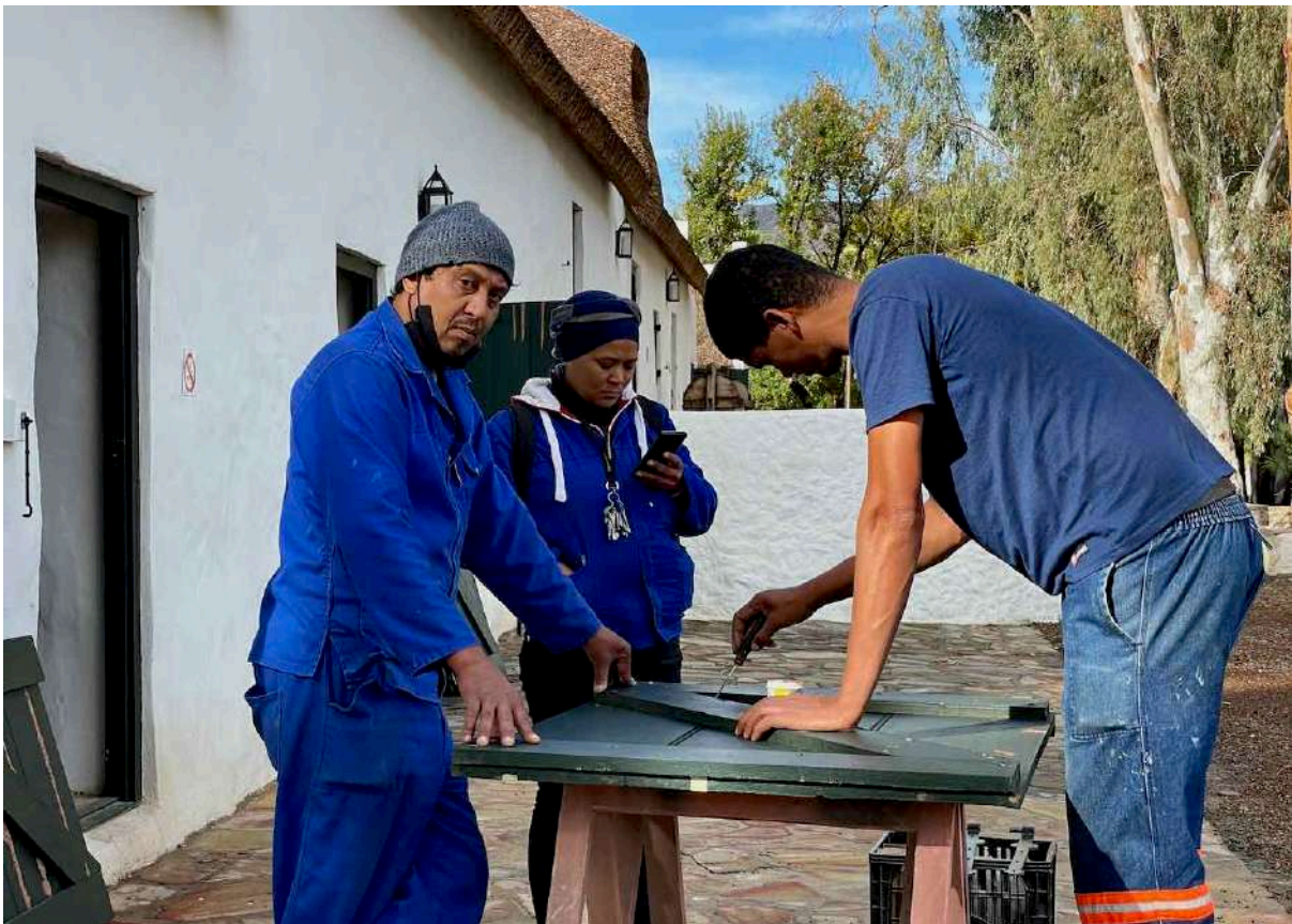
8 June 2021: Hanging new doors at Leipoldt House.
