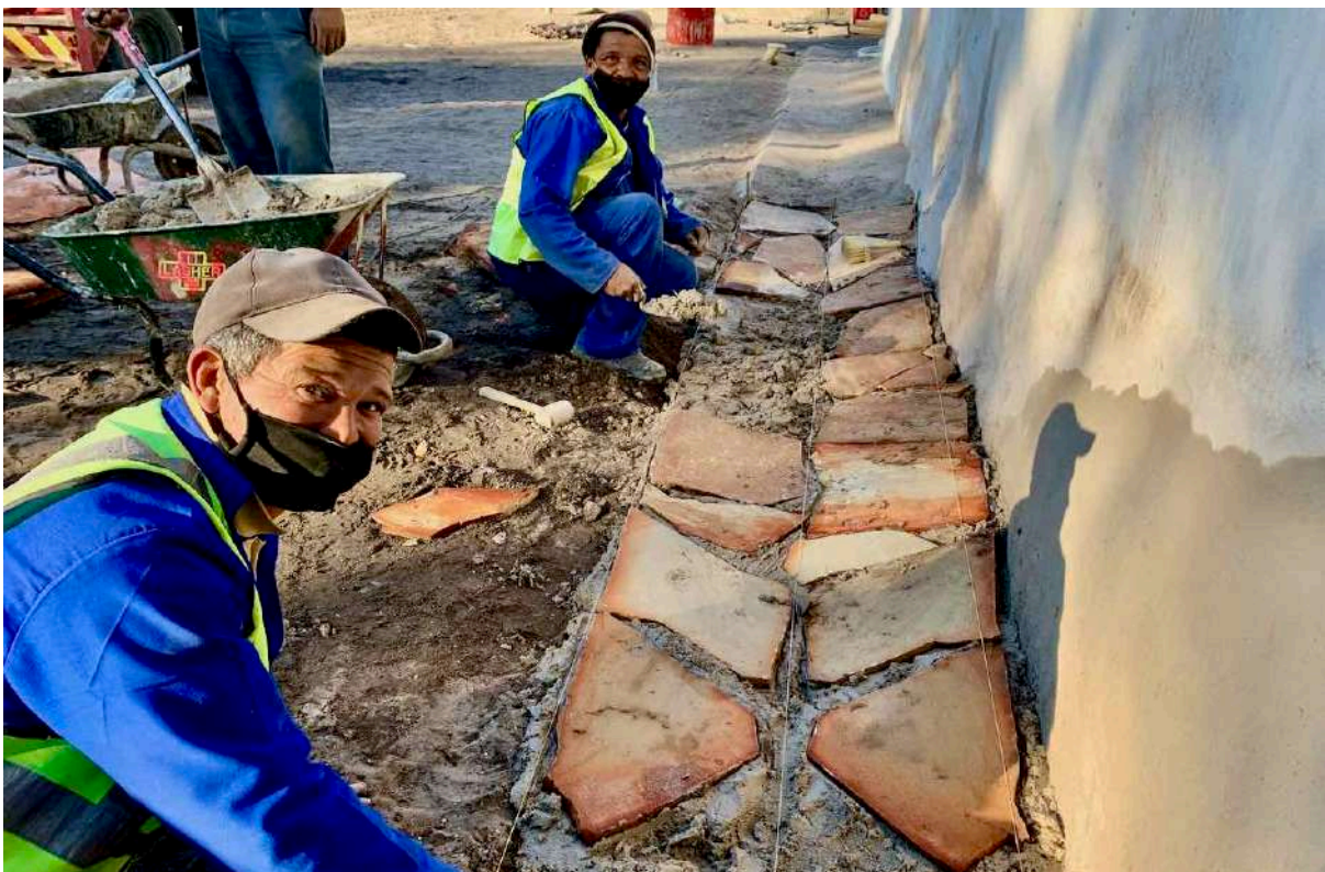
6 August 2020: Laying new rainwater channels for Leipoldt House.
