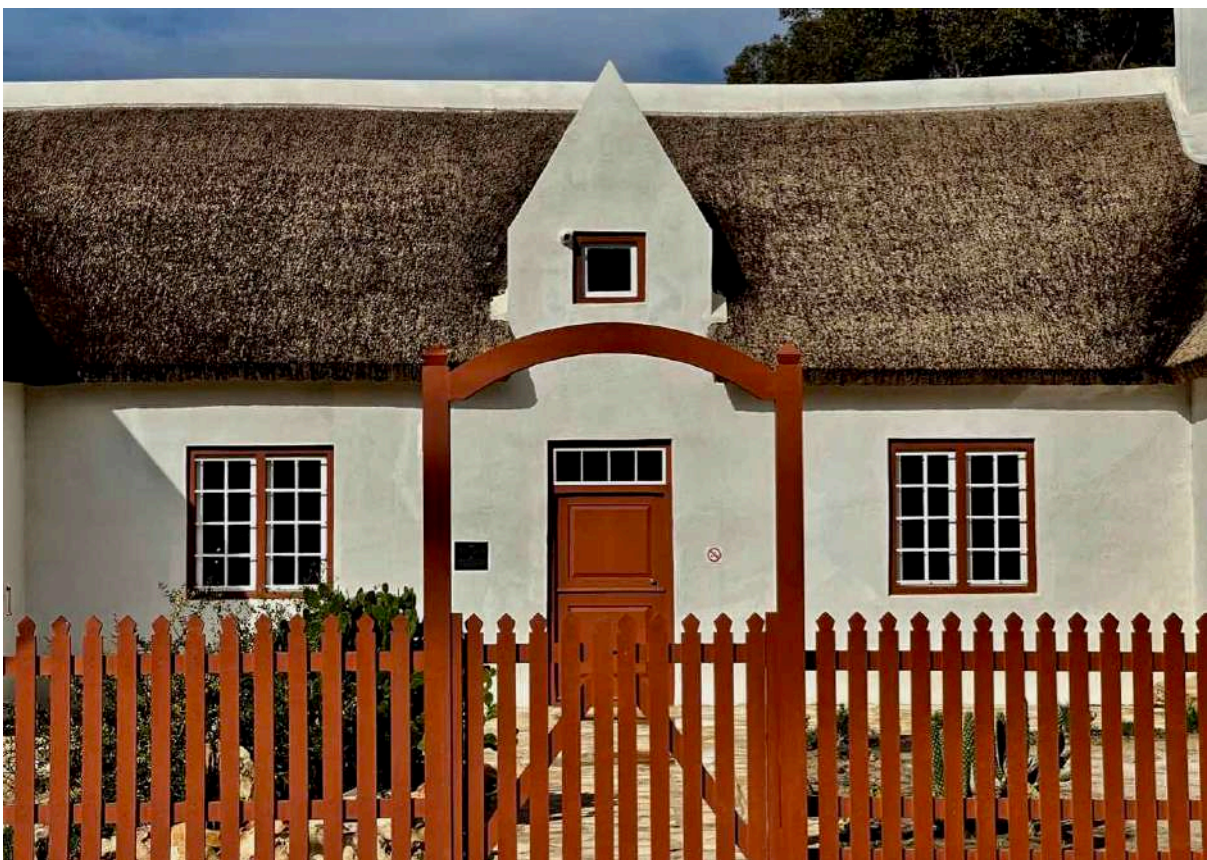
FIGURE 14D: The front façade of the Parsonage after restoration. (Image: ARCON, 8 June 2021).
