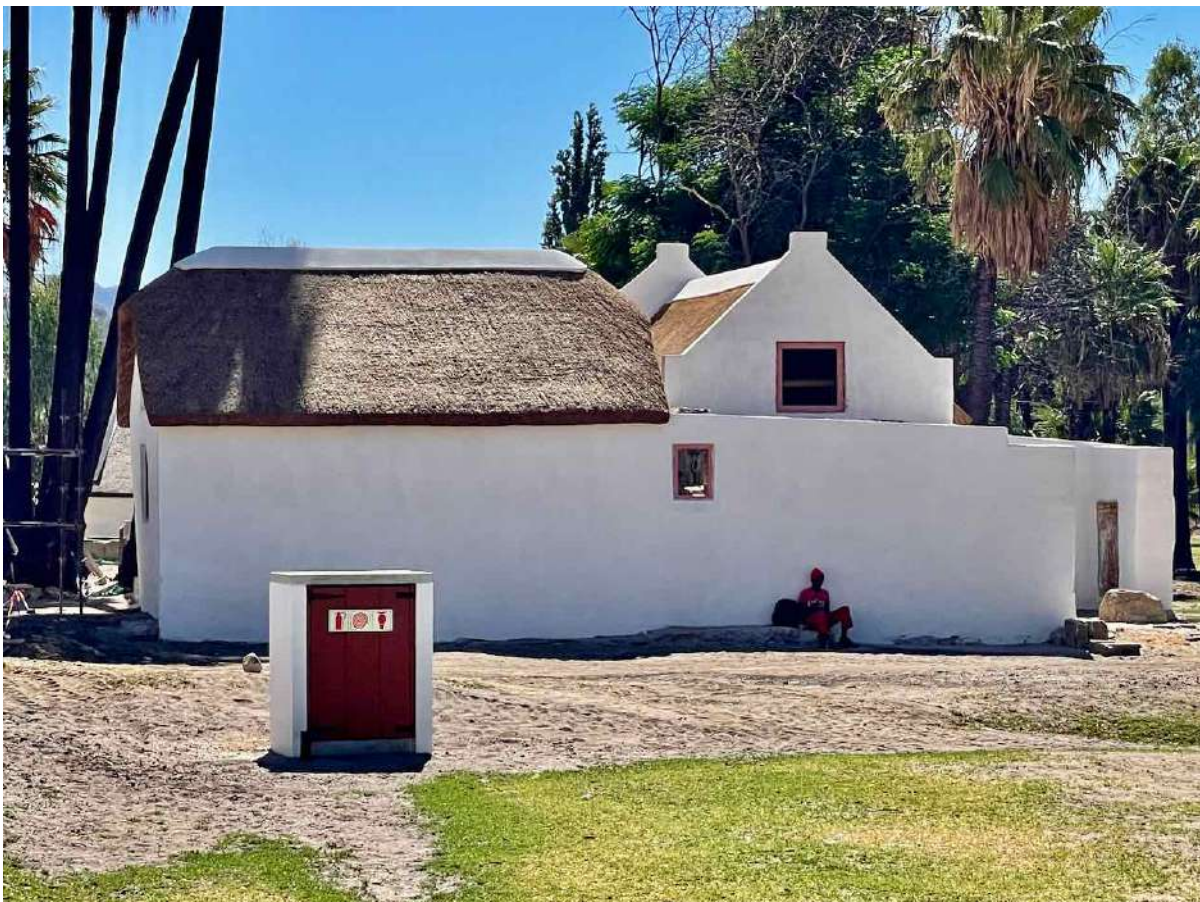
FIGURE 23D: Typical example of a fire hydrant kiosk. These enclosures were scaled to respond to the simple architecture of the precinct while being as visually unobtrusive as possible. (Image: ARCON, 23 February 2021).
