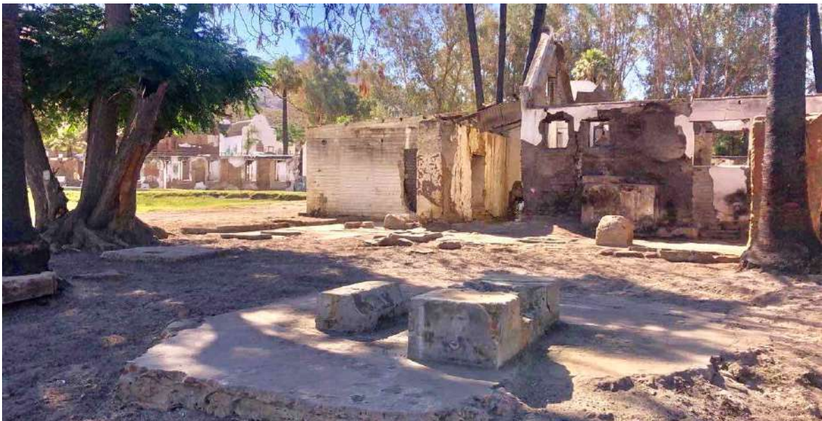
FIGURE 19C: View of the back (southwest end) of the fire gutted shell of the tannery. The fabric on the extreme left comprised the remains of a shallow mono-pitch extension which has stylistically latter 1950's/1960's bagged and horizontally raked 1 brick thick walls constructed with cement mortar. The burned out shell of one of the school hostels is visible in the background to the extreme left. The cement and concrete slabs and bases in the foreground once formed part of the now defunct tanning operation. These elements were finally removed after the project archaeologist gave the go-ahead. The concrete tanning tanks (not visible in this image) were retained. (Image: ARCON, 6 December 2019).
