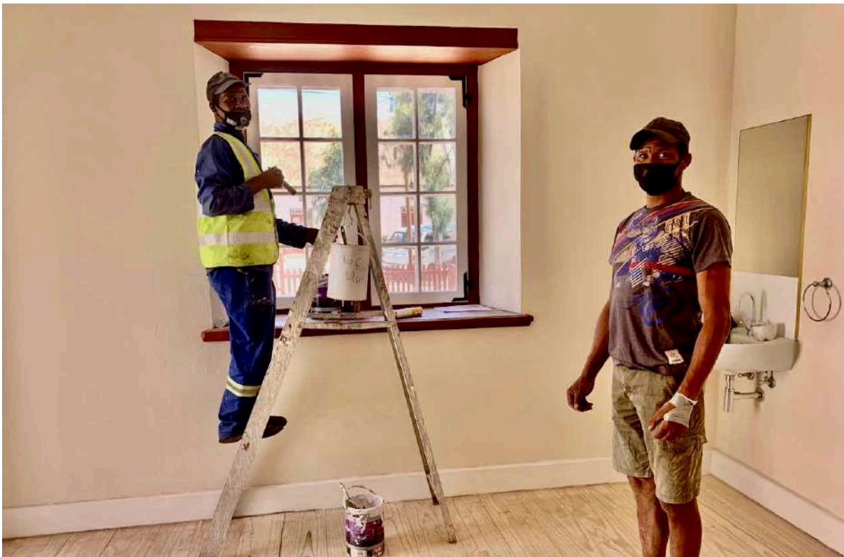
14 January 2021: Finishing work inside the Old Parsonage.
