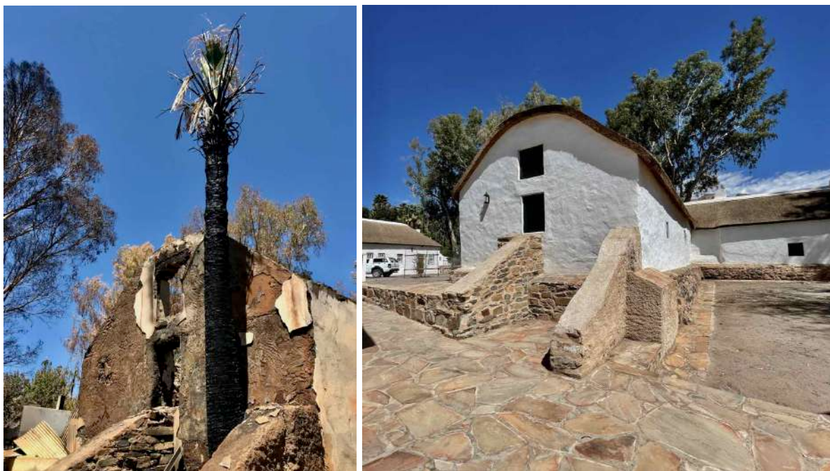
FIGURE 23B: Palms were likely the most instrumental in spreading the fire in the Church Precinct due to the aeration imparted by the shape of their fronds. Although palms strongly characterize the precinct, these and other trees close to the thatch buildings had to be removed as a precaution against the spreading of future fires. This example would have been at least partly responsible for the gutting of Leipoldt House. Its removal was debated at the time because of the risk its removal posed to the foundations of this historic building. Ultimately, it was removed and a small buttress constructed to reinforce the base of the wall in its place. (Images: ARCON, 24 February 2019 & 23 March 2021).
