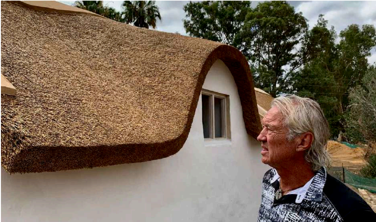
27 January 2020: Thatching contractor checking work at the Blacksmith's Shop.
