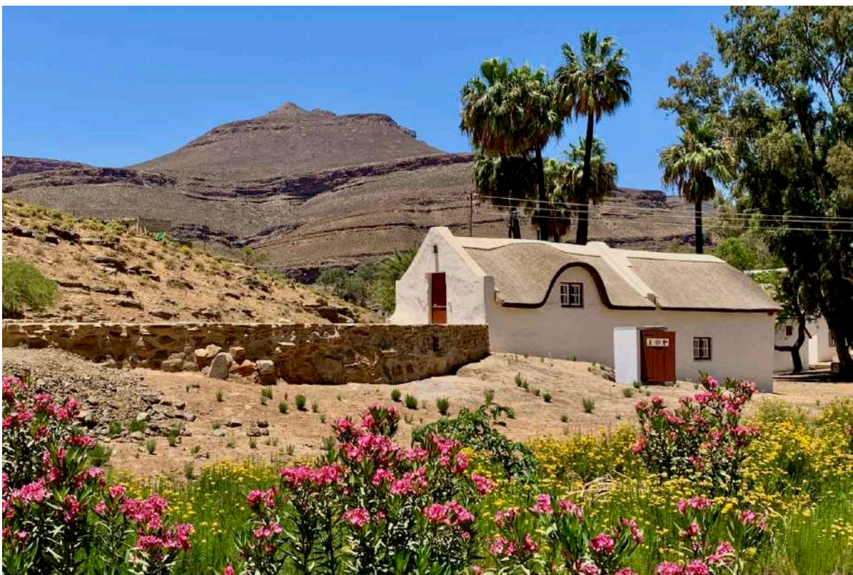
FIGURE 22F: The Blacksmith's Shop with threshing floor on the left and a fire hydrant kiosk to its right. It was not initially intended to restore the threshing floor but it was in such bad condition that the Foundation agreed to include it in the program. The roof dormer is a new insert to provide natural light to an otherwise dark upper level after it was decided to use the building as the town's information centre. (Image: ARCON, 23 February 2021).
