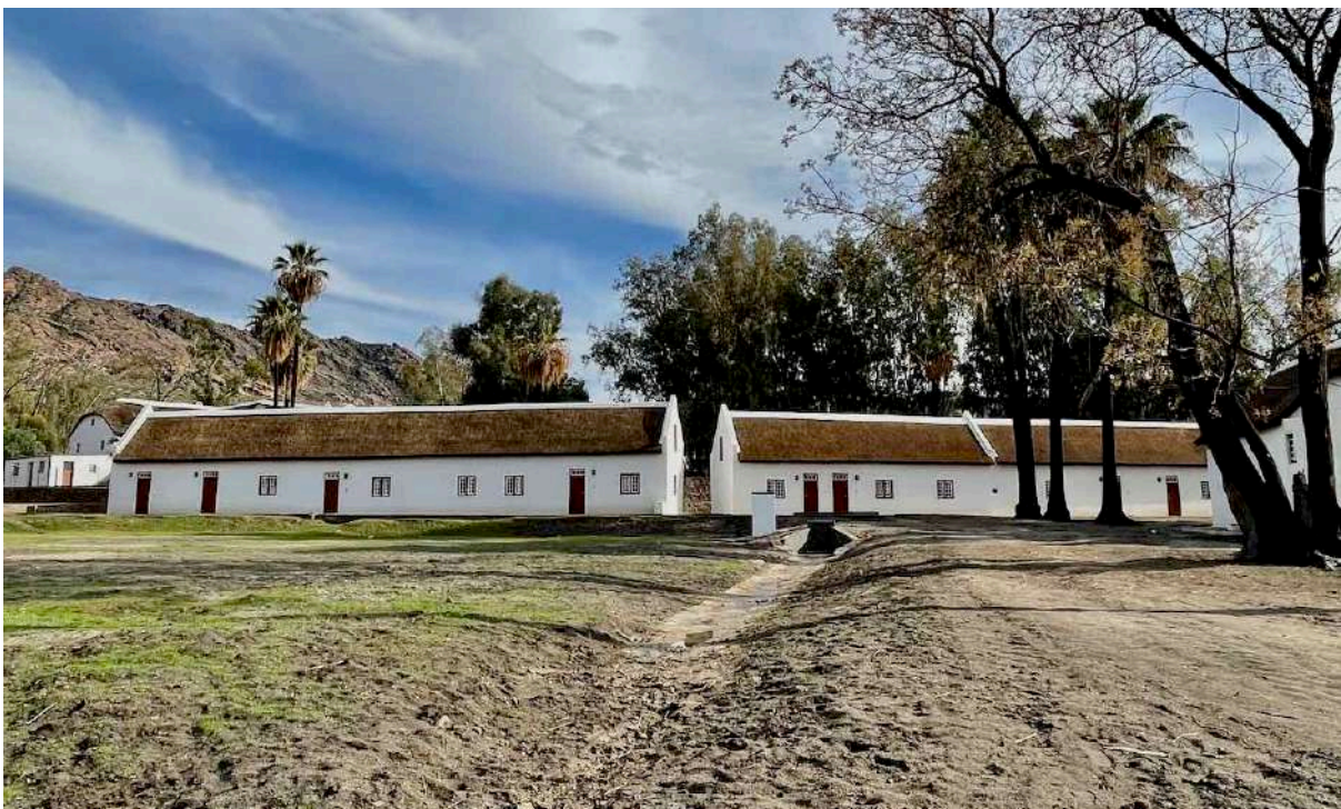
FIGURE 20F: View of both restored hostel buildings, now repurposed as guest accommodation for the village. The channel and outfall in the center of this image is part of a new stormwater system installed by the Foundation to control flood waters which had previously been a problem, after heavy rains. (Image: ARCON, 4 May 2021).
