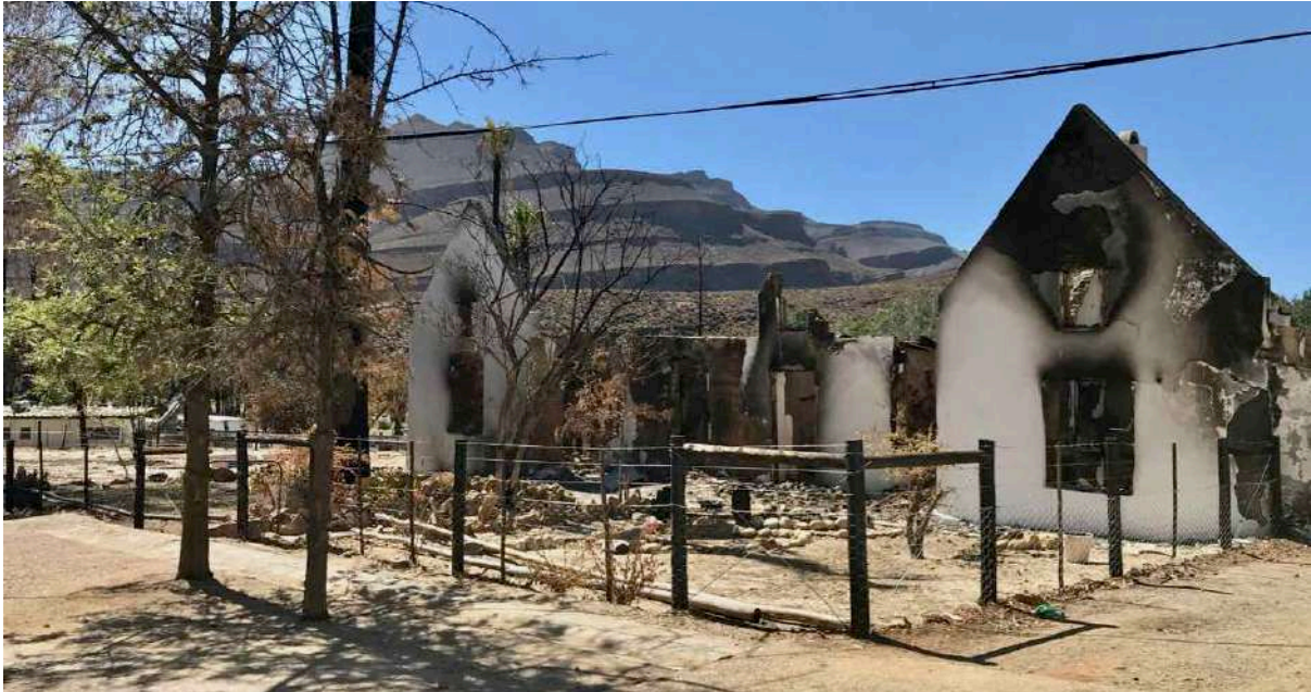
FIGURE 14A: The Parsonage after the fire. (Image: ARCON, 24 January 2019).
