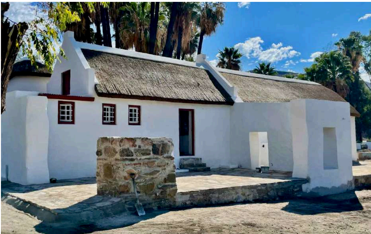
FIGURE 19E: View of the back of the tannery after restoration for use as guest accommodation. The new stone structure in the foreground is a braai. Most of the concrete bases in Figure 19D were retained under the new stoep. (Image: ARCON, 4 May 2021).
