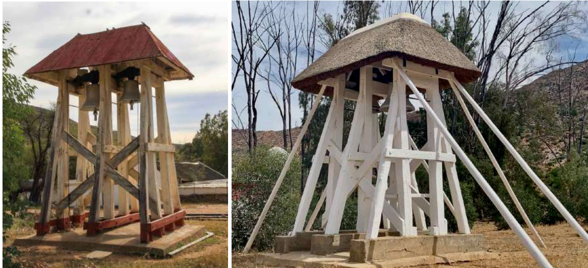
FIGURE 24A: The campanile behind the church. Left: before refurbishment. Right: the campanile after refurbishment. The stays had been added by the locals at some stage after the 2009 photograph on the left and did not form part of the restoration project. (Image left: Gabriel Fagan Architects, 22 September 2009; right: ARCON, 27 October 2020).
