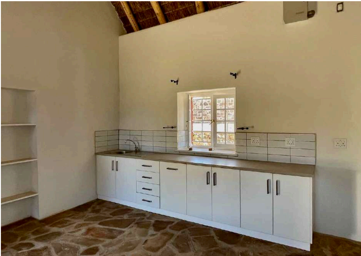
FIGURE 20E: Kitchenette in one of the guest flatlets. Door openings that were bricked in were left recessed as a record of that opening, and to double as shelf space. (Image: ARCON, 4 May 2021).
