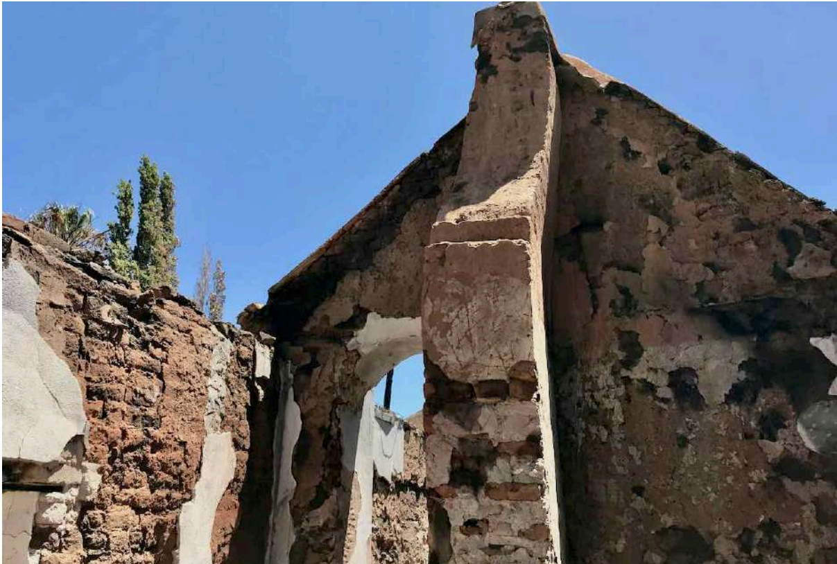
FIGURE 22C: The remains of the forge flue after the fire. (Image: ARCON, 24 January 2019).
