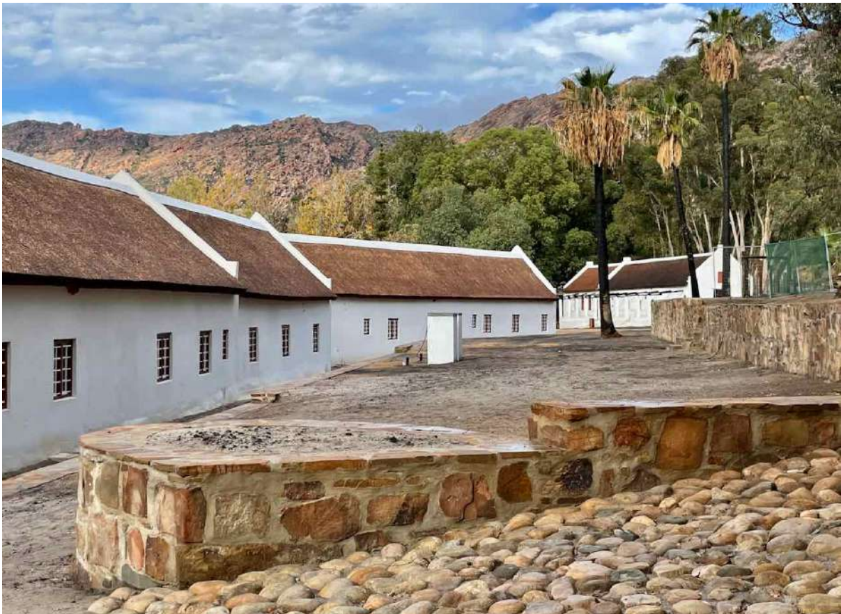
FIGURE 26F: Reconstructed stone walls behind the restored Hostel Buildings (left). The Shoe Factory is in the background to the right. (Image ARCON, 8 June 2021).
