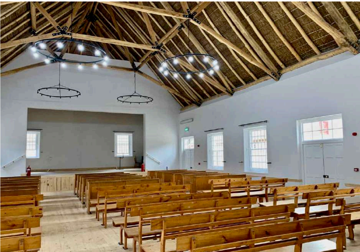
FIGURE 11D: The interior of the Community Hall after restoration was practically complete. The roof trusses are a more rustic re-design of the destroyed originals, which had been made of uniformly turned members. The simple chandeliers were specially designed for the interior. (Image: ARCON, 9 July 2020).
