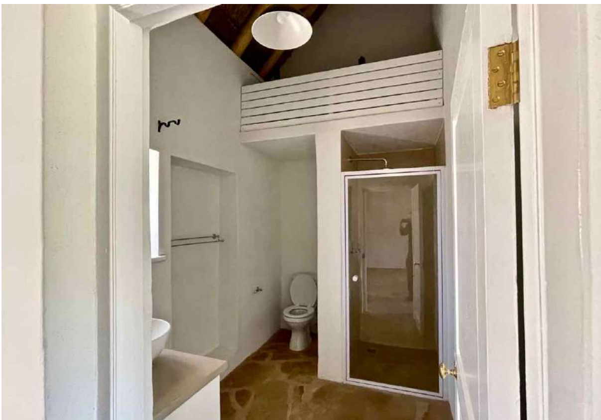
FIGURE 20D: Part of the same interior, now a bathroom for one of the new guest flatlets. Where window openings were bricked in, the infill brickwork was recessed as a record of that opening. Stone for the new floors was all locally sourced. (Image: ARCON, 18 May 2021).
