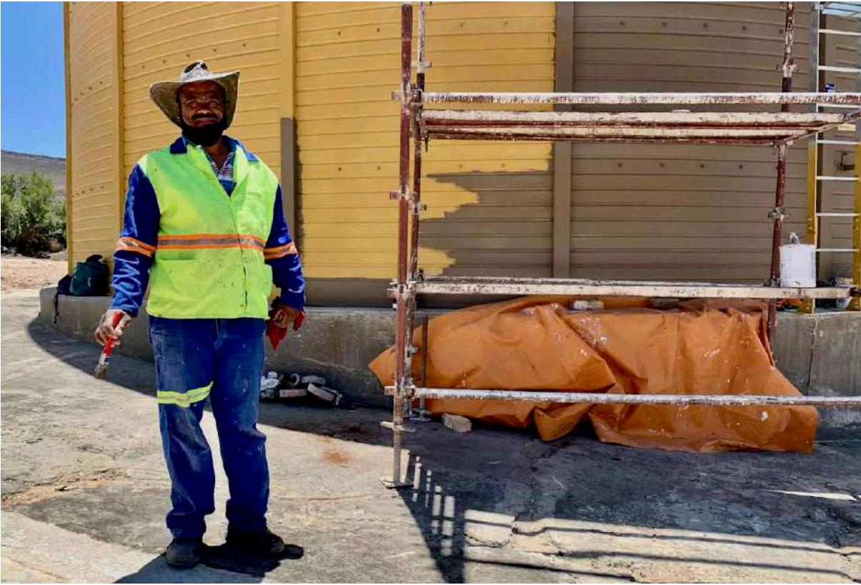
14 January 2021: Painting the town's new water reservoir.
