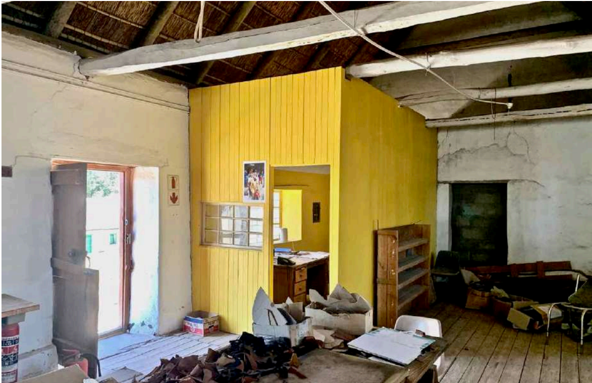
FIGURE 18B: Interior of the Shoe Factory before refurbishment. (Image: ARCON, 17 March 2020).
