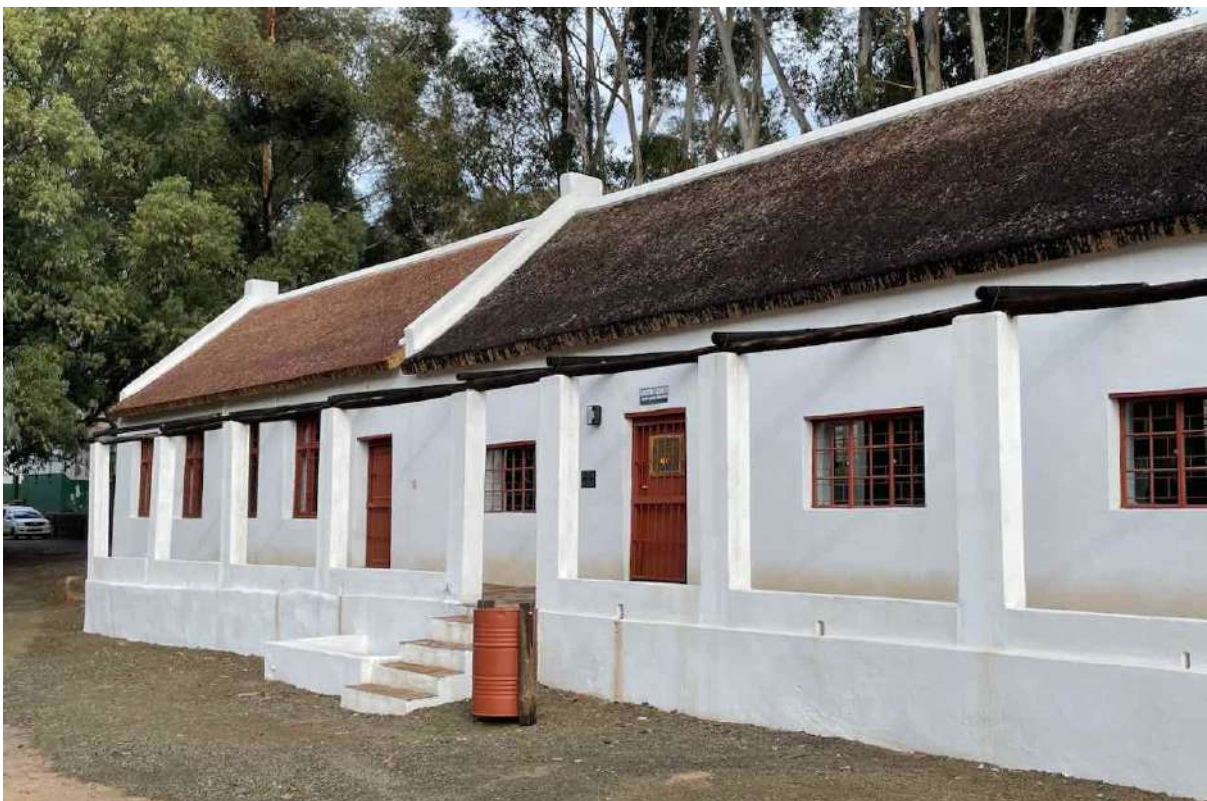
FIGURE 18E: Exterior of the Shoe Factory after refurbishment. The extension on the far left was provided with a thatched roof to match the roofscape of the rest of the town centre. The interior was refurbished to provide a shop for the factory. The steel windows were retained. (Image: ARCON, 8 June 2021).
