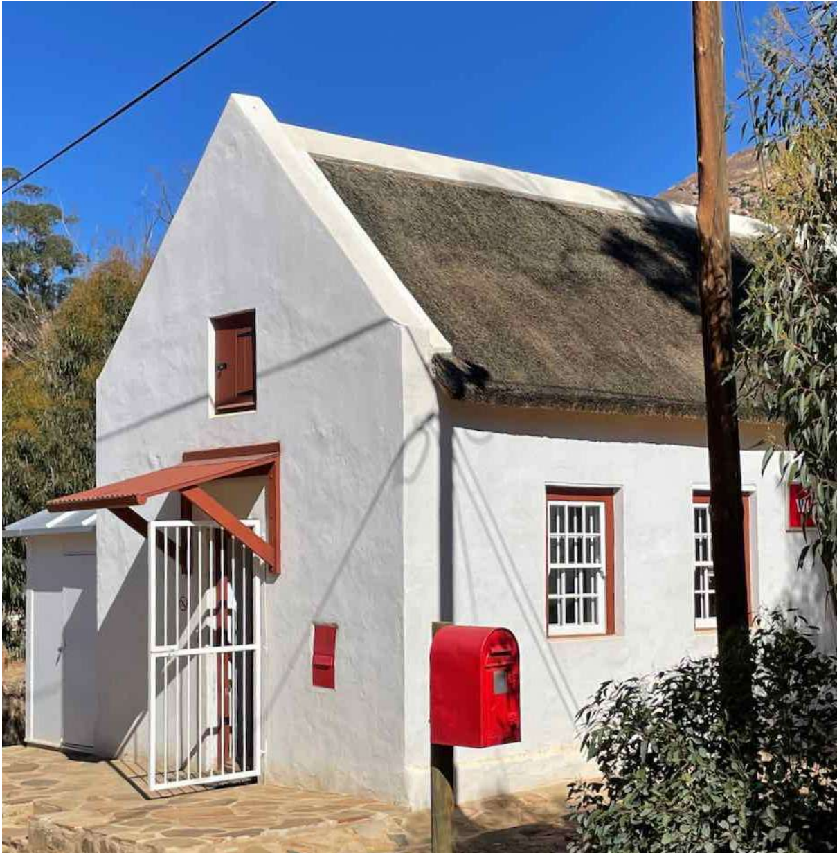
FIGURE 17B: The Post Office Building after refurbishment including new paving on the front stoep using locally sourced sandstone laid by local labour. A smaller corrugated iron front entrance canopy replaced the previous burned out thatch canopy which had been pitched too shallow to withstand the weather for long. (Image: ARCON, 18 May 2021).
