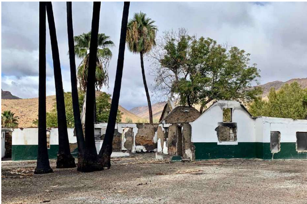
FIGURE 19A: The Old Tannery after the fire. Burning palm fronds played a large role in spreading the fire in the strong wind that had prevailed. (Image: ARCON, 26 May 2020).
