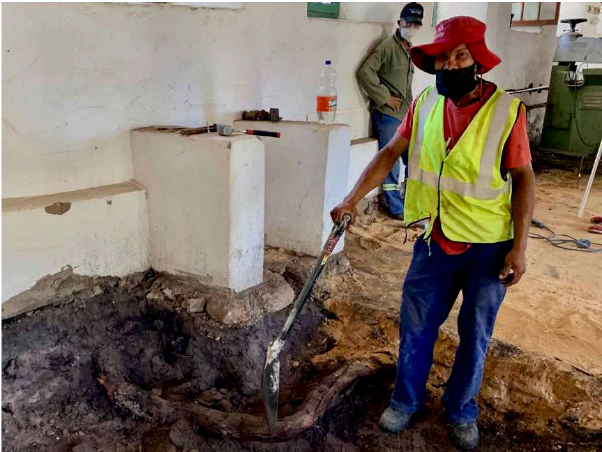
27 November 2020: Removing a massive tree root under the Shoe Factory floor.
