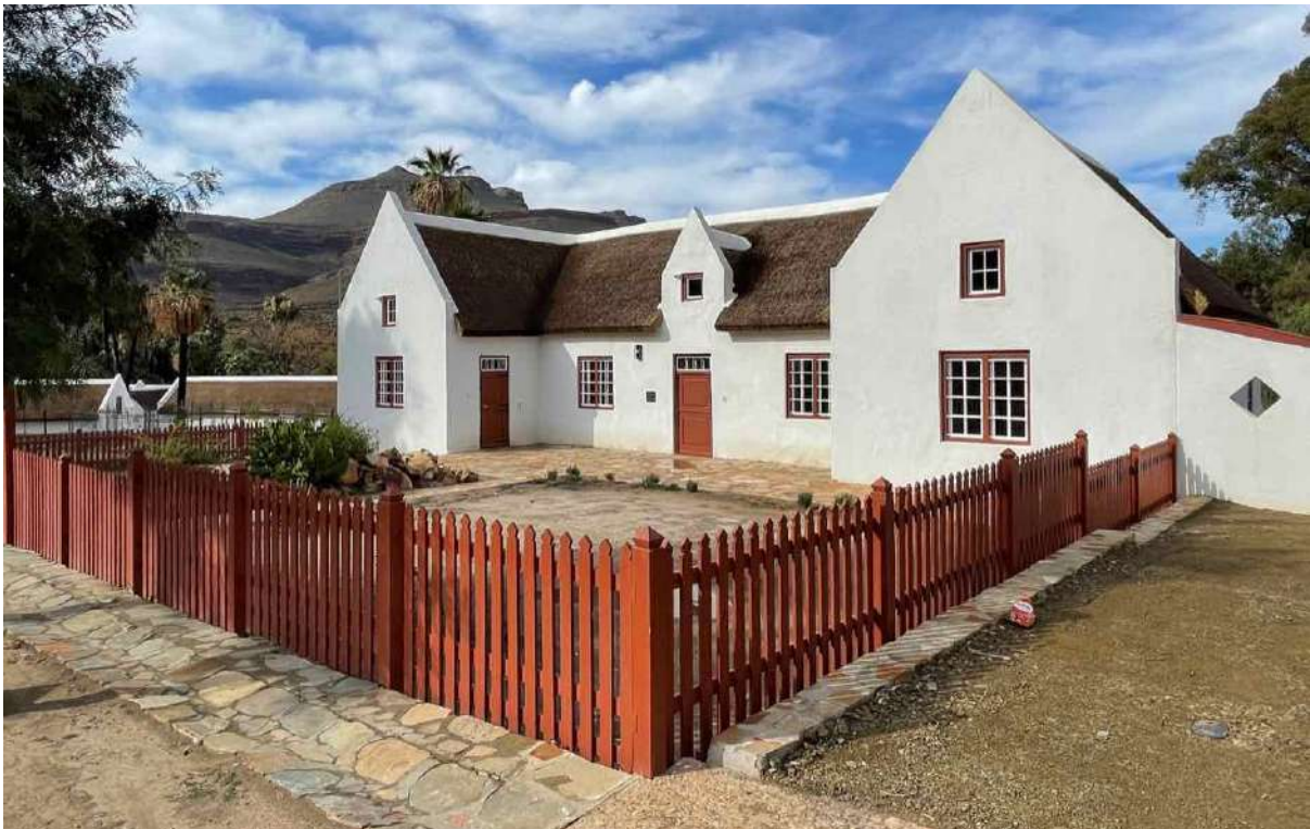
FIGURE 14B: The Parsonage after restoration. The palisade fence was copied from remains that survived the fire in front of the Winkelhuis opposite. (Image: ARCON, 8 June 2021).
