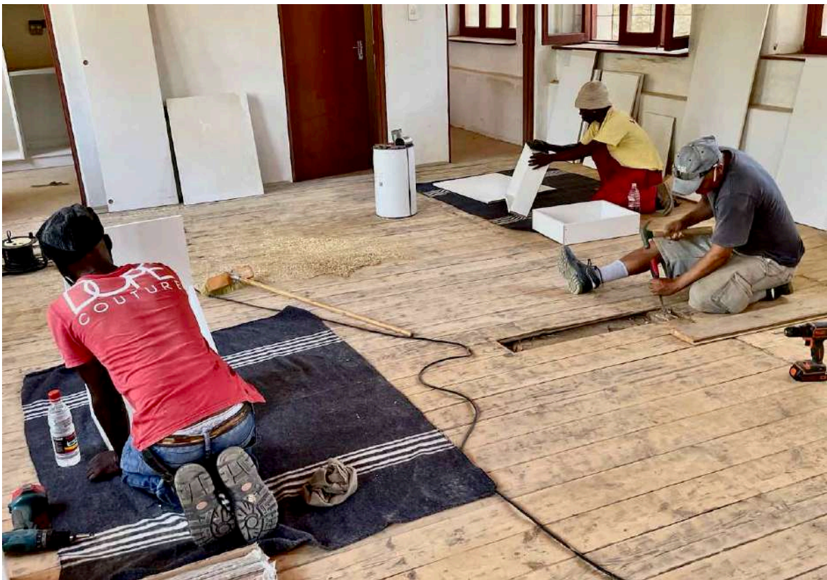
23 March 2021: Repairing the floor in the new Shoe Factory shop space.
