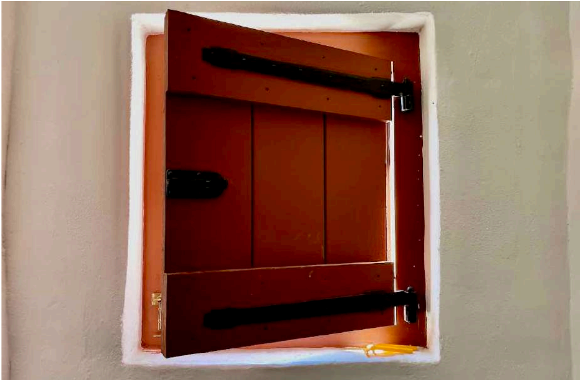
FIGURE 13E: Example of old wrought iron strap hinges recovered after the fire, refurbished and reinstalled in the Mission Stores building. (Image: ARCON, 7 April 2021).
