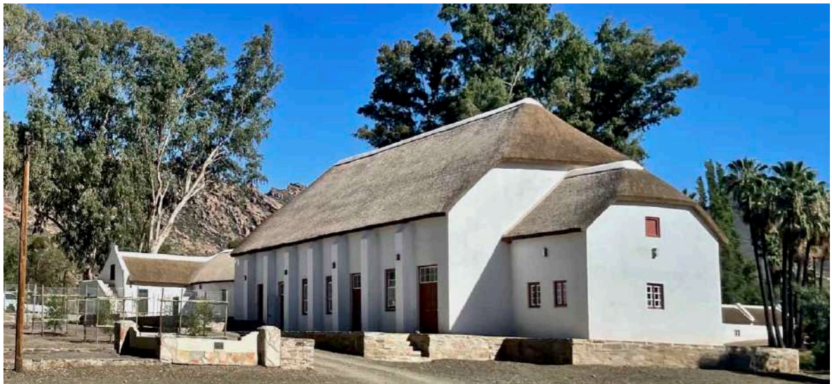
FIGURE 11B: Exterior of the Community Hall after restoration. The small addition in the foreground replaces an earlier cement brick addition that stored the brass band's instruments, and suffered bad structural cracking in the fire. It had to be totally reconstructed because of the damage sustained to its cement brick walls. The walls and buttresses of the main hall were able to be retained. The building is relatively recent, having been constructed in 1980. It was designed by renowned architects Revel Fox & Pnrs. (Image: ARCON, 8 June 2021).
