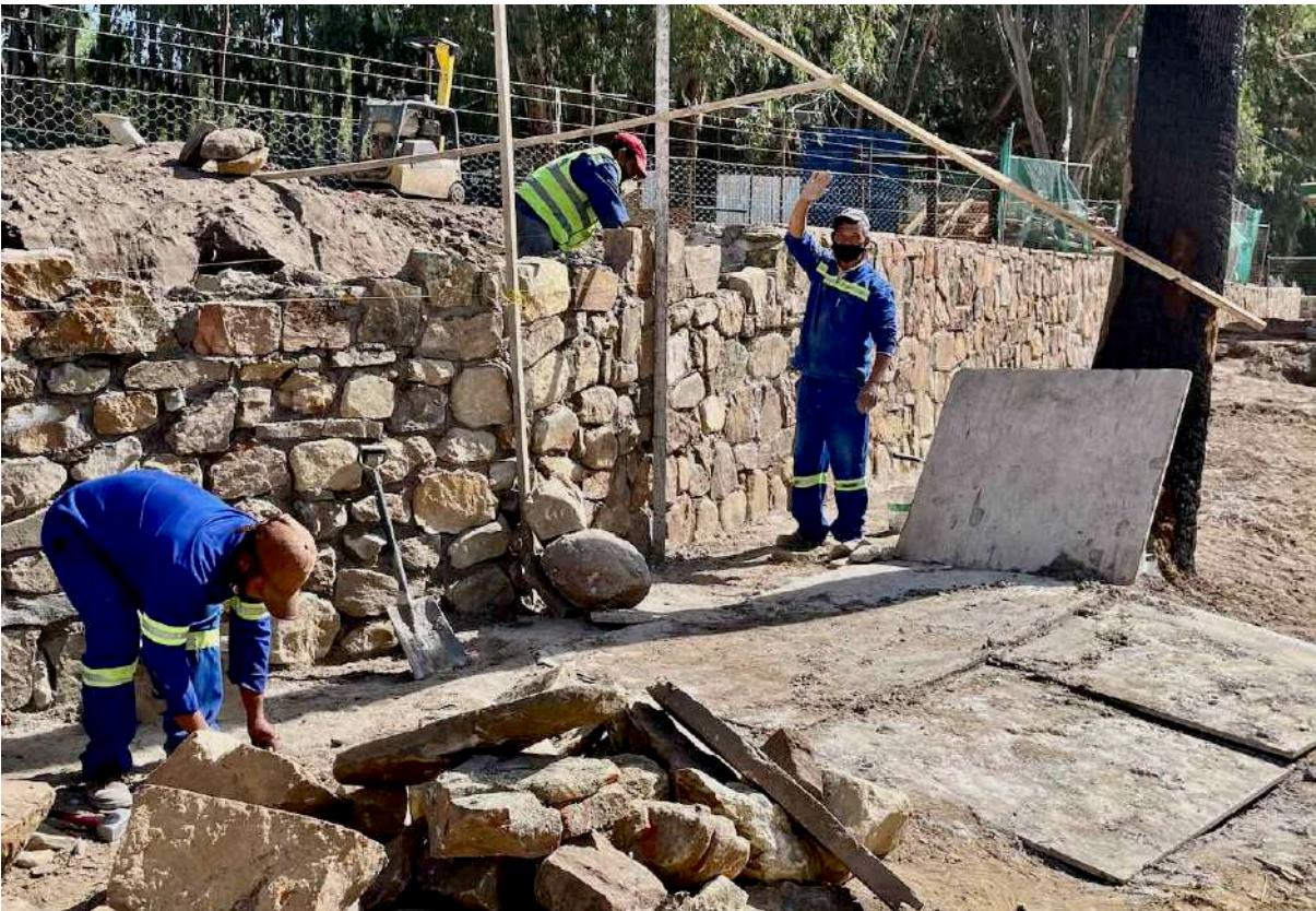
9 March 2021: Reconstructing the retaining walls behind the School Hostels.
