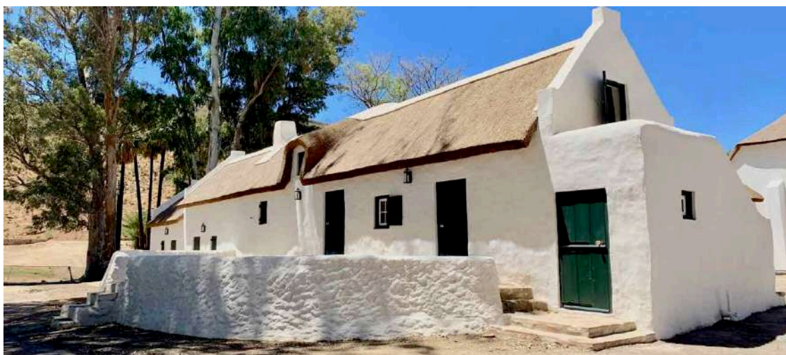
FIGURE 10B: Exterior of Leipoldt House after restoration. (Image: ARCON, 27 Nov 2020).
