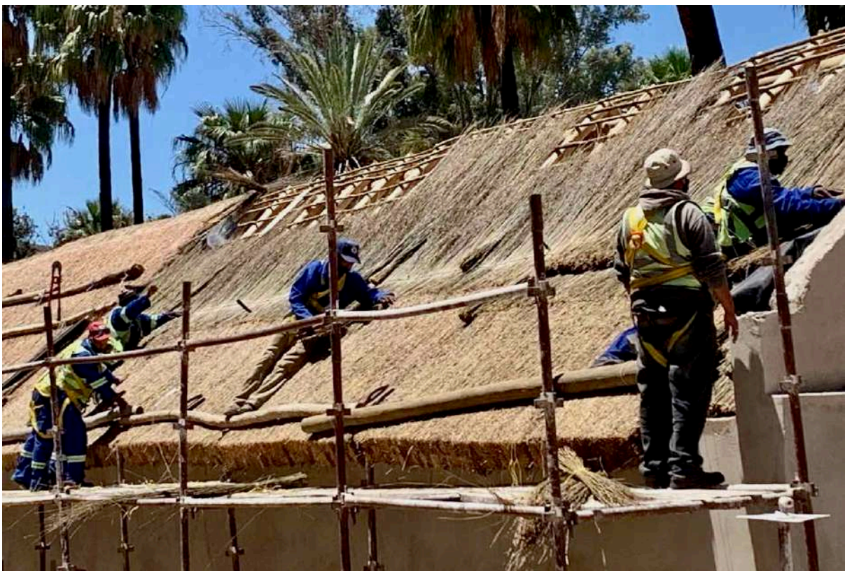
20 November 2020: Thatching one of the School Hostels.
