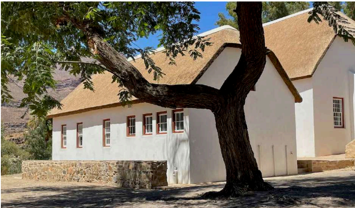
FIGURE 12B: The Creche Building completed. (Image: ARCON, 23 February 2021).
