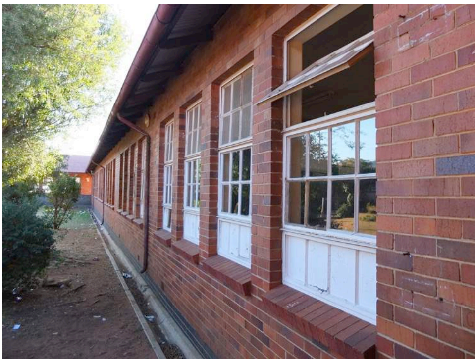
Fig. 35 Detail of brick work and steel frame windows. (Source: tsica heritage consultants, 2016)
