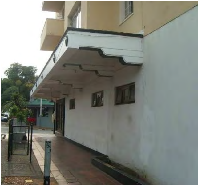
Fig. 6 Melville Mansions, 7 th Street in Melville_example for reinforced concrete cantilever, for Art Deco buildings slabs were supported on brackets with stepped or rounded edge forms.
