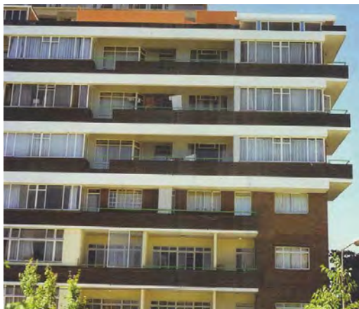
Fig. 13 (Left) University Gate, Braamfontein, 1961 by Clive Chipkin_large deep balconies with box food planting areas. Projections act as summer sun protection. (left)
