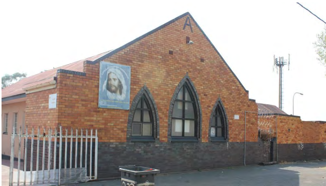
Fig. 270 Side view shows that face brick façade was added later on (Source: tsica heritage consultants, 2015)
