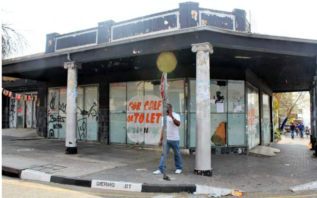
Fig. 245 Image showing altered facades where large windows have replaced original brick walls (Source: tsica heritage consultants, 2015)
