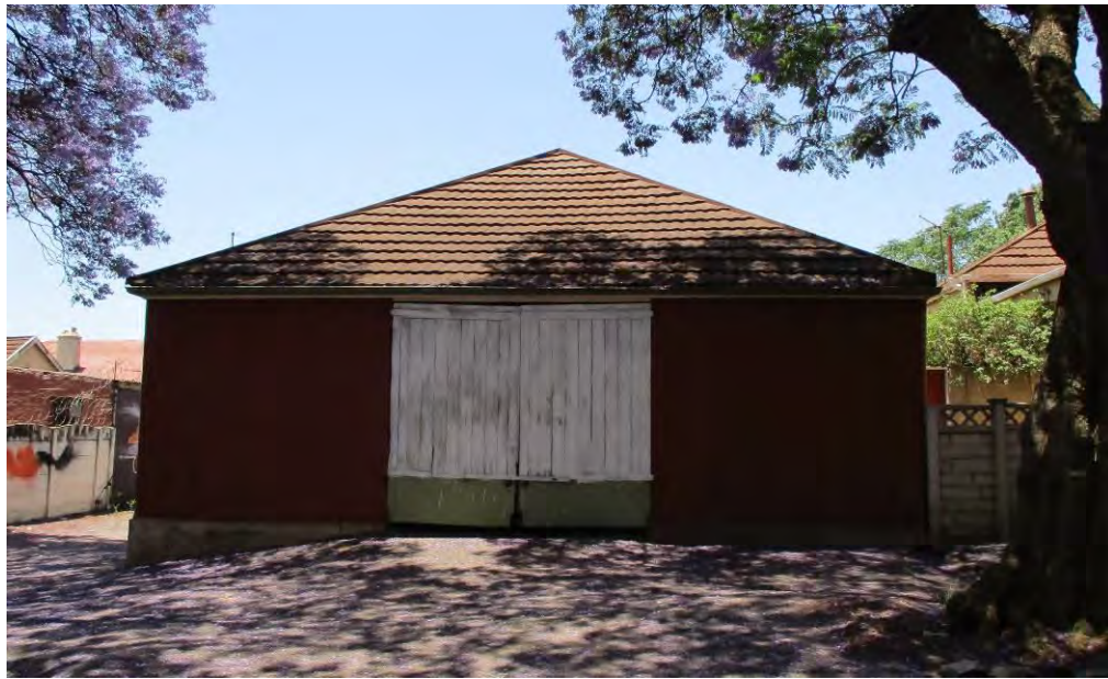
Fig. 196 Coach House main entrance (Source: tsica heritage consultants, 2015)
