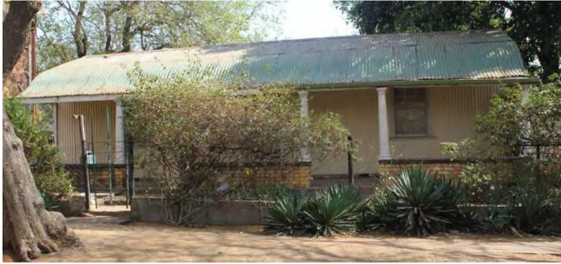
Fig. 140 Original corrugated iron clad house (Source: tsica heritage consultants, 2015)
