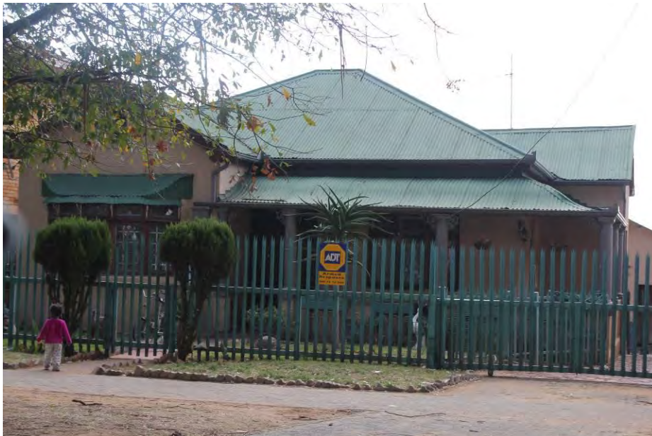
Fig. 157 Original precast columns supporting the verandah are still intact (Source: tsica heritage consultants, 2015)
