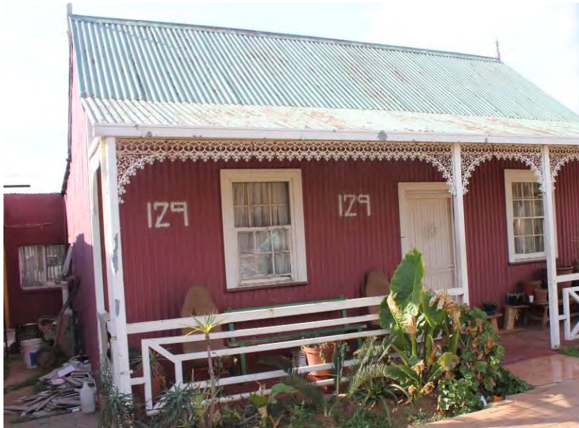
Fig. 138 Original corrugated iron clad house (Source: tsica heritage consultants, 2015)
