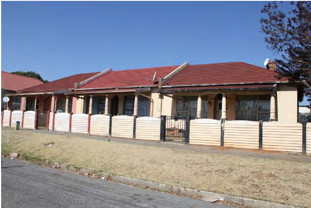
Fig. 149 Row housing front façade facing Biccard Street (Source: tsica heritage consultants, 2015)
