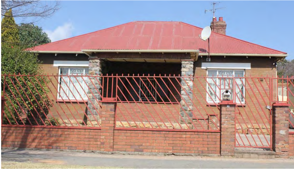
Fig. 184 Single storey corrugated iron house with raised centrally located stoep (Source: tsica heritage consultants, 2015)
