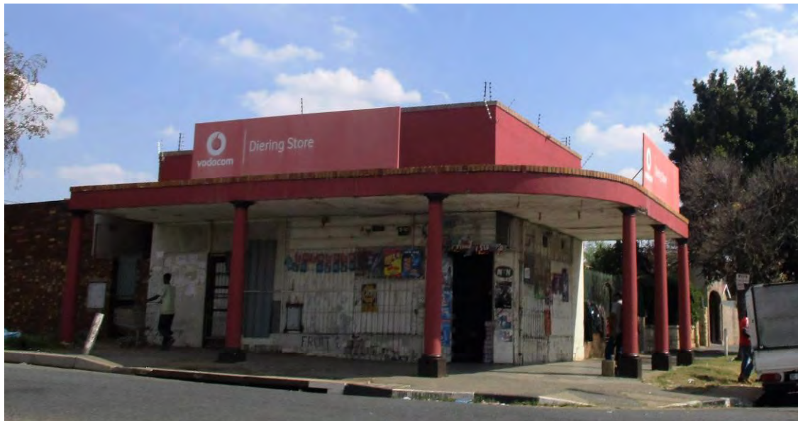
Fig. 256 Corner shop along Diering Street (Source: tsica heritage consultants, 2015)
