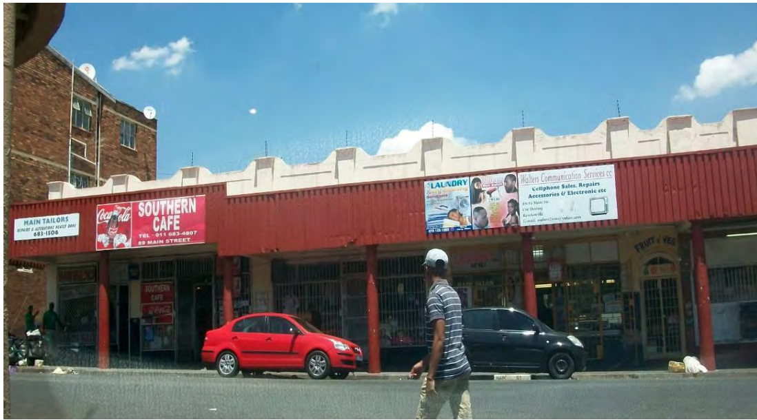
Fig. 247 Row of shops along Main street (Source: tsica heritage consultants 2015)
