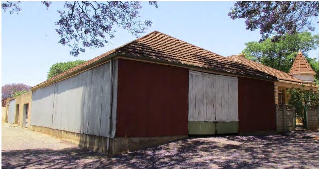
Fig. 153 Original coach house in corrugated iron cladding (Source: tsica heritage consultants, 2015)
