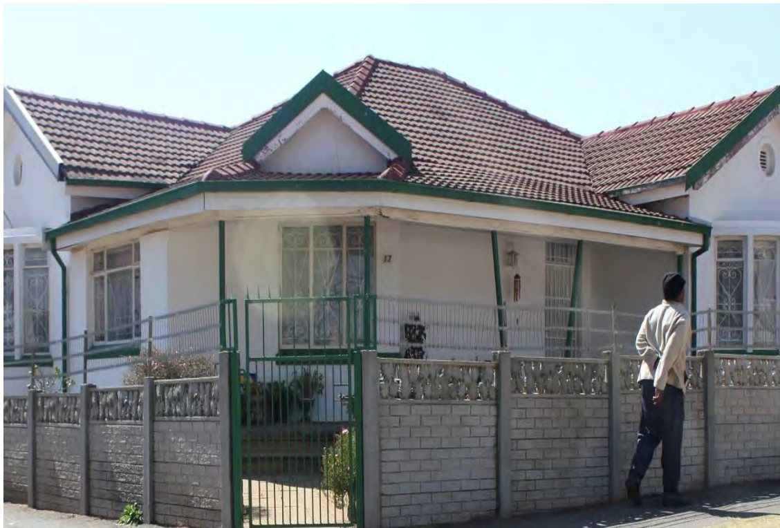
Fig. 169 Corner house (Source: tsica heritage consultants, 2015)
