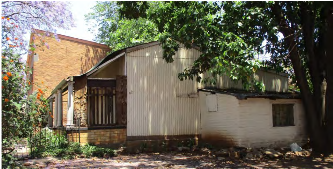
Fig. 141 Side elevation corrugated iron clad house (Source: tsica heritage consultants, 2015)
