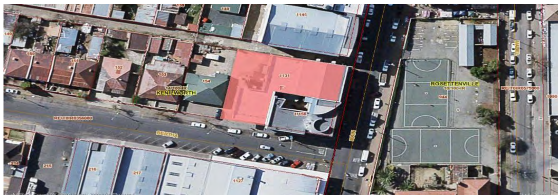
Fig. 234 Located at an advantageous position along Main Street at the border of Rosettenville and Kenilworth (Source: City Council of Johannesburg, GIS map)
