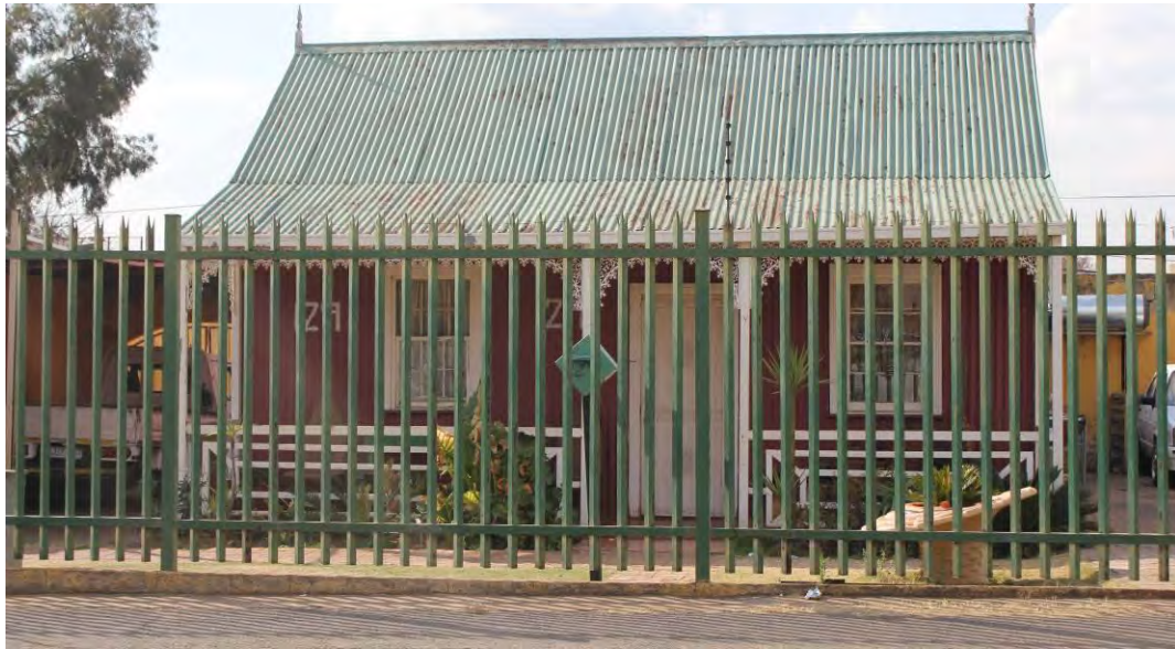
Fig. 137 Original corrugated iron clad house (Source: tsica heritage consultants, 2015)
