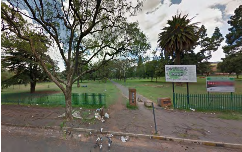
Fig. 211 Rotunda Park before the upgrade (Source: tsica heritage consultants)
