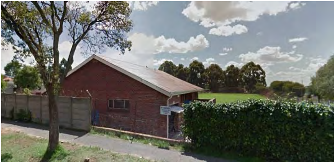
Fig. 216 View of the buildings from President Street (Source: tsica heritage consultants, 2015)
