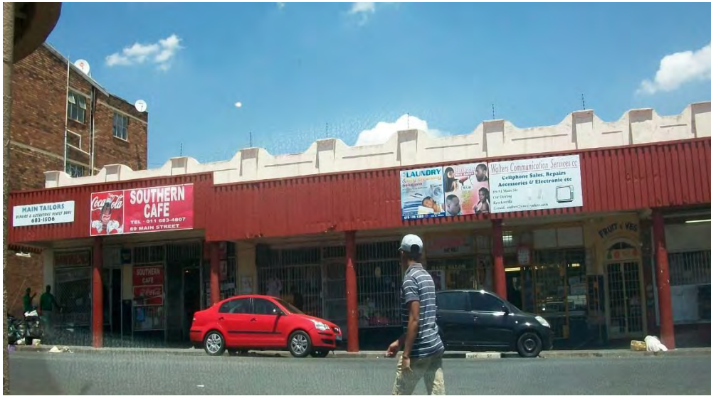
Fig. 228 Row of single storey shops (Source: tsica heritage consultants, 2015)
