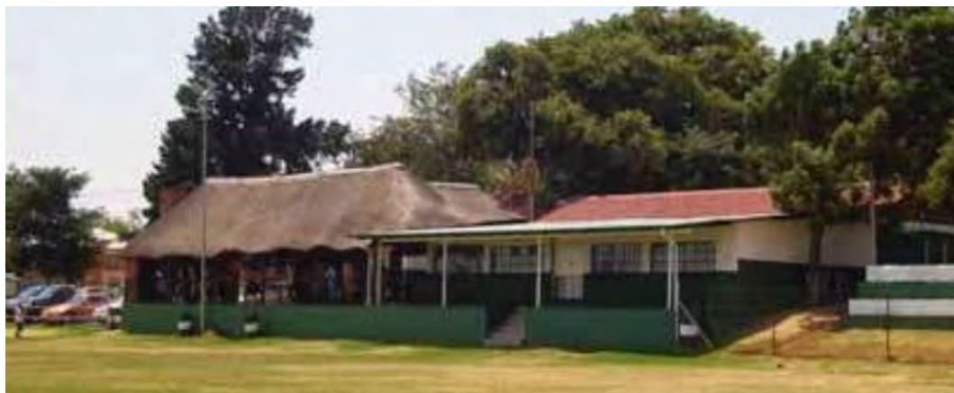
Fig. 217 View of the buildings from President Street (Source: tsica heritage consultants, 2015)
