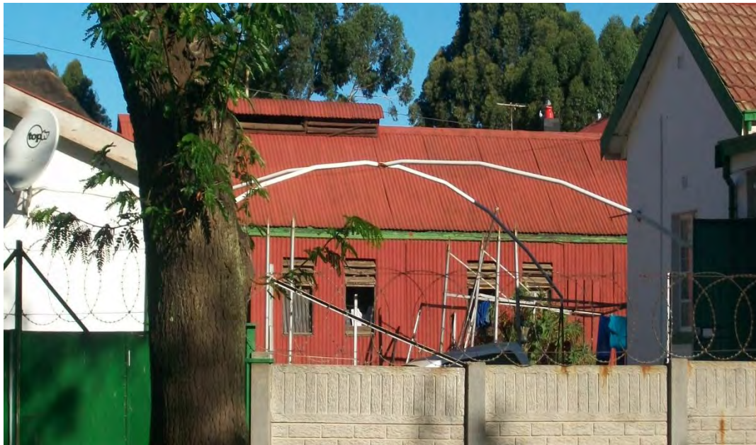
Fig. 171 Zoom in to the original stables with corrugated iron cladding (Source: tsica heritage consultants, 2015)
