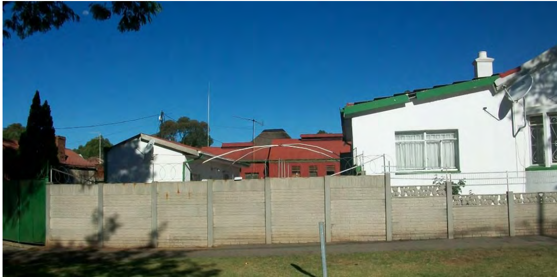
Fig. 170 Original corrugated iron stables in the backyard (Source: tsica heritage consultants, 2015)
