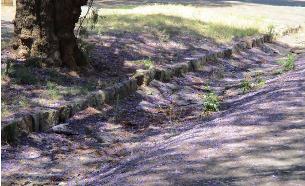
Fig. 202 Stone water channels along Von Brands Street (Source: tsica heritage consultants, 2015)
