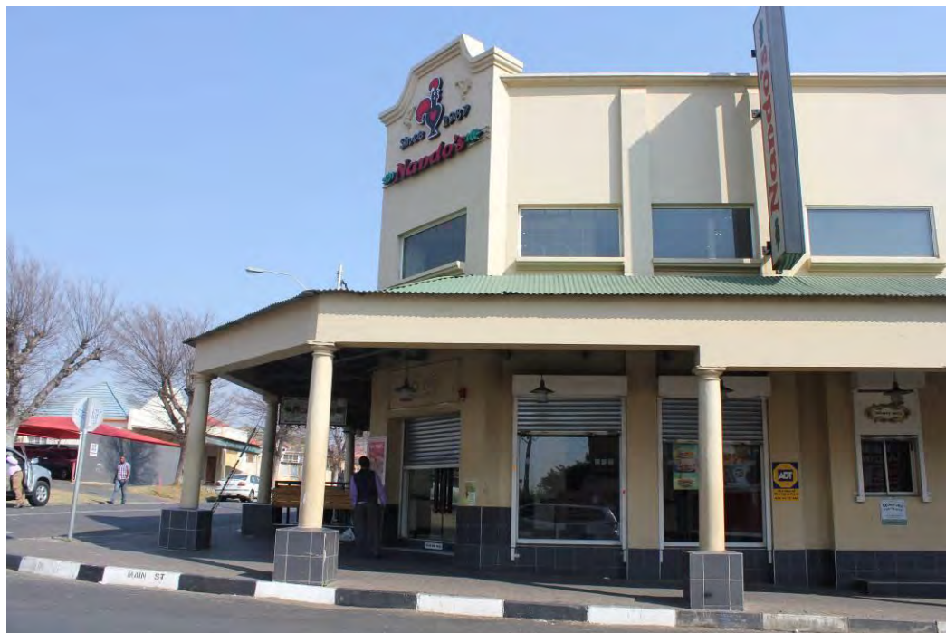
Fig. 250 First Nandos building in Kenilworth along Main street (Source: tsica heritage consultants 2015)
