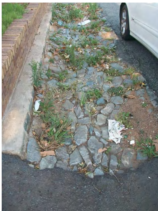
Fig. 201 Stone water channels along Donnelly Street (Source: tsica heritage consultants, 2015)
