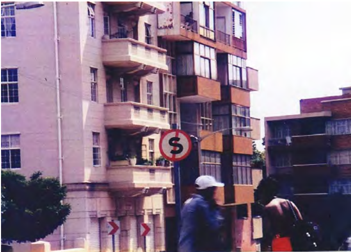
Fig. 28 Ridge View Corner Banket Street (left); Reading Court (right), Ridge View is a setback flat block from the 1920's which creates a memorable urban space (Photograph: Clive Chipkin)
