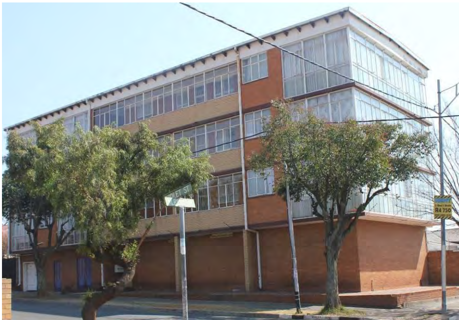
Fig. 123 Front façade is south facing at the corner of Violet Street and Albert Street (Source: tsica heritage consultants, 2015)
