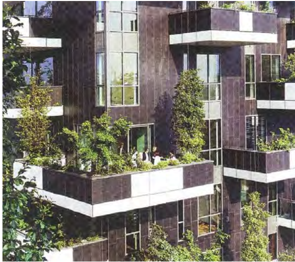
Fig. 12 Balconies as plant areas. Bosco Verticale, Milan. Architect: Boeri Studio. (Source: Earthworks journal, Issue 24/2015)
