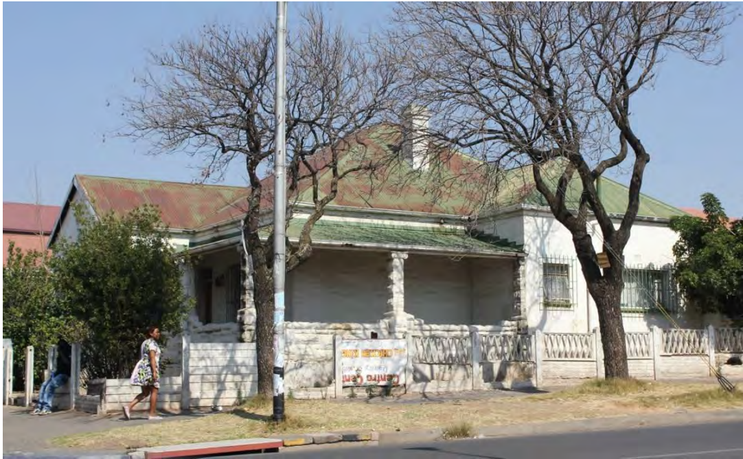
Fig. 129 Original street frontage along Geranium Street (Source: tsica heritage consultants, 2015)
