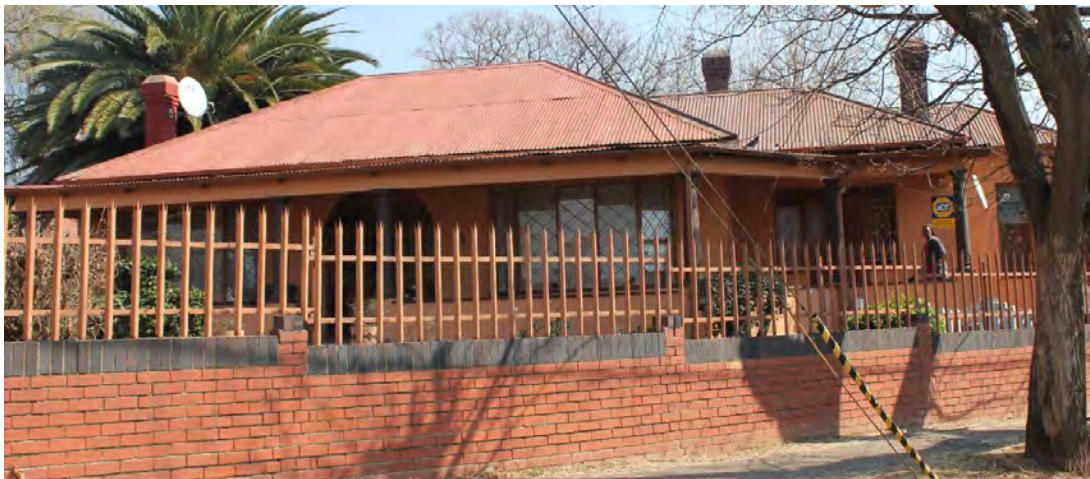
Fig. 136 Original street frontage corner Haig and Mabel Street (Source: tsica heritage consultants, 2015)
