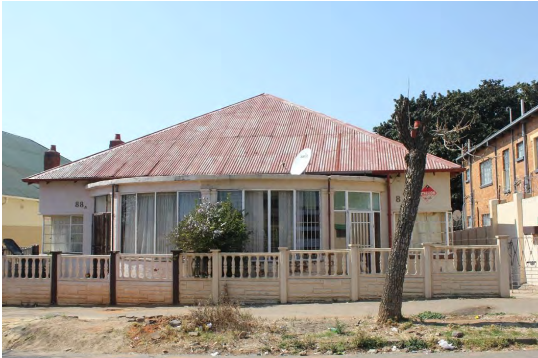
Fig. 157 Original street façade facing Bouquet Street (Source: tsica heritage consultants, 2015)
