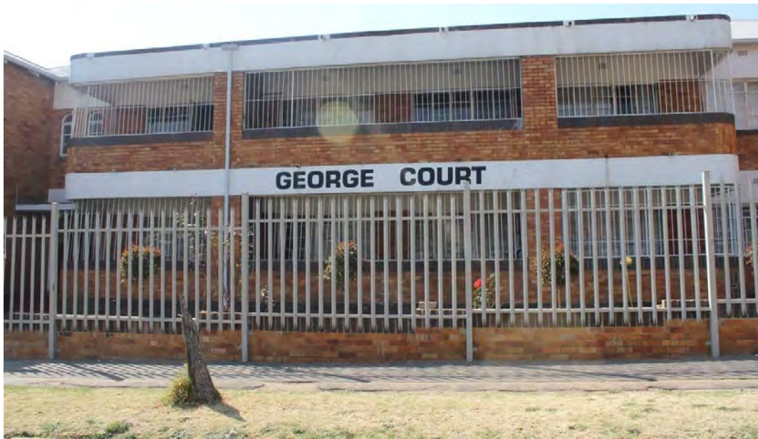
Fig. 114 Original street frontage along George Street (Source: tsica heritage consultants, 2015)
