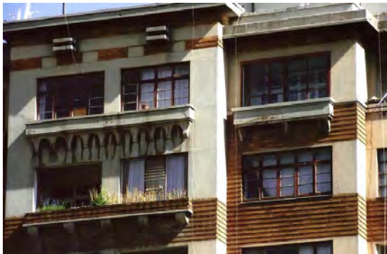
Fig. 19 & Fig. 20 Clarendon Circle – a hub of 1920s and 1930s blocks of flats. Majestic Mansions and Parktown Mansions are gone but Circle Court (1936), the essence of Clarendon Circle, remains. The Art Deco sub-theme reaches its full expression in an entrance foyer that is an Art Deco exemplar.
