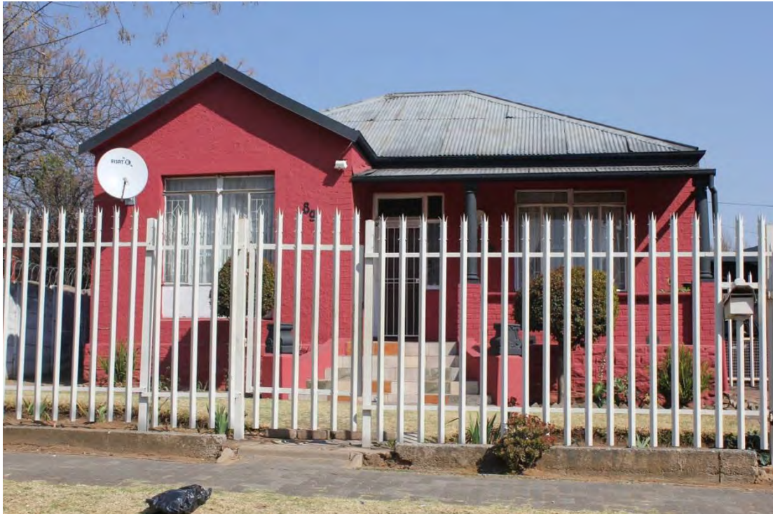
Fig. 138 Street façade along Mabel Street (Source: tsica heritage consultants, 2015)
