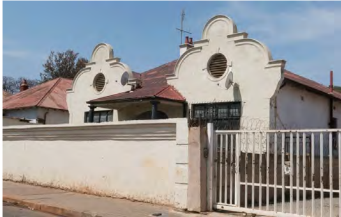
Fig. 3 Semi-Dutch gabled houses along Hillbrow Street from 1910-1920s (Source: tsica heritage consultants, 2015)
