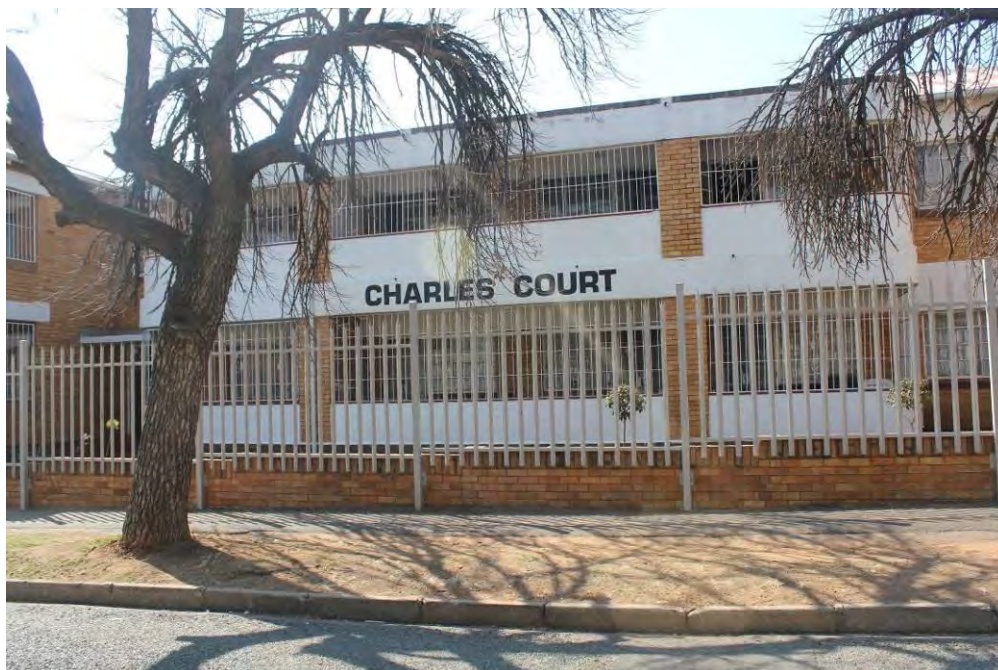
Fig. 115 Another flat an exact copy of George Court situated on the same street (Source: tsica heritage consultants, 2015)
