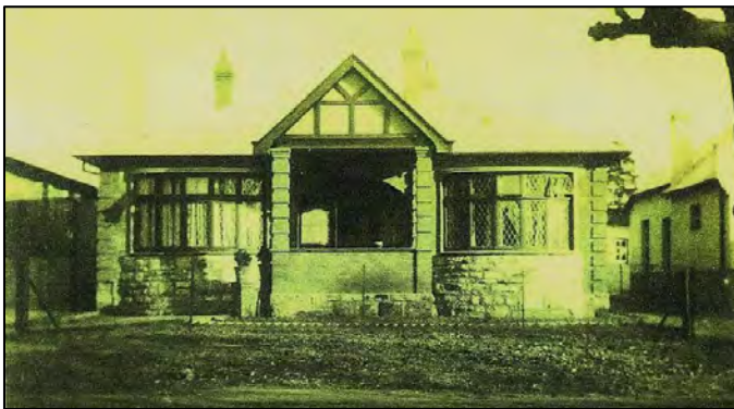
Fig. 4 House along St. Georges Street in Yeoville with projecting stoep, triangular half-timbered gable in mock Tudor and English bay windows (Source: Clive Chipkin Archive)
