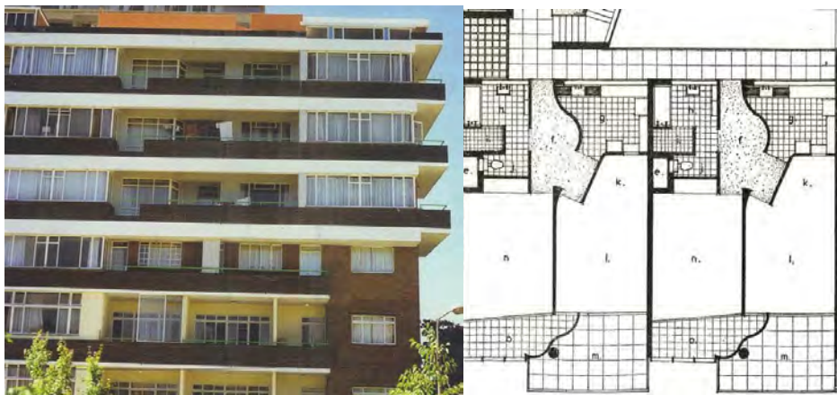
Fig. 13 (Left) University Gate, Braamfontein, 1961 by Clive Chipkin_large deep balconies with box food planting areas. Projections act as summer sun protection. (left)
