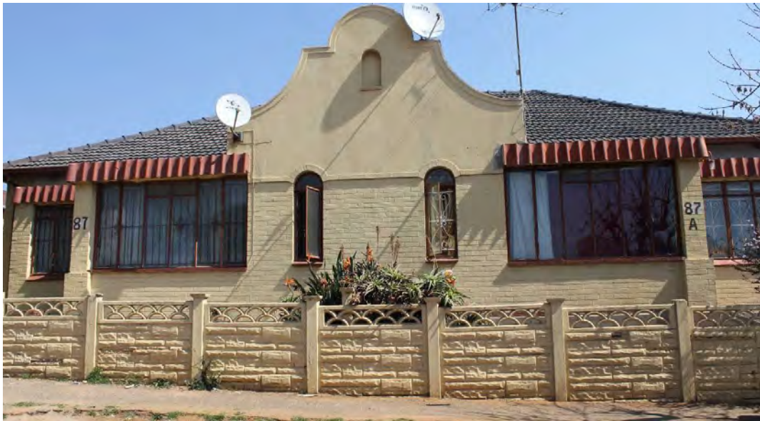
Fig. 154 Original street façade facing Bouquet Street (Source: tsica heritage consultants, 2015)
