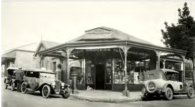
Fig. 5 Corner shop built in 1905 along 7th Street and 3rd Avenue in Melville, cast iron columns supporting the roof structure
