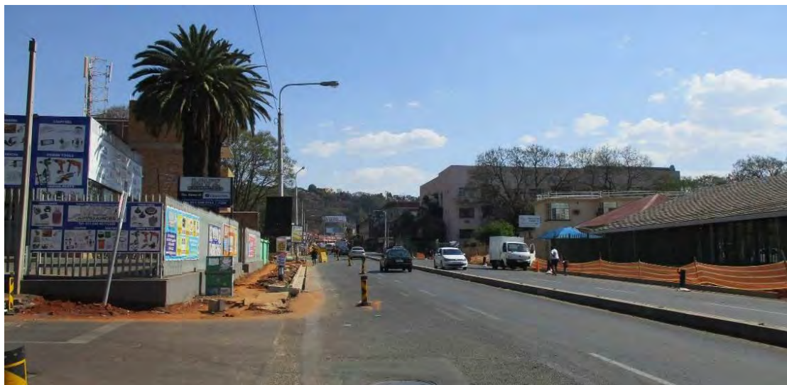
Fig. 19 View in southern direction with the local library building located in western direction along Louis Botha Avenue (Source: tsica heritage consultants, 2015)
