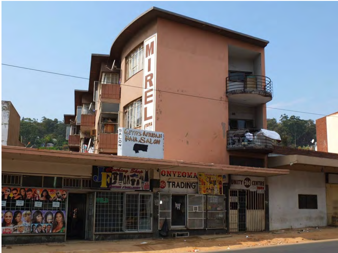
Fig. 37 Three storey commercial mixed-use building with shops on street level and apartments above along the south-western side of Louis Botha Avenue (Source: tsica heritage consultants, 2015)
