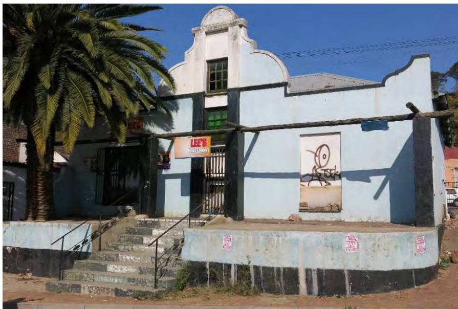
Fig. 25 Single storey building with centrally located Cape Dutch Gable along the southern side of Louis Botha Avenue (Source: tsica heritage consultants, 2015)
