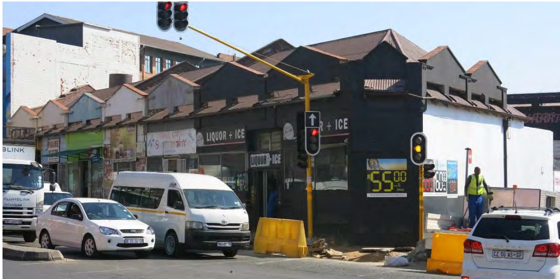
Fig. 49 Single storey row of shops on street level located on the north-western corner of Seventh and Louis Botha Avenue (Source: tsica heritage consultants, 2015)
