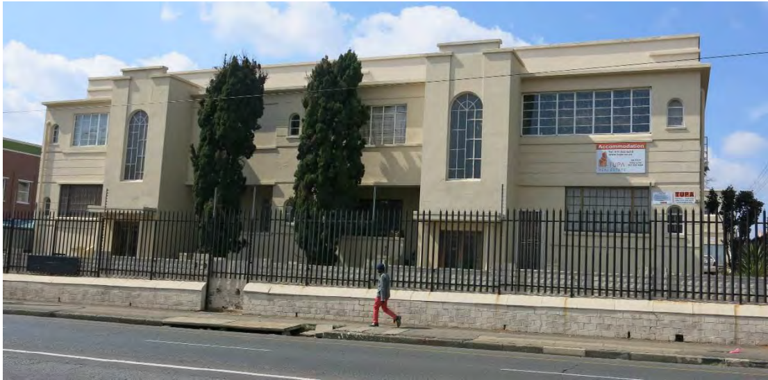
Fig. 79 East elevation along Louis Botha features two main entrances with staircase section breaking the horizontally structured façade vertically (Source: tsica heritage consultants, 2015)
