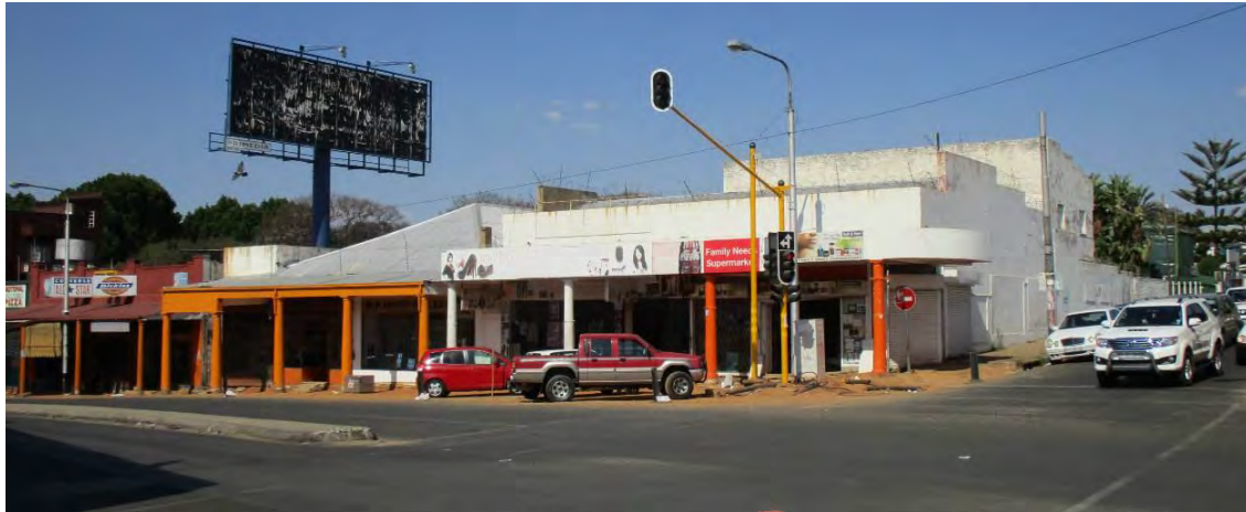
Fig. 53 Single storey row of shops on street level located on the north-eastern corner of Eighth and Louis Botha Avenue (Source: tsica heritage consultants, 2015)
