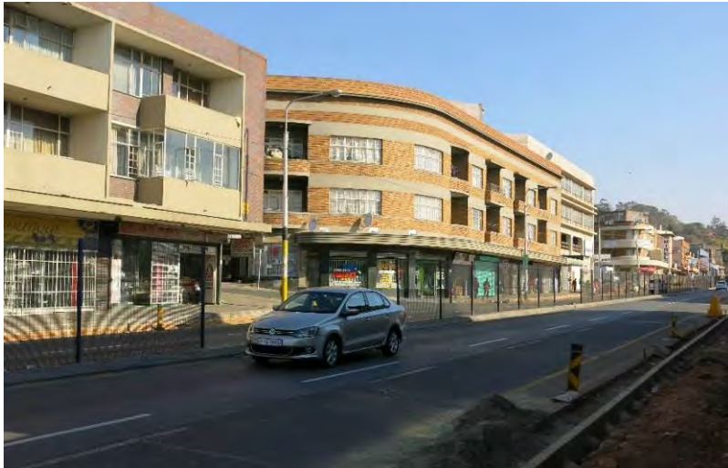
Fig. 15 View in south-western direction with mixed-use buildings all along that section of Louis Botha Avenue (Source: tsica heritage consultants, 2015)
