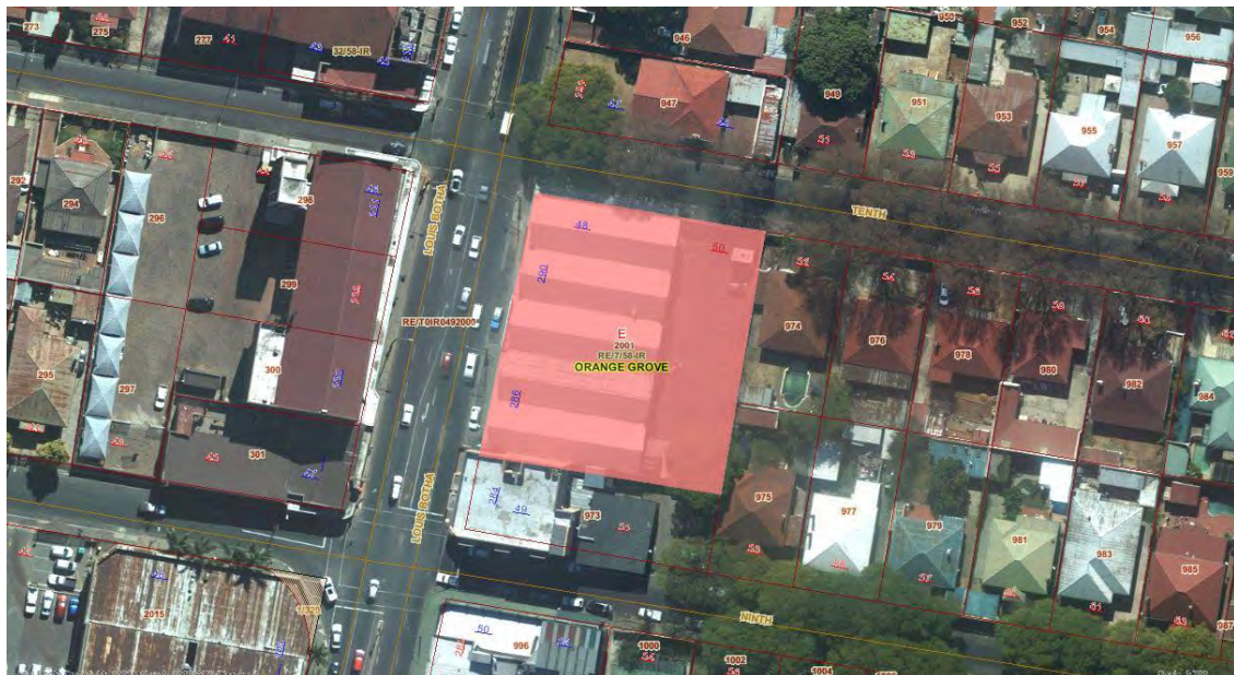
Fig. 62 Stand 2001 is located on the south-eastern corner of Louis Botha Avenue and Tenth Street
