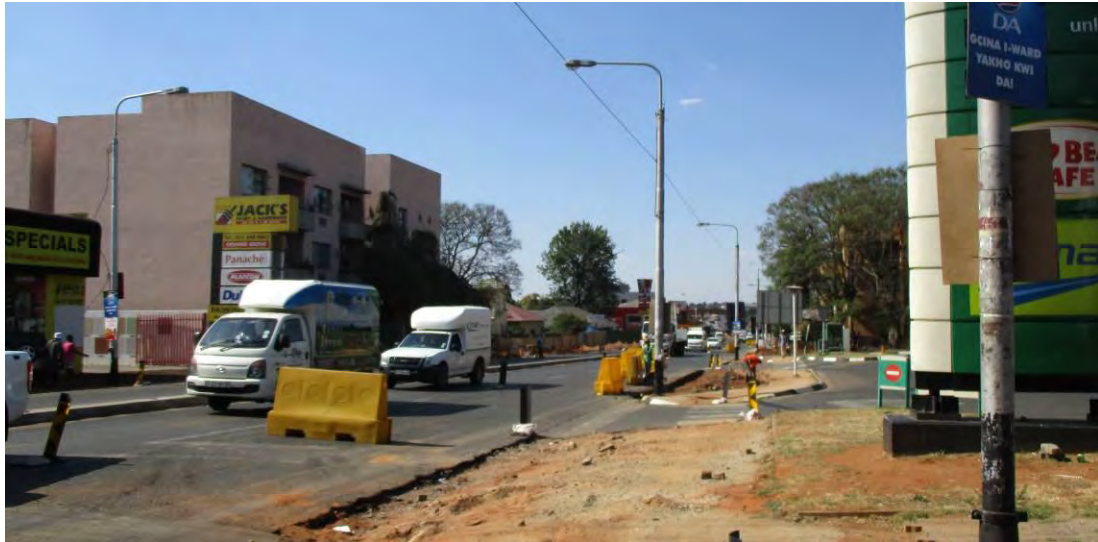
Fig. 18 View in northern direction with a number of commercial and mixed-use buildings all along that section of Louis Botha Avenue (Source: tsica heritage consultants, 2015)
