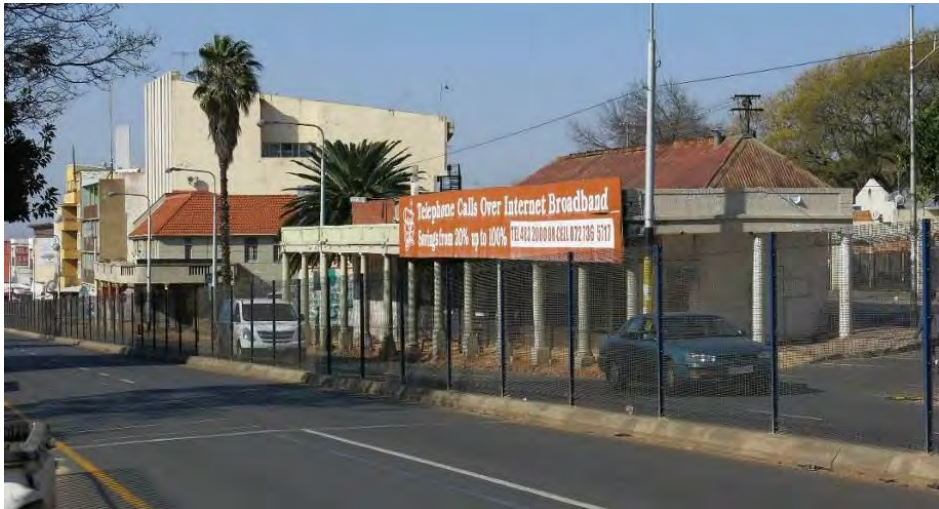
Fig. 12 View in north-eastern direction along Louis Botha Avenue, south-western boundary line of Orange Grove (Source: tsica heritage consultants, 2015)
