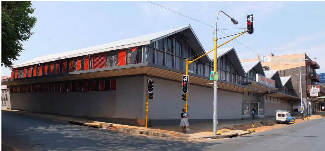
Fig. 63 OK Bazaar from 1956 on the Corner of Louis Botha Avenue and Tenth Street (Source: tsica heritage consultants, 2015)
