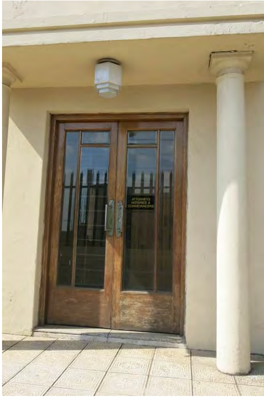
Fig. 81 Original main entrance along Louis Botha Avenue (Source: tsica heritage consultants, 2015)
