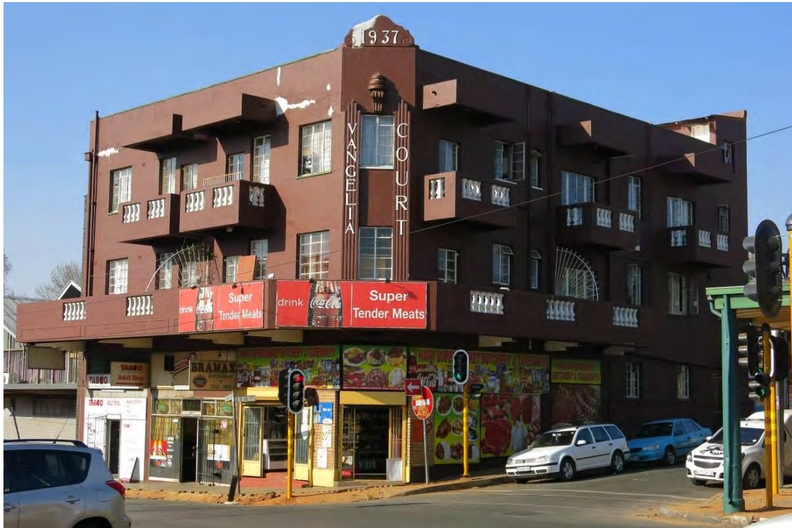
Fig. 61 Vangelia Court from 1937 on the Corner of Louis Botha Avenue and Ninth Street (Source: tsica heritage consultants, 2015)
