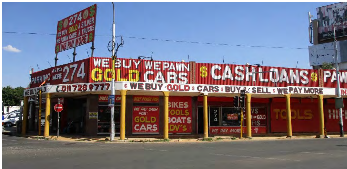
Fig. 45 Originally single storey row of shops with covered veranda along shop front (Source: tsica heritage consultants, 2015)
