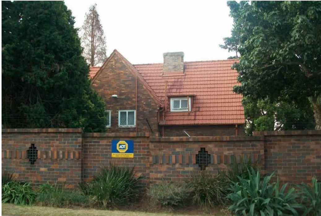
Fig. 113 Single storey red face brick residence with steep pitched tiled roof and triangular centrally located front gable, roof is used as additional living space (Source: tsica heritage consultants, 2015)
