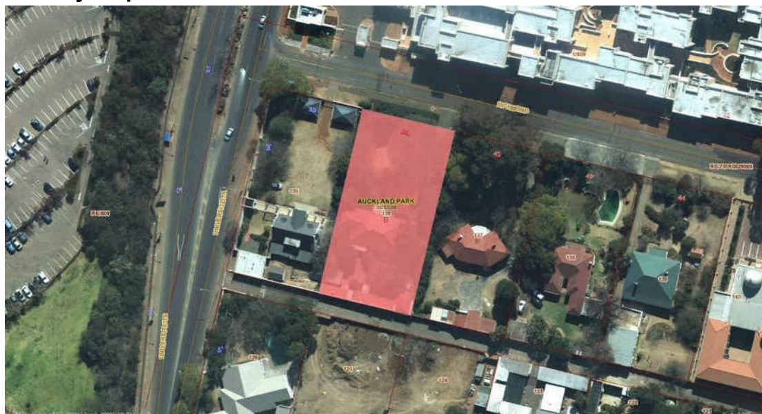
Fig. 81 Stand 136 is located along the northern side of Richmond Avenue which runs parallel to Kingsway Avenue in Auckland Park and is rarely visible from the street (Source: City Council of Johannesburg, GIS map)
