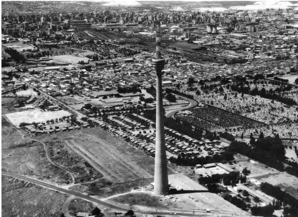
Fig. 164 Sentech tower under construction with Jan Hofmeyr in the background (Source: City Council of Johannesburg, GIS Map)
