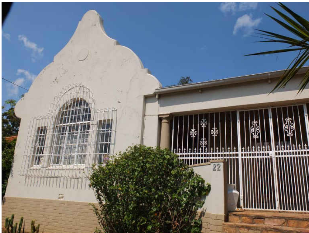
Fig. 149 North elevation with semi-Dutch gable and corner stoep (Source: tsica heritage consultants, 2015)
