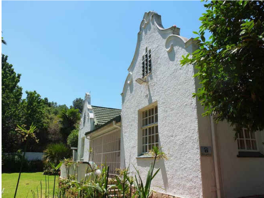
Fig. 160 Double semi-dutch gables on both sides with centrally located front stoep (Source: tsica heritage consultants, 2015)
