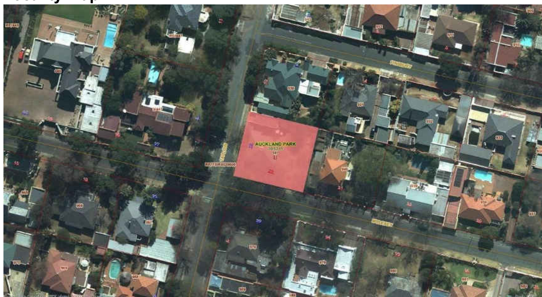
Fig. 139 Stand 941 is located along the northern side of Finsbury Avenue in close proximity to Cookham Road
