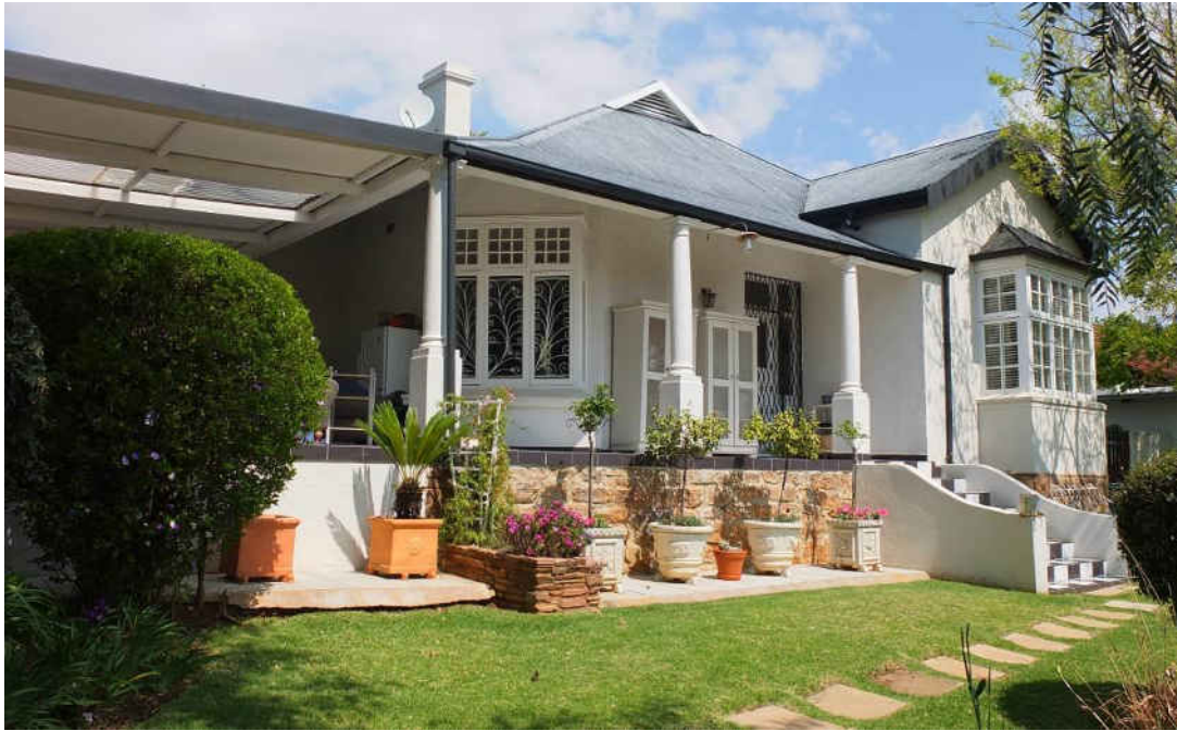
Fig. 121 Single storey residence with natural stone plinth and columns supported corner stoep (Source: tsica heritage consultants, 2015)
