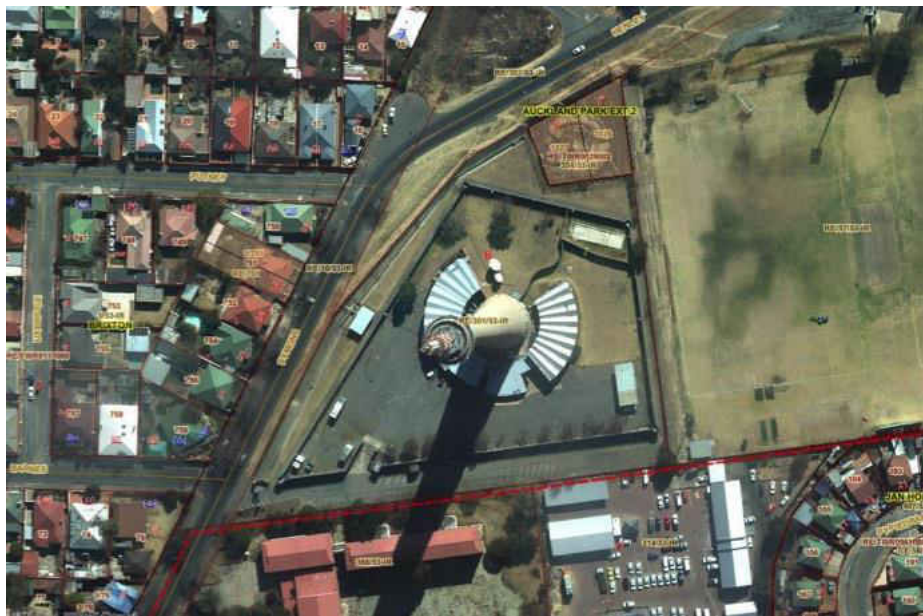
Fig. 163 Sentech tower along the eastern side of Symons Road (Source: City Council of Johannesburg, GIS Map)
