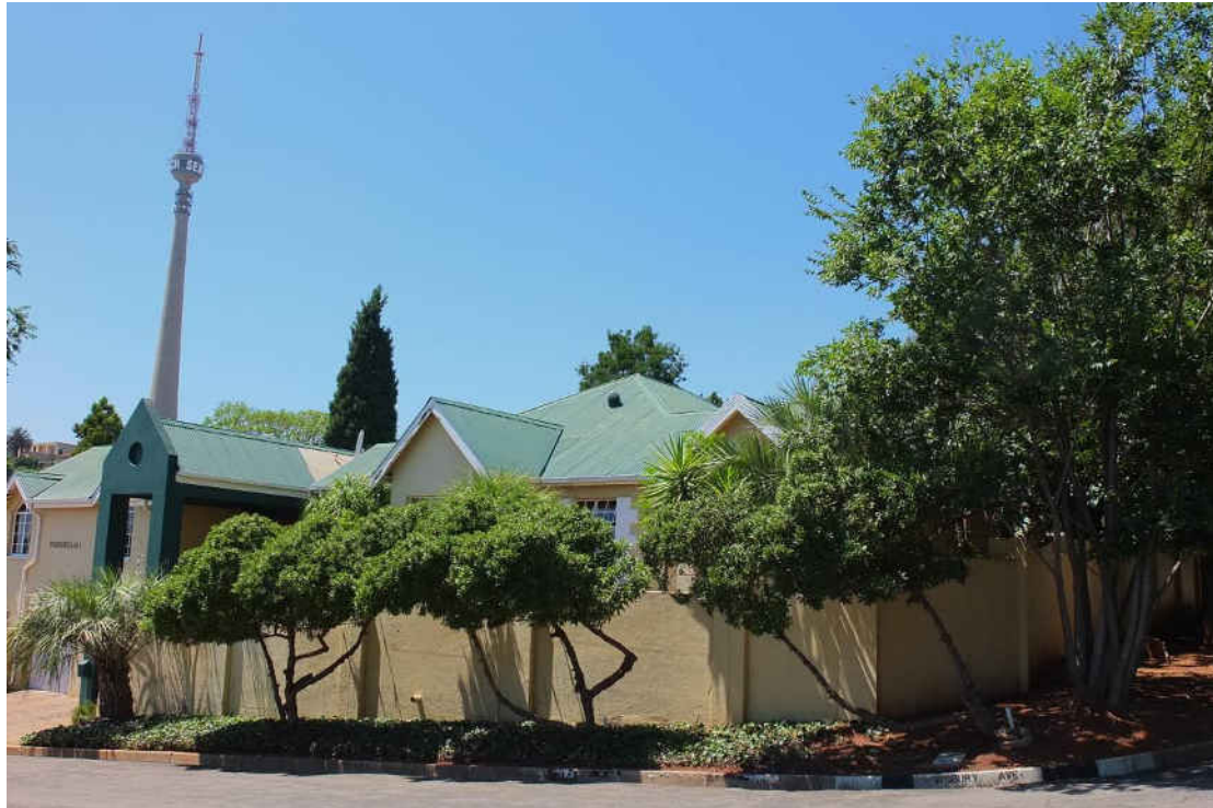
Fig. 119 Single storey residence with corrugated iron roofing was added on to along the eastern side but still forms part of historical corner streetscape in Auckland Park (Source: tsica heritage consultants, 2015)
