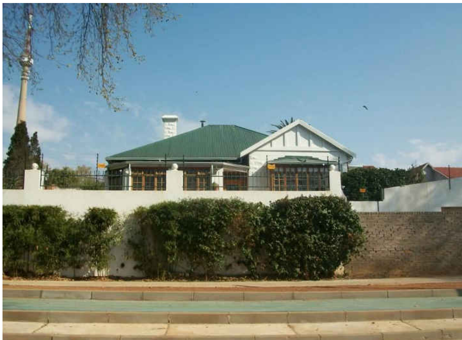
Fig. 108 View towards the northern façade of the single storey freestanding residence with corrugated iron roof and triangular gable with bay window (Source: tsica heritage consultants, 2015)
