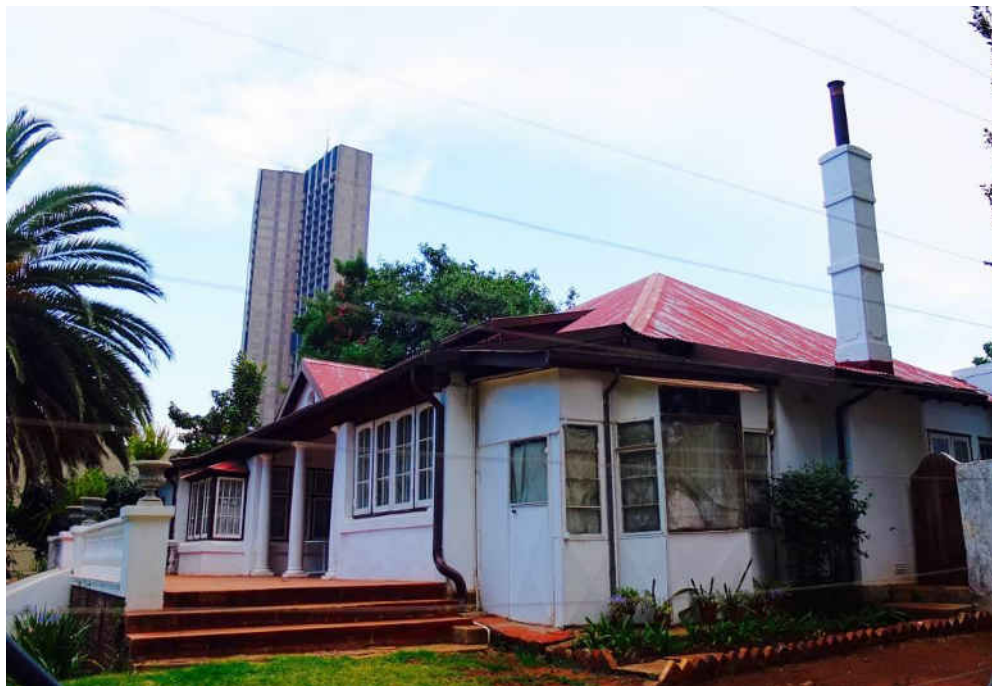
Fig. 80 View towards the North-western elevations with the SABC office block in the background along Henley Road (Source: tsica heritage consultants, 2015)
