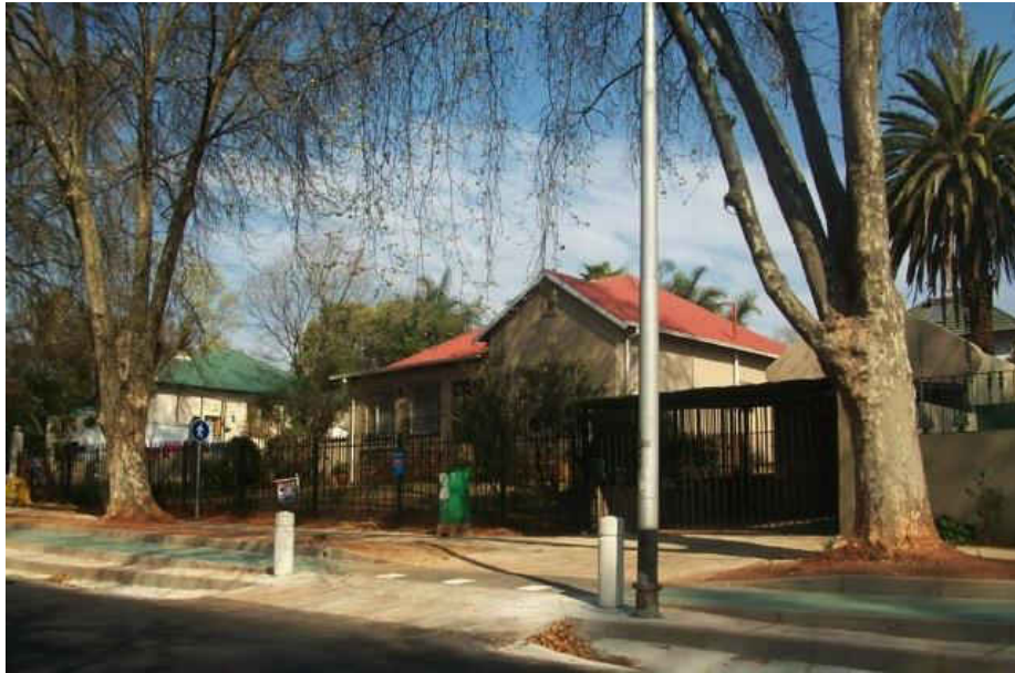
Fig. 111 View towards the northern façade of the single storey freestanding residence with corrugated iron roof and triangular gable (Source: tsica heritage consultants, 2015)
