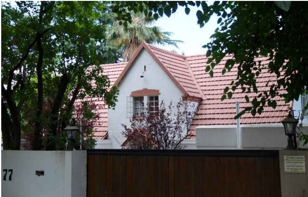
Fig. 74 View in northern direction of main entrance gate of Stand 161, original slate-tiled roof was replaced with clay tiles (Source: tsica heritage consultants, 2015)
