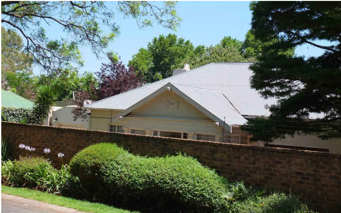
Fig. 115 Single storey residence with centrally located front stoep which was more recently enclosed (Source: tsica heritage consultants, 2015)
