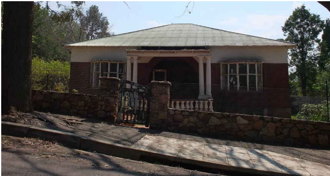
Fig. 140 Typical single storey freestanding residence with corrugated iron roofing and red face brick façade, two pairs of double columns supporting the centrally located front stoep roof
