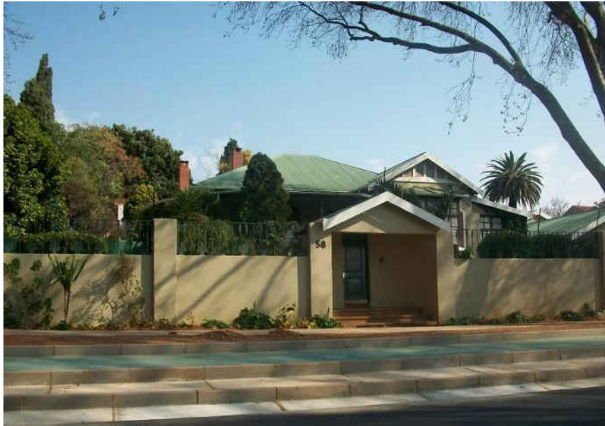
Fig. 109 View towards the northern façade of the single storey freestanding residence with corrugated iron roof and triangular gable with bay window (Source: tsica heritage consultants, 2015)
