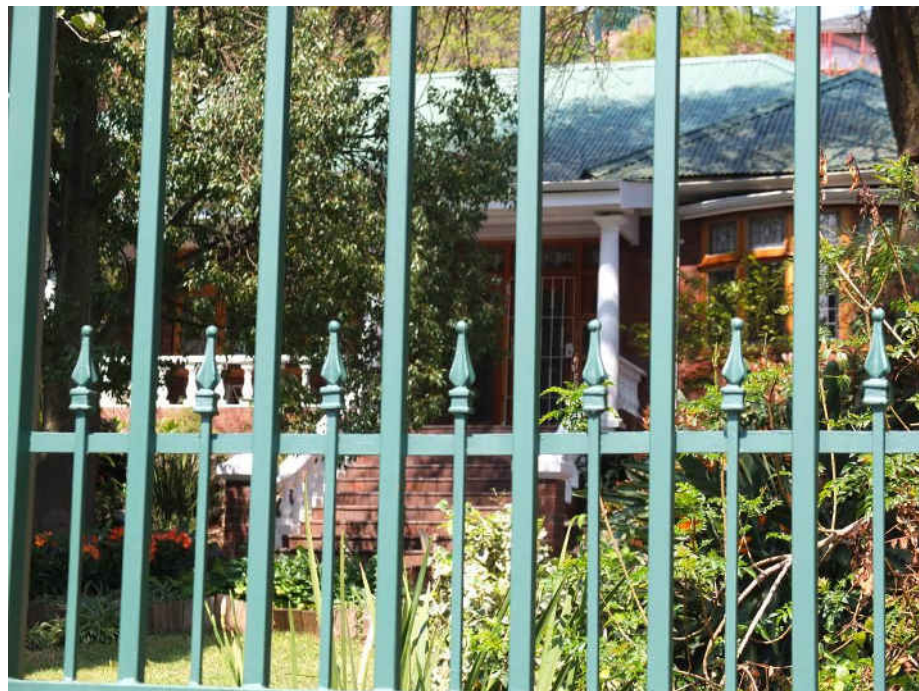
Fig. 146 A number of original design features are visible and still in a very good condition, like wooden windows and doors (Source: tsica heritage consultants, 2015)
