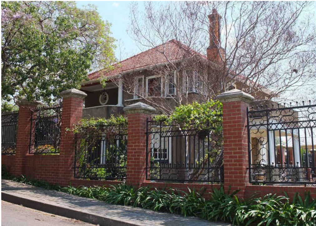
Fig. 142 Double storey residence with tiled roofing and prominent design features of the 1920s (Source: tsica heritage consultants, 2015)
