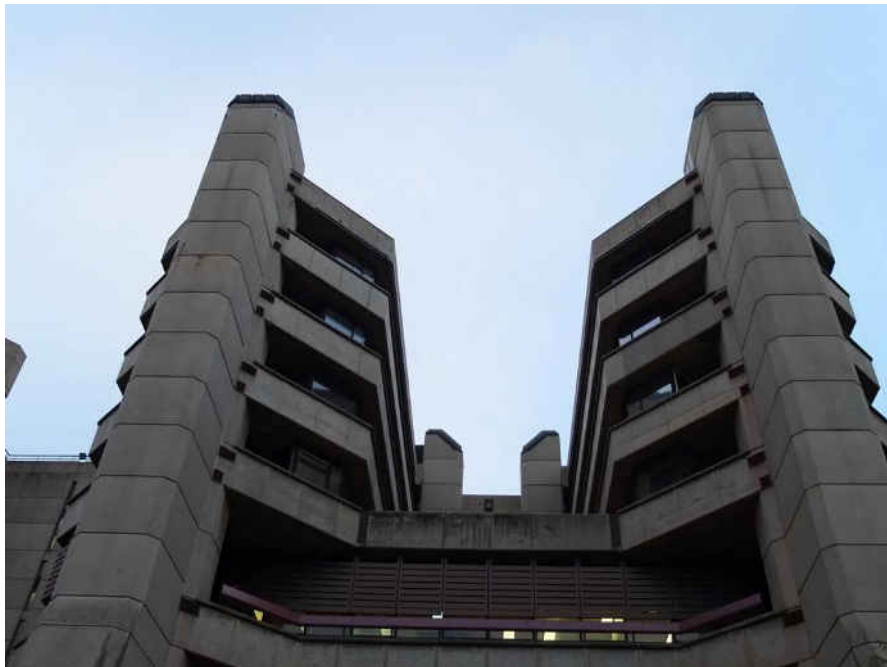
Fig. 46 Reinforced concrete pylons of main ring (Source: tsica heritage consultants, 2015)
