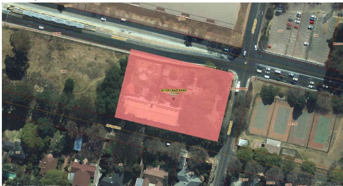
Fig. 61 The ATS-Theological Seminar building is located along the northern side of Richmond Avenue parallel to Kingsway Avenue (Source: City Council of Johannesburg, GIS map)
