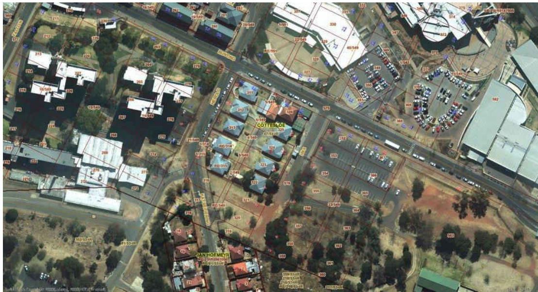
Fig. 15 Stands 311 to RE/315 and 322 to 326 constitutes a block bounded by Ibis Street, Bunting Road and Herold/ Katjeepering Street
