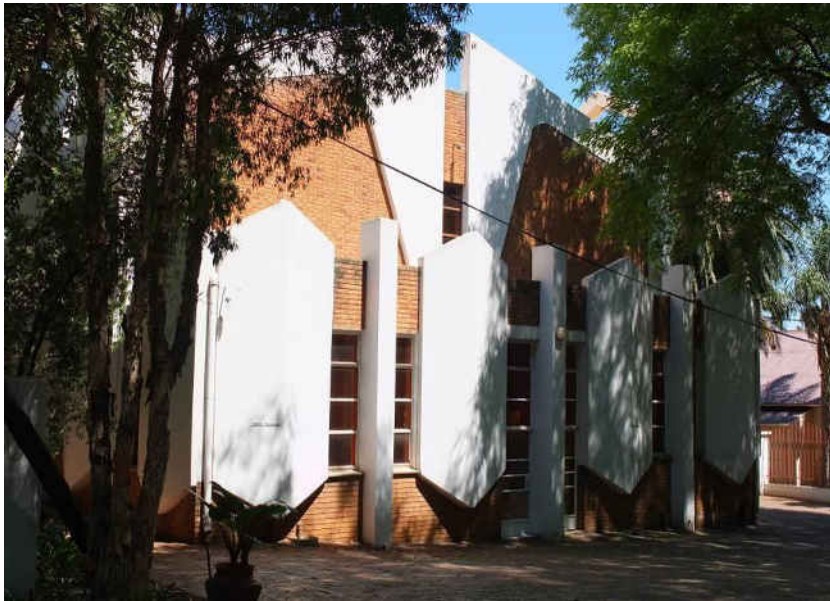
Fig. 62 East elevation with combined face brick and white painted concrete (Source: tsica heritage consultants, 2015)
