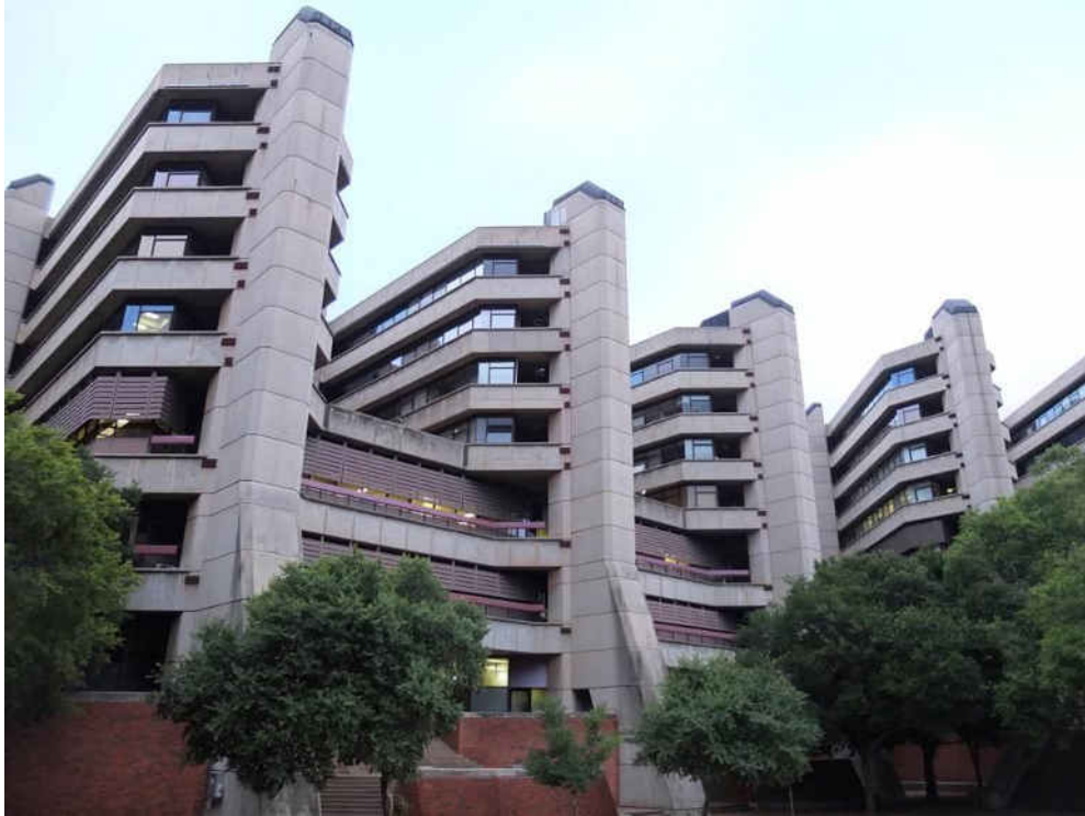
Fig. 47 Reinforced concrete pylons of main ring (Source: tsica heritage consultants, 2015)
