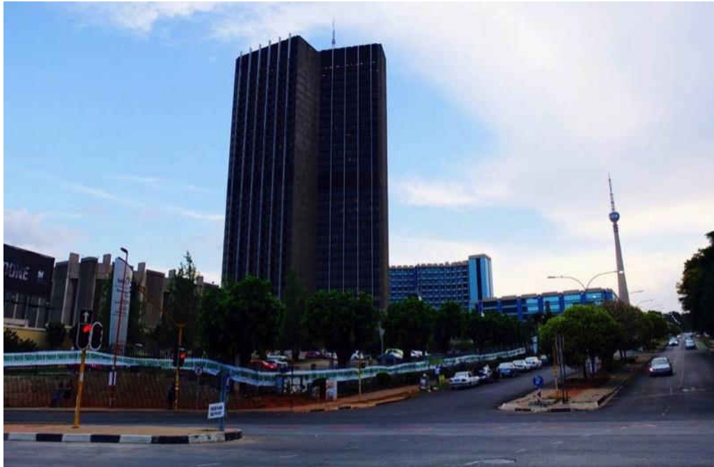
Fig. 39 North elevation, SABC complex (Source: tsica heritage consultants, 2015)
