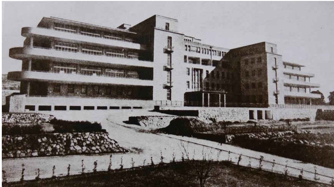
Fig. 34 The original block was designed following “Beaux Arts principles and symmetrically arranged around a recessed middle section” (Source: Van der Waal 1987:190)
