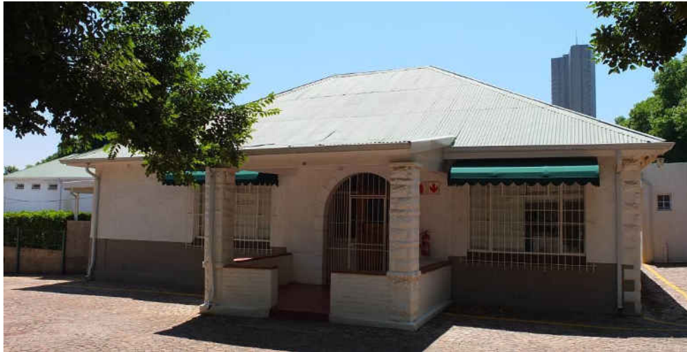
Fig. 60 Single storey residence on Stand 114 along Cookham Road forms part of the school ground (Source: tsica heritage consultants, 2015)
