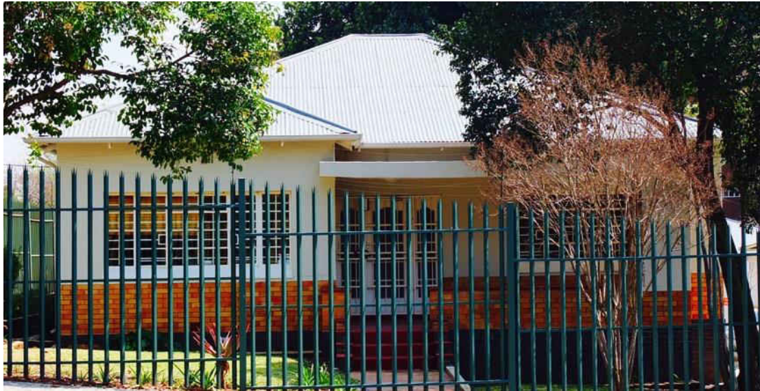
Fig. 25 Stand 322, 7 Ibis Street, Single storey, corrugated iron roof cottage on dark brown face brick plinth. East elevation (Source: tsica heritage consultants, 2015)
