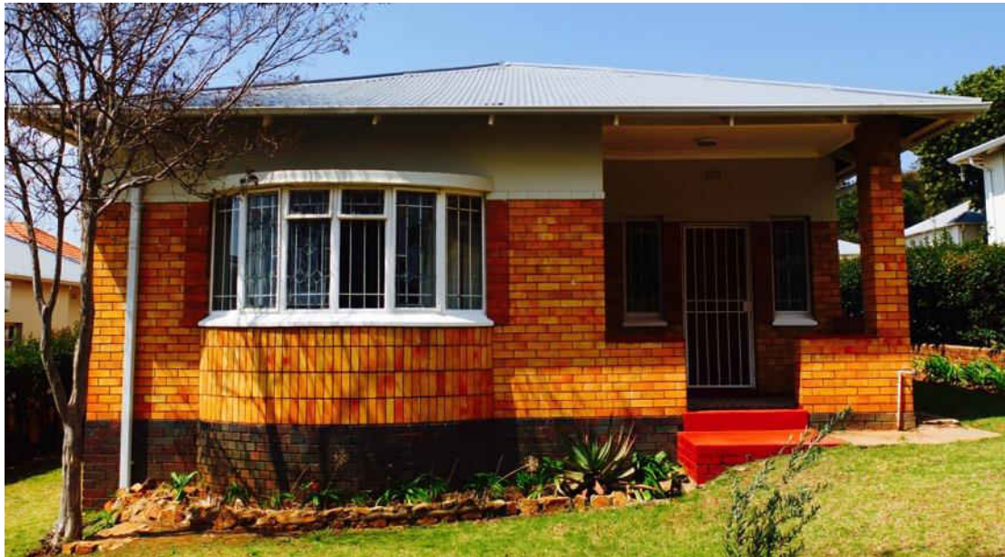
Fig. 24 Stand 313, 12 Herold Road, pitched roof corrugated iron roof, with yellow and dark brown face brick. West elevation (Source: tsica heritage consultants, 2015)
