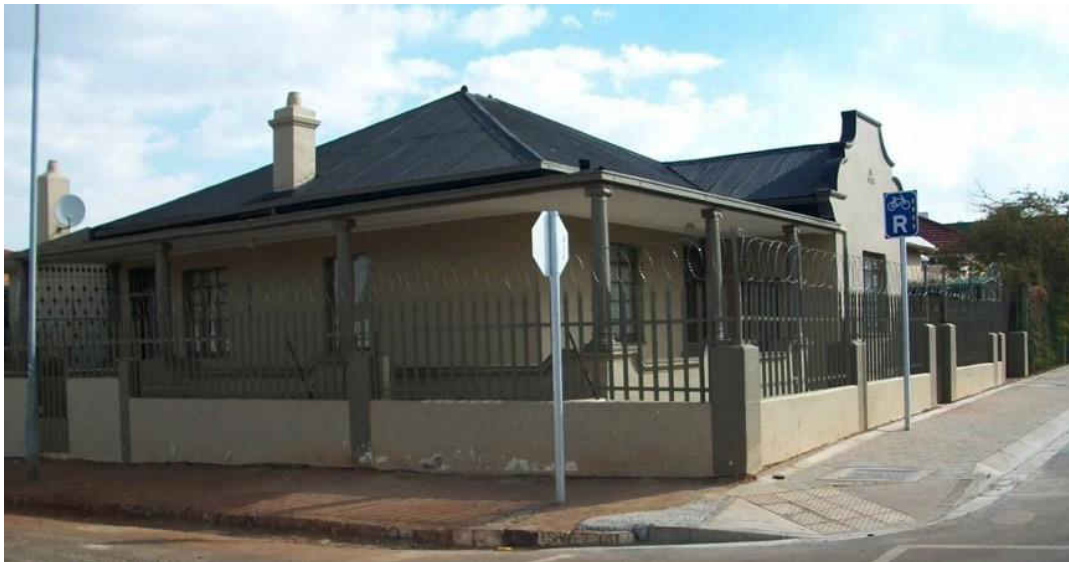
Fig. 181 Corrugated iron roof single storey house with side gable and corner stoep (Source: tsica heritage consultants, 2015)
