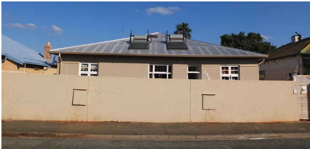
Fig. 233 Stand 69 along Barnes Road (Source: tsica heritage consultants, 2016)
