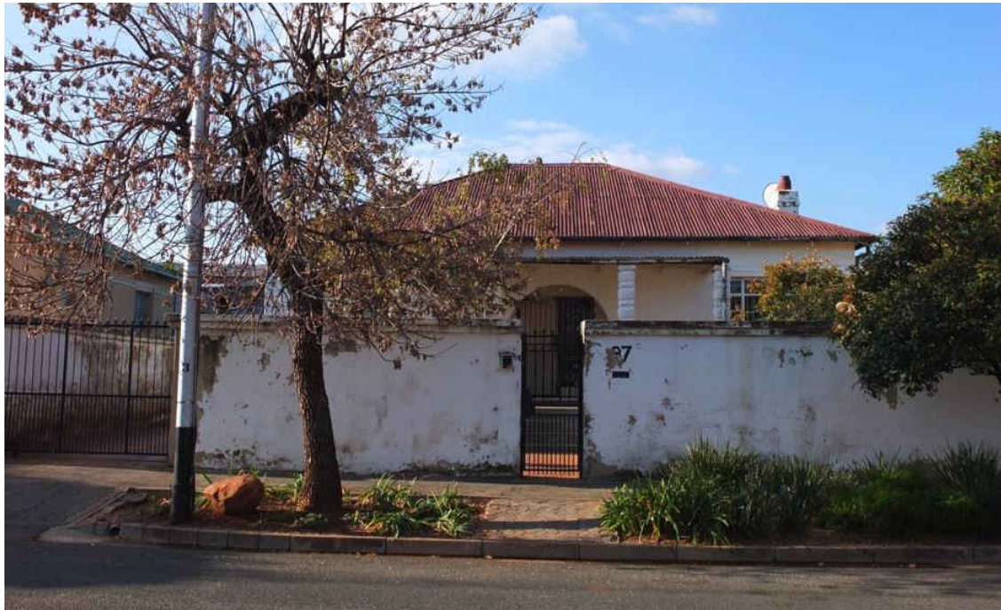
Fig. 127 Stand 143_south facing façade (Source: tsica heritage consultants, 2016)
