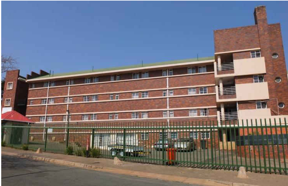
Fig. 276 Northern elevation facing onto Threadneedle street. Four-storey apartment building with cubistic balconies and rectangular and round steel windows (Source: tsica heritage consultants, 2015)
