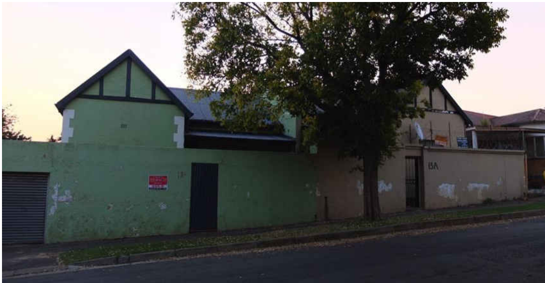
Fig. 268 Corrugated iron roof with side gables and central veranda, north elevation (Source: tsica heritage consultants, 2016)
