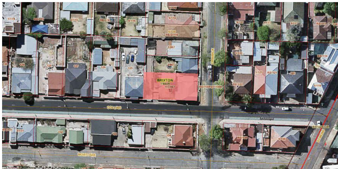
Fig. 266 Stand RE/867 on southern boundary of Beverley Road (Source: City Council of Johannesburg, GIS Map)
