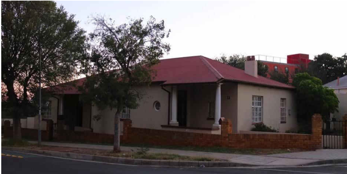
Fig. 193 Corrugated iron roof single storey semis with side stoeps (Source: tsica heritage consultants, 2016)
