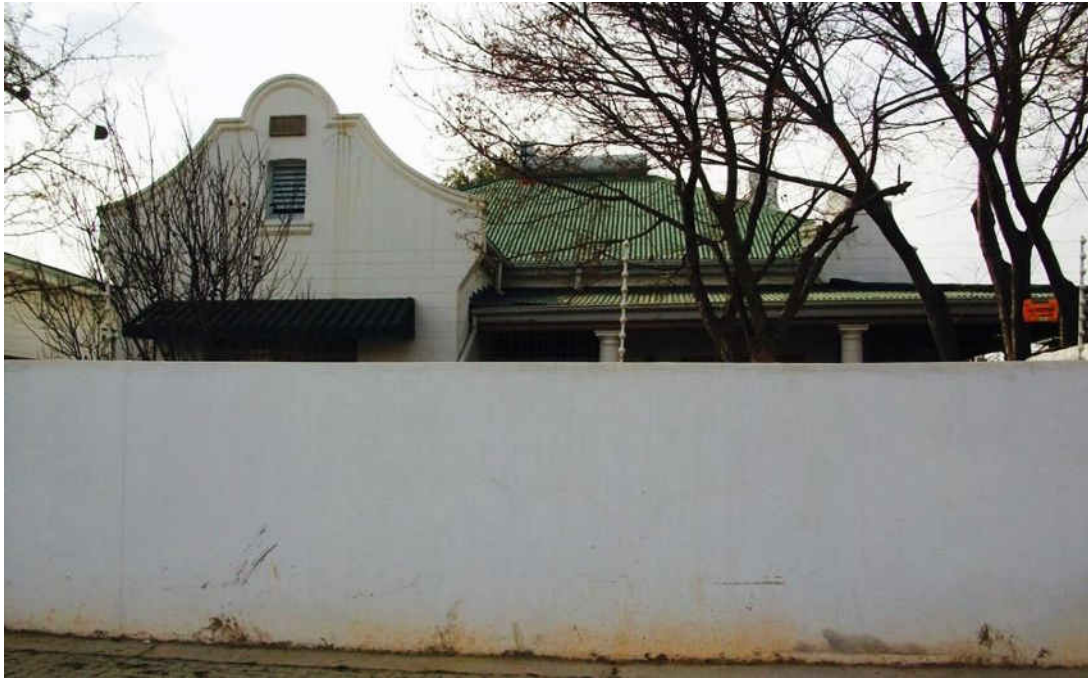
Fig. 189 Corrugated iron roof single storey house with side gable and corner stoep (Source: tsica heritage consultants, 2015)
