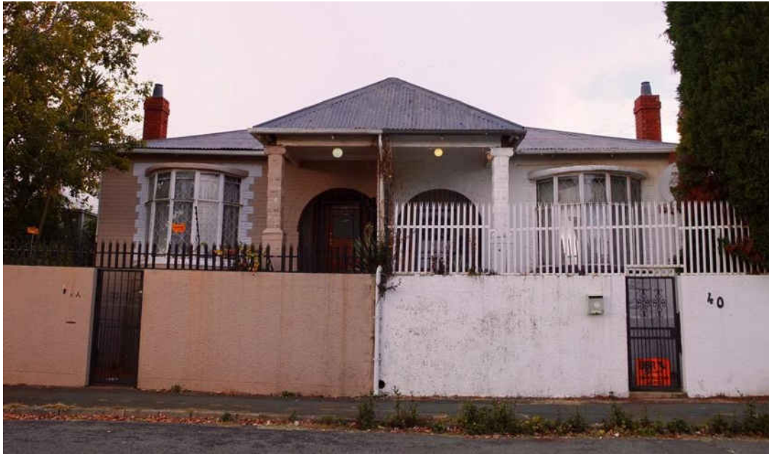
Fig. 174 Pair of semis_Corrugated iron roof with wrap central stoeps and side baywindows (Source: City Council of Johannesburg, GIS Map)
