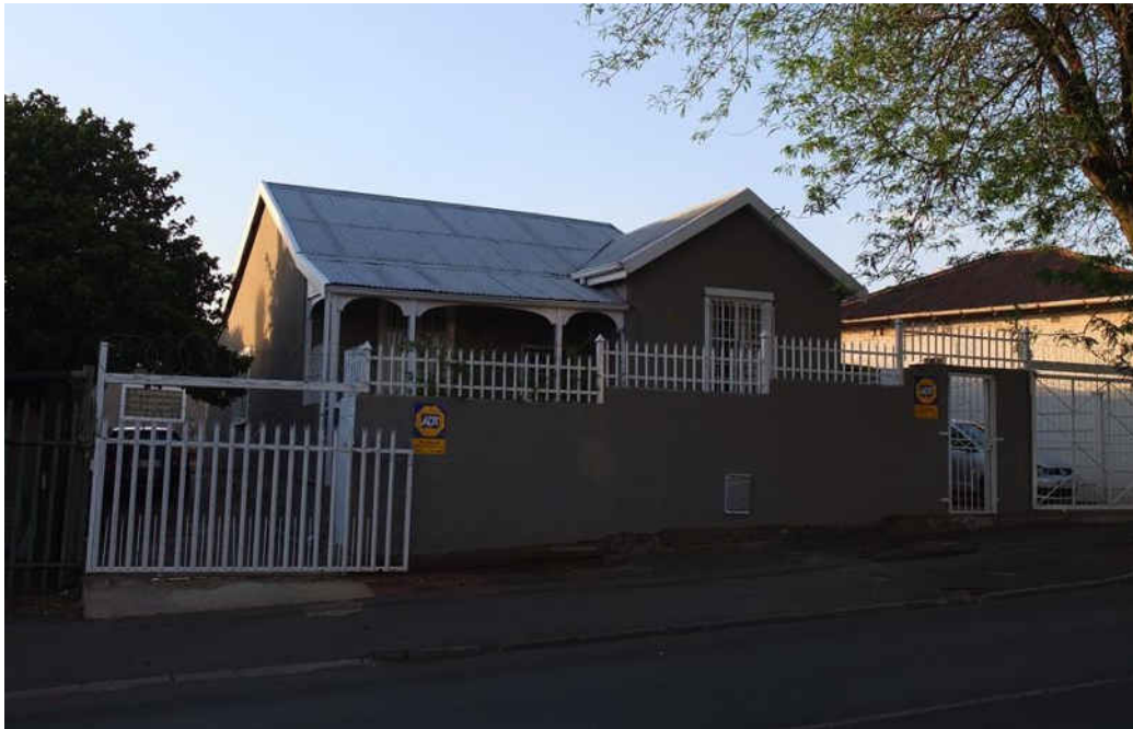
Fig. 219 Stand 1/76_Pitched roof corrugated iron house with side gable and stoep (Source: tsica heritage consultants, 2016)
