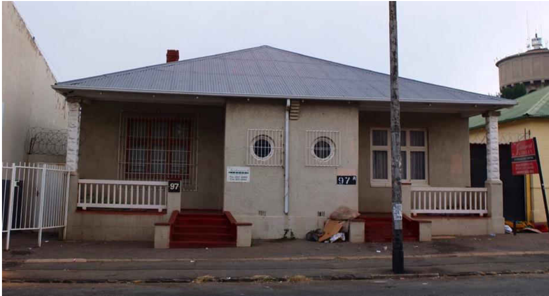
Fig. 159 Pair of semis with side stoeps, corrugated iron roofs and wooden window frames. (Source: tsica heritage consultants, 2015)
