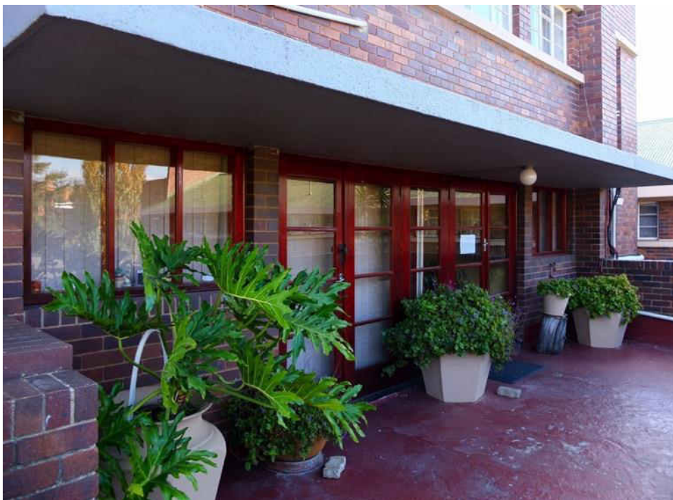
Fig. 279 Main entrance (Source: tsica heritage consultants, 2016)
