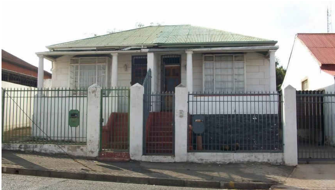
Fig. 145 Corrugated iron roof single storey semis with colonnaded stoeps (Source: tsica heritage consultants, 2015)
