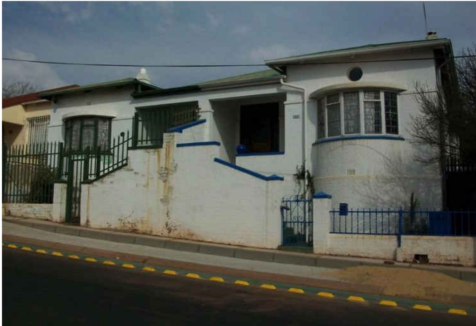
Fig. 178 Corrugated iron roof single storey semis (Source: tsica heritage consultants, 2015)
