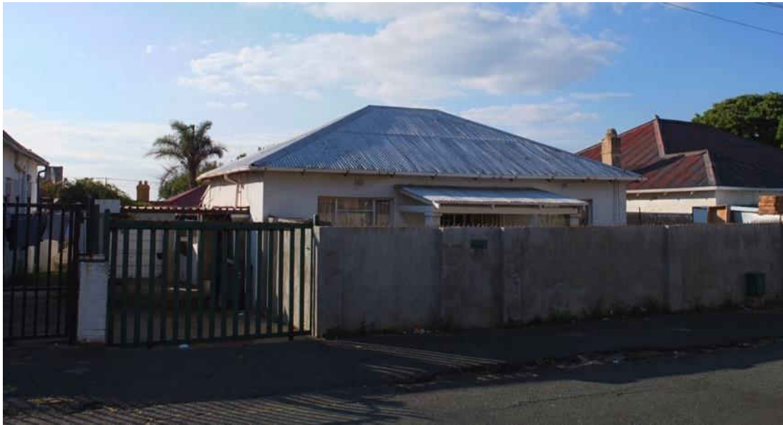
Fig. 310 Freestanding corrugated iron roof with central stoep (Source: tsica heritage consultants, 2016)
