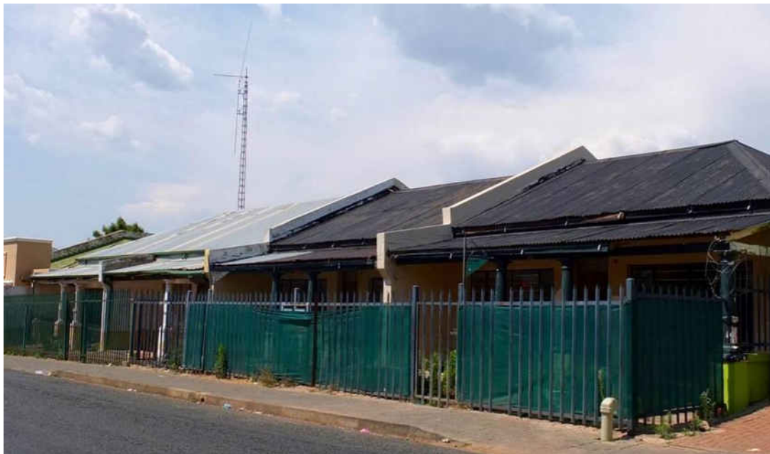
Fig. 167 Single storey corrugated iron roof row houses (Source: tsica heritage consultants, 2015)
