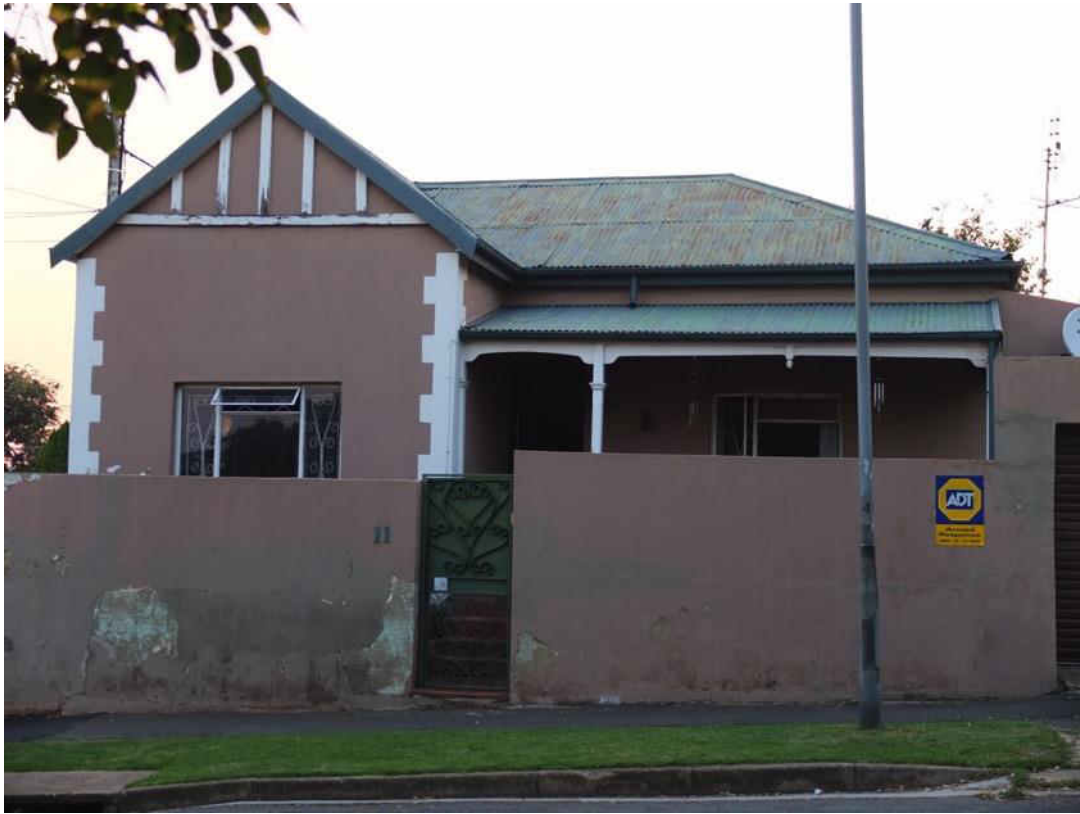
Fig. 267 Corrugated iron roof with side gables and central veranda, north elevation (Source: tsica heritage consultants, 2016)
