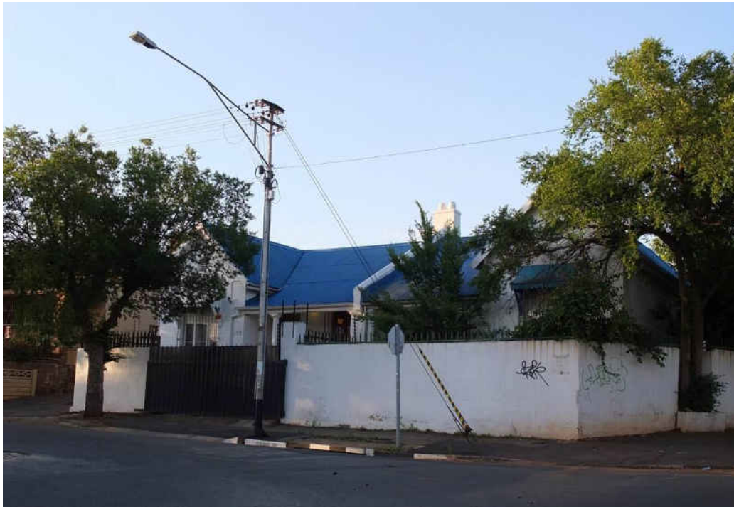
Fig. 217 Stand 72/6_Pair of semis on important streetscape where Symons & Fulham meet (Source: tsica heritage consultants, 2016)
