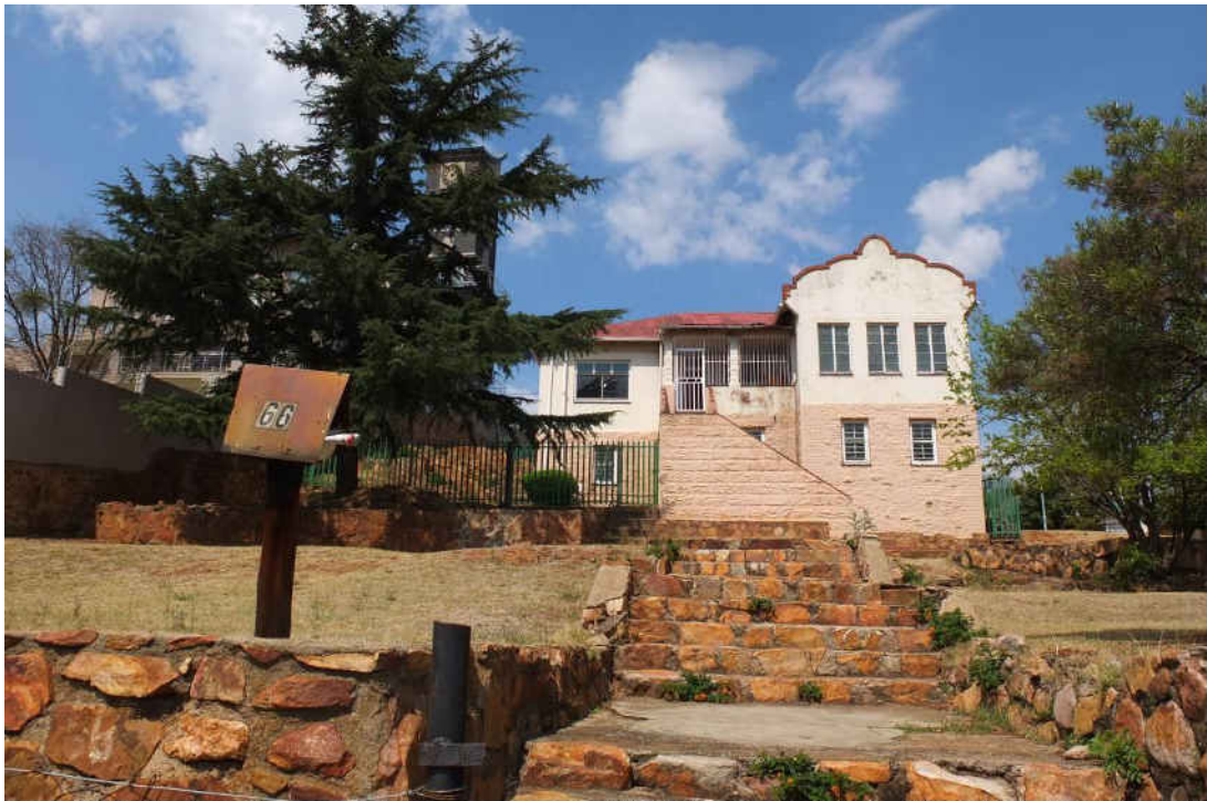
Fig. 282 Double storey residence with corrugated iron roof forms part of historical streetscape along Hampton Avenue along the boundary line towards Brixton (Source: tsica heritage consultants, 2015)
