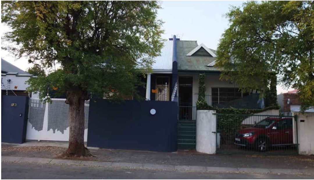
Fig. 202 Semis with fire wall, front stoeps and air vents (Source: tsica heritage consultants, 2015)
