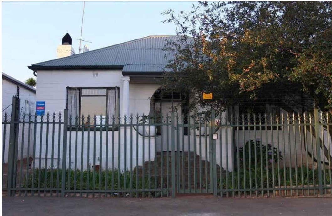
Fig. 199 Corrugated iron roof single storey house with central doorway and portico. (Source: tsica heritage consultants, 2015)
