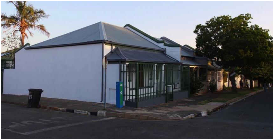
Fig. 274 Corrugated iron roof row housing (Source: tsica heritage consultants, 2015)
