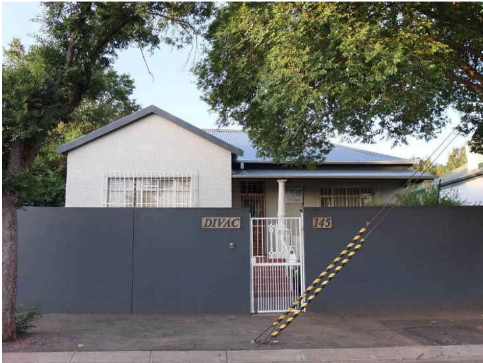
Fig. 196 Corrugated iron roof single storey house with side gable and corner stoep. (Source: tsica heritage consultants, 2015)
