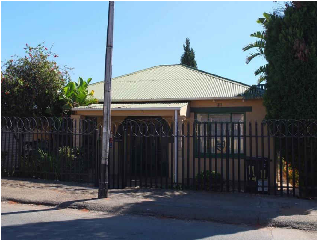
Fig. 305 Freestanding corrugated iron roof with central stoep (Source: tsica heritage consultants, 2016)
