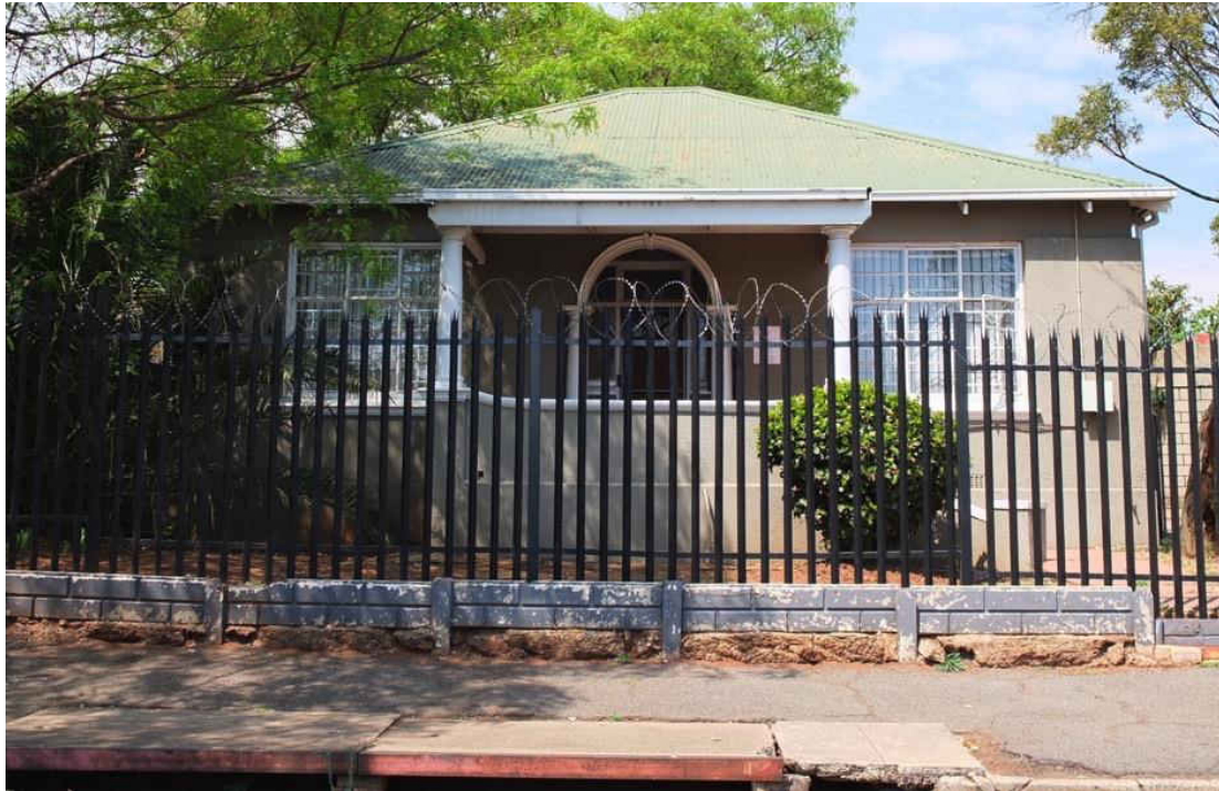
Fig. 147 Corrugated iron roof with central stoep (Source: tsice heritage consultants, 2016)
