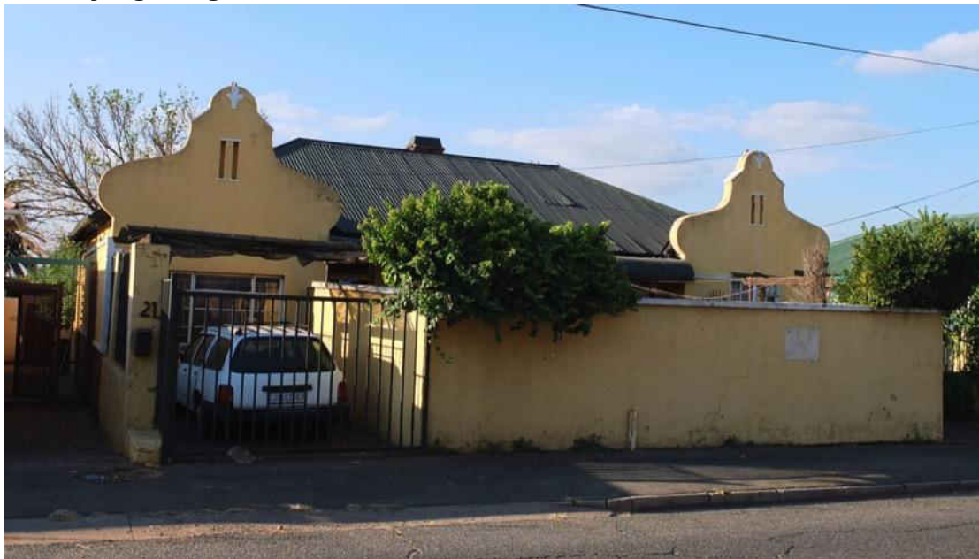
Fig. 297 Pair of semis on the northern boundary of Threadneedle Street (Source: tsica heritage consultants, 2016)
