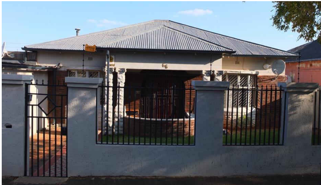
Fig. 136 Stand 159_north facing façade_baywindows & stoep intact. (Source: tsica heritage consultants, 2016)
