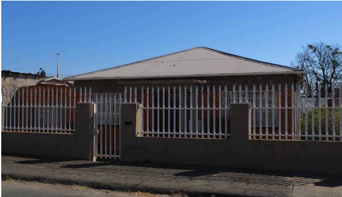
Fig. 299 Freestanding corrugated iron roof with central stoep (Source: tsica heritage consultants, 2016)
