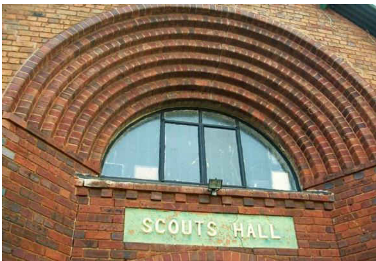
Fig. 84 Detail of brickwork above entrance door (Source: tsica heritage consultants, 2015)
