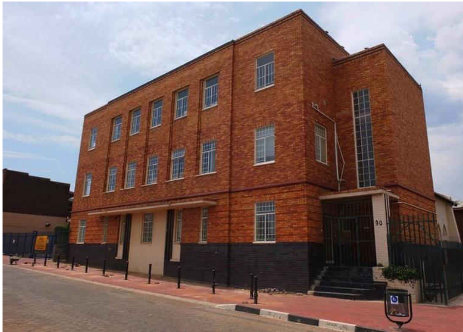
Fig. 59 West facing front façade of three storey yellow face brick with steel windows and black face brick plinth (Source: tsica heritage consultants, 2015)
