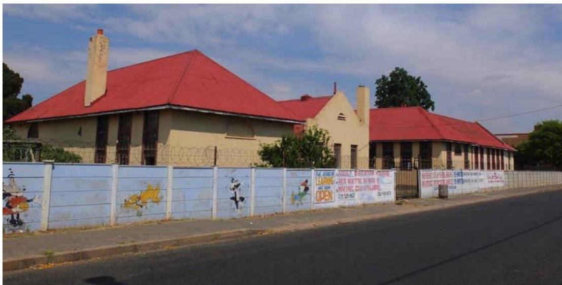
Fig. 89 View in western direction of main building on southern section of Caroline Street (Source: tsica heritage consultants, 2015)
