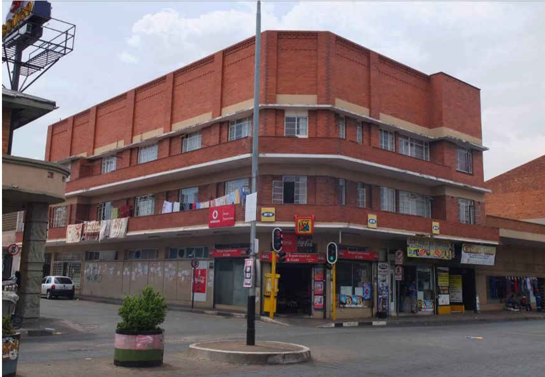
Fig. 36 Three storey commercial mixed use building with parapet along the northern side of High Street.
