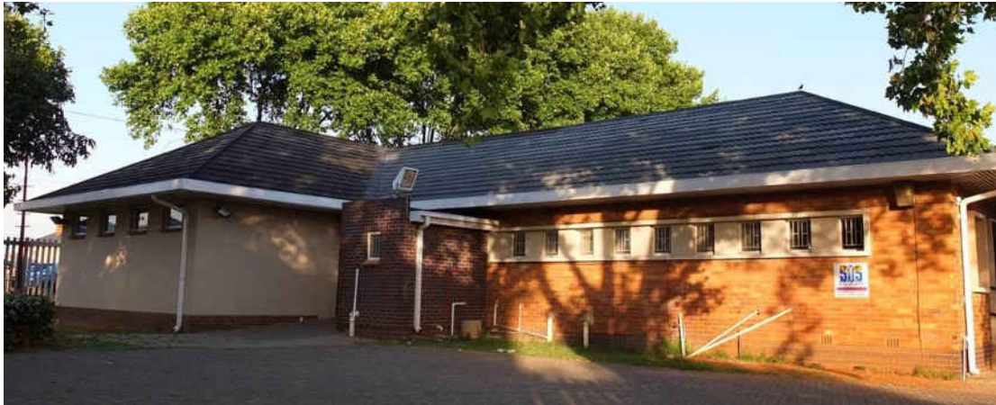
Fig. 69 Brixton Library, western elevation (Source: tsica heritage consultants, 2015)
