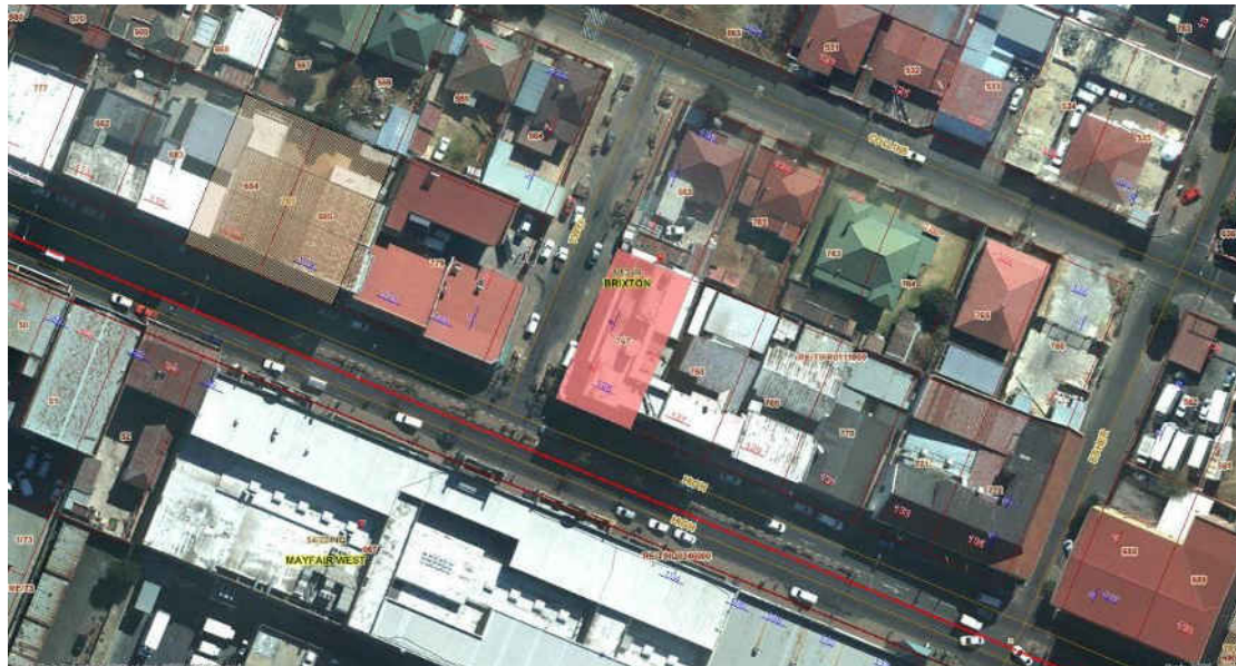
Fig. 37 Stand 767 is located along the northern side of High Street on the corner of High and Twyf Streets
