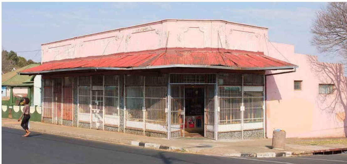
Fig. 44 Single storey corner shop building with corrugated iron veranda roofing and parapet wall above (Source: tsica heritage consultants, 2015)
