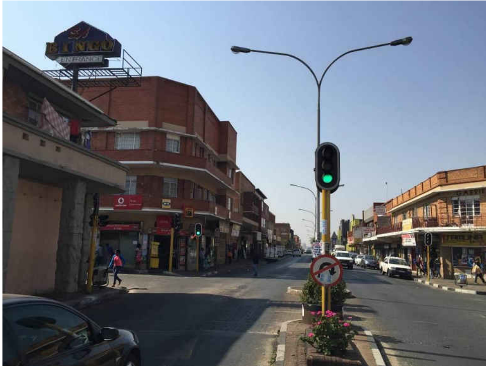
Fig. 23 Street scene with typical 1930s corner buildings with curbing in centre of roadway (Source: tsica heritage consultants, 2015)
