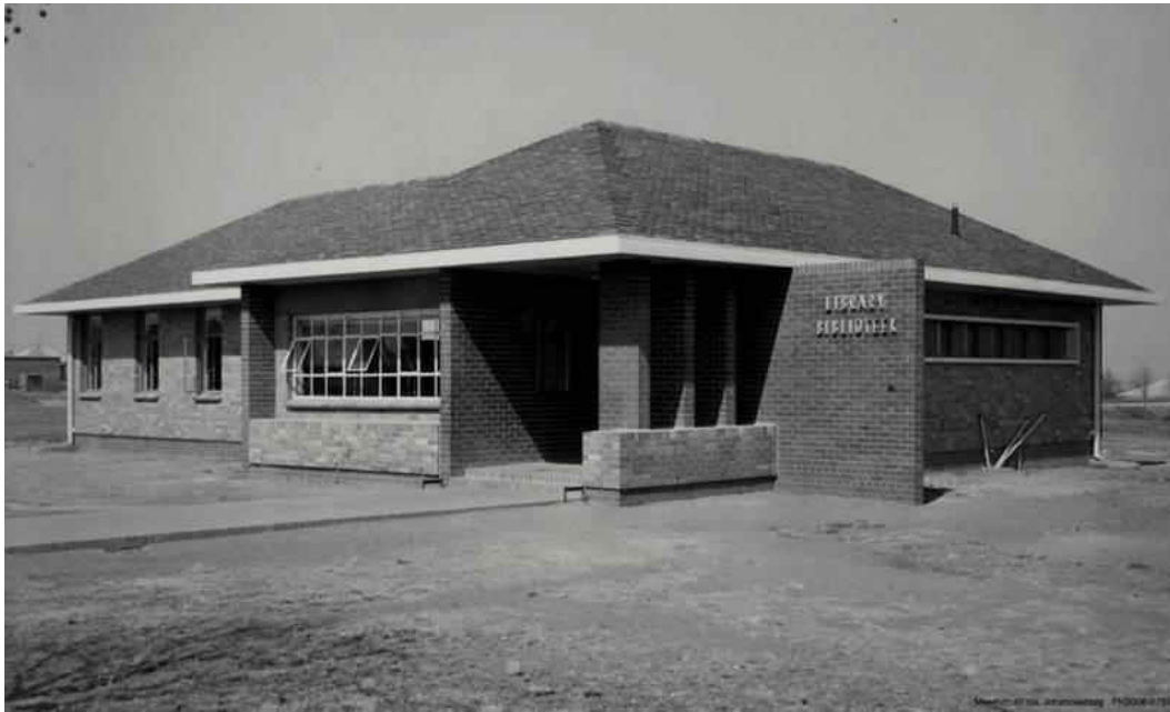
Fig. 14 Main entrance of Brixton Library shortly after completion in 1949 (Source: Museum Africa)
