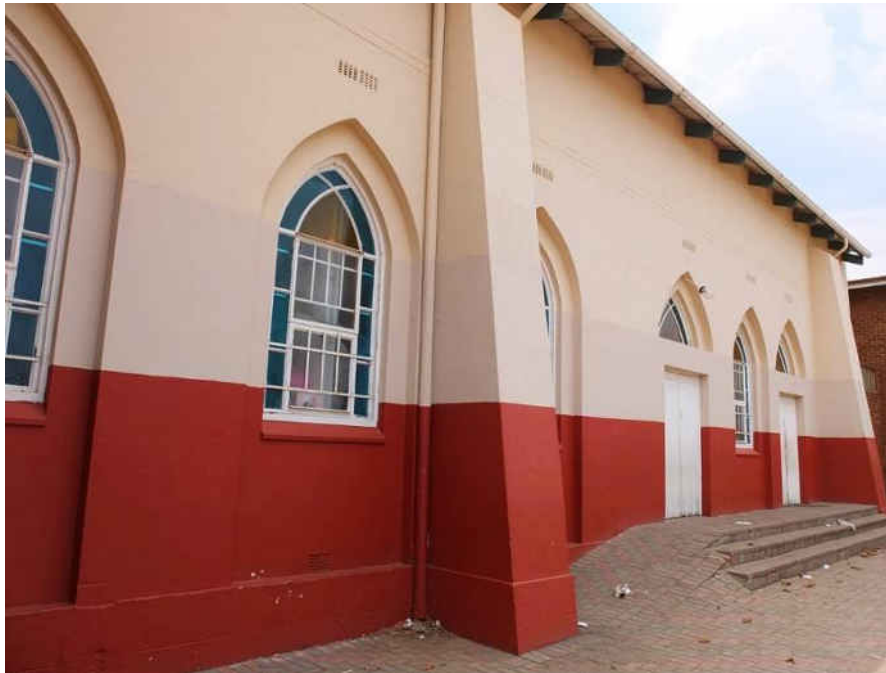
Fig. 60 Southern section of chapel showing gothic windows and buttresses (Source: tsica heritage consultants, 2015)
