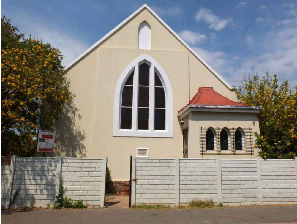
Fig. 104 North elevation of Wesleyan Church on Caroline Street (Source: tsica heritage consultants, 2015)
