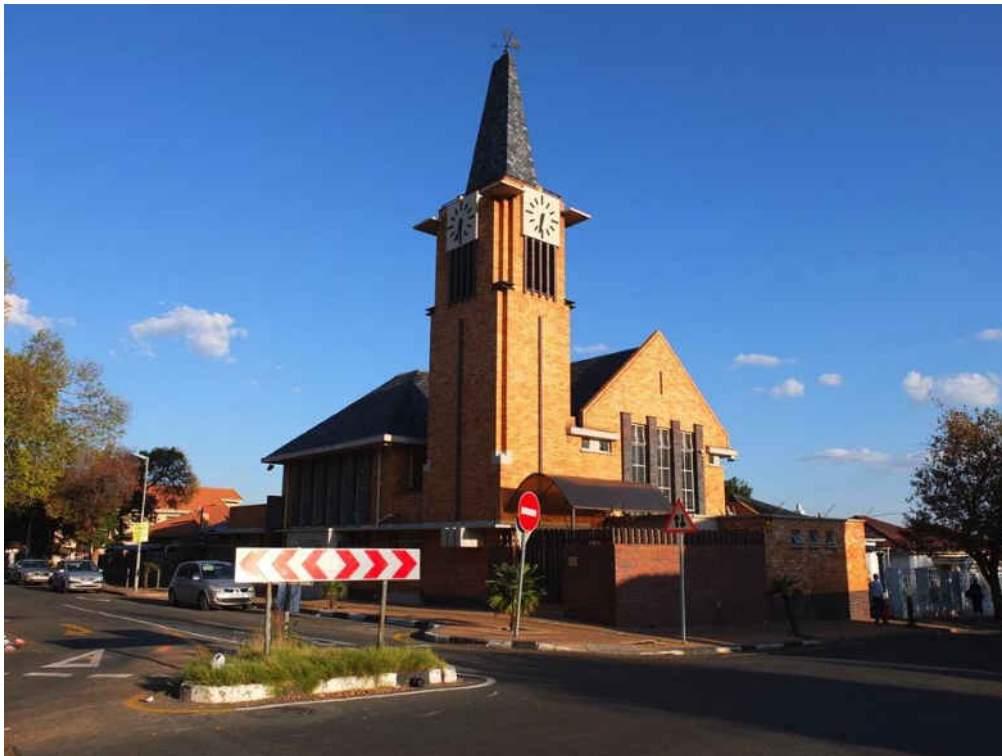
Fig. 100 View of church building from the north-western side (Source: tsica heritage consultants, 2016)
