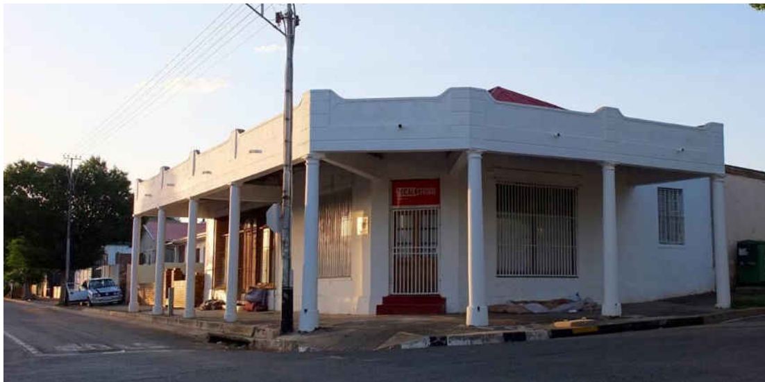
Fig. 53 Colonnaded corner shop with parapet and pitched corrugated iron roof prior to redevelopment. (Source: tsica heritage consultants, 2015)
