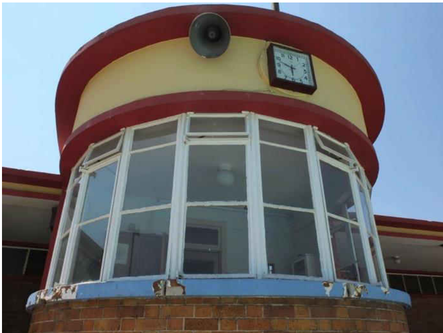
Fig. 79 Central watch tower (Source: tsica heritage consultants, 2015)
