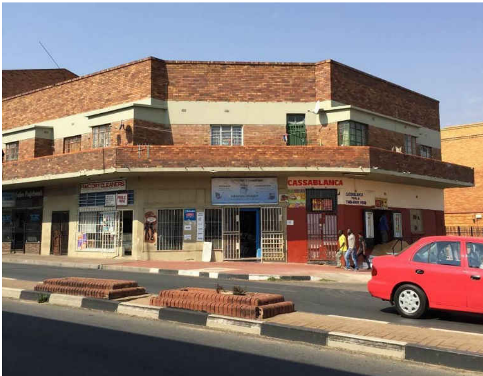
Fig. 22 Southern intersection of High Street (Source: tsica heritage consultants, 2015)
