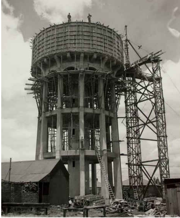
Fig. 10 Construction underway of the Brixton water tower, circa 1939 (Source: Museum Africa)
