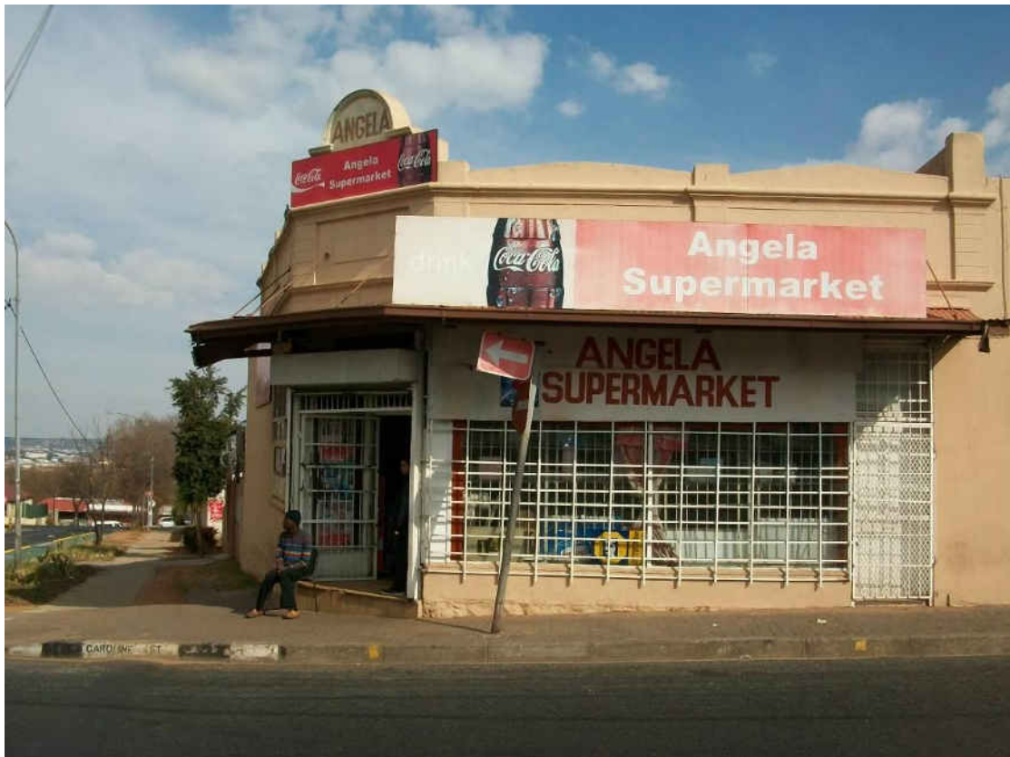
Fig. 41 Single storey corner shop building with corrugated iron veranda roofing and parapet wall above (Source: tsica heritage consultants, 2015)
