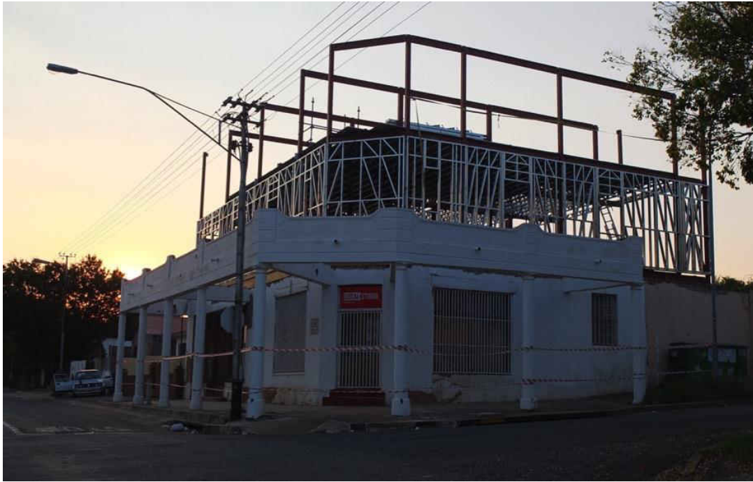
Fig. 54 Redevelopment of site underway_2016 (Source: tsica heritage consultants, 2016)
