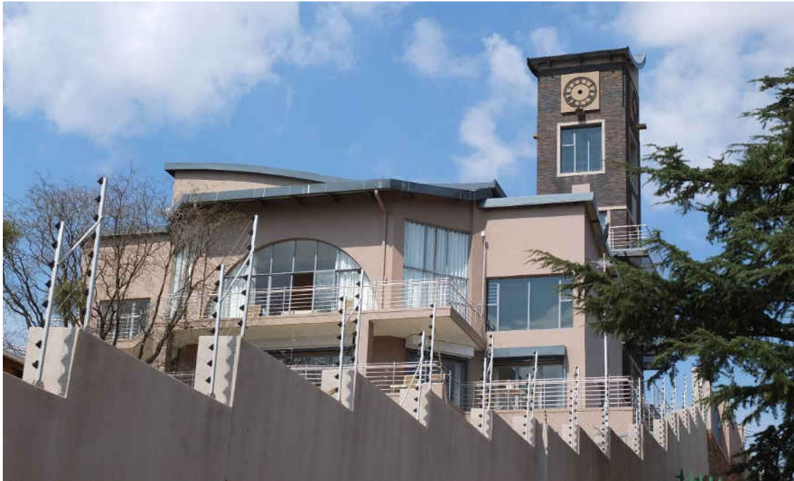
Fig. 116 View towards northern elevation of the Gerard Moerdyk church along Brixton ridge with converted façade and usage (Source: tsica heritage consultants, 2015)
