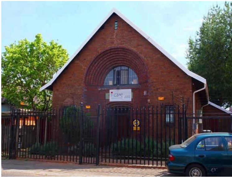
Fig. 82 Southern façade towards Caroline Street (Source: tsica heritage consultants, 2015)
