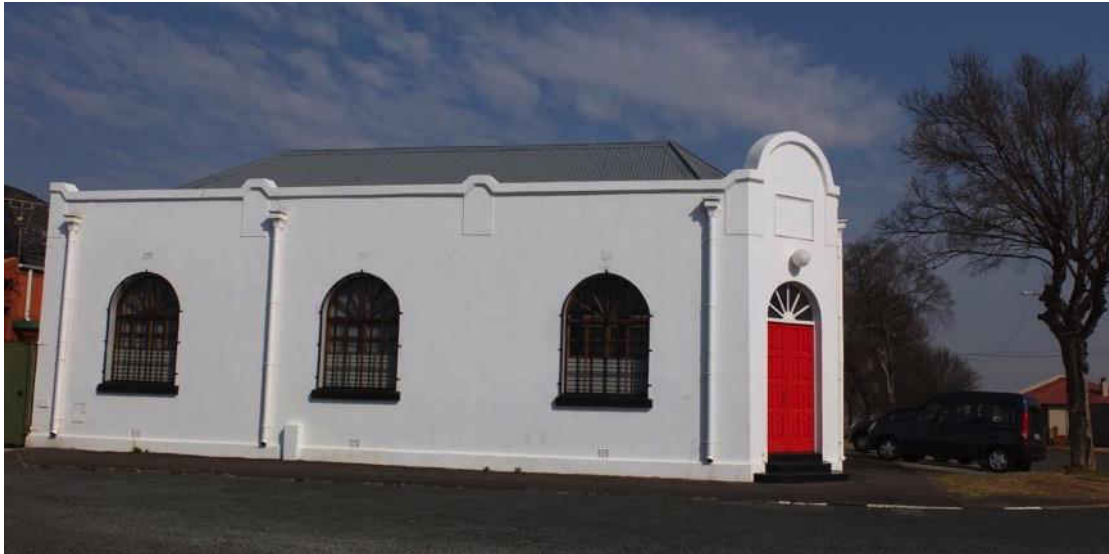
Fig. 56 Single storey original corner shop with parapet and pitched corrugated iron roof now used as architectural offices (Source: tsica heritage consultants, 2015)
