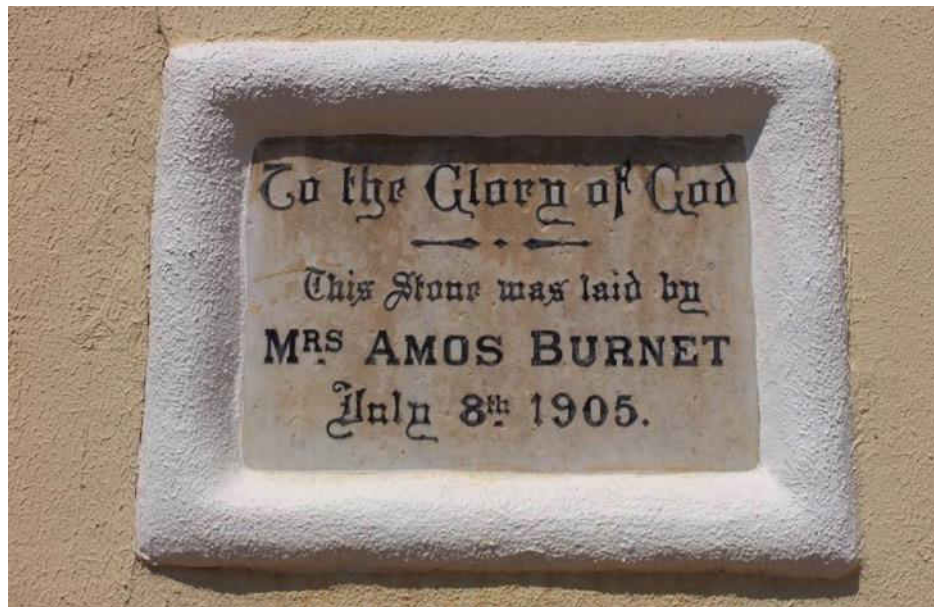
Fig. 103 Foundation stone from 1905 of the Church (Source: tsica heritage consultants, 2015)
