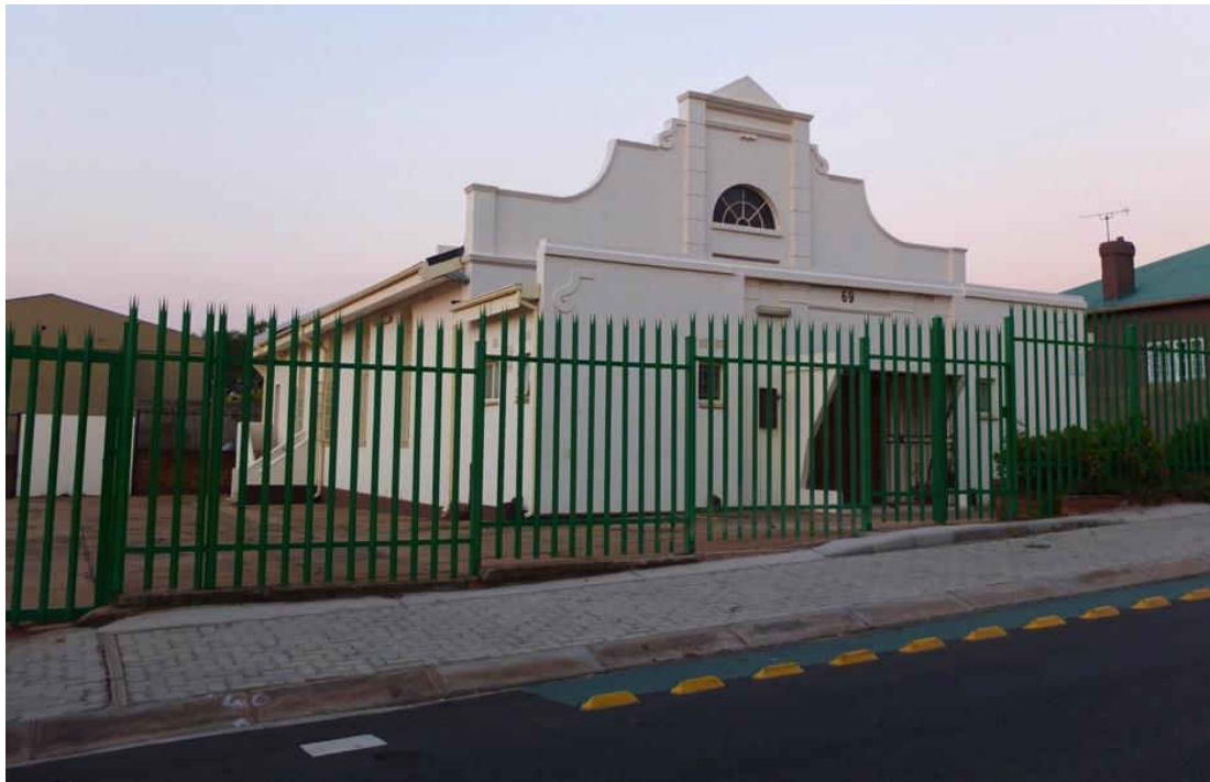
Fig. 112 South elevation along Fulham Road (Source: tsica heritage consultants, 2015)
