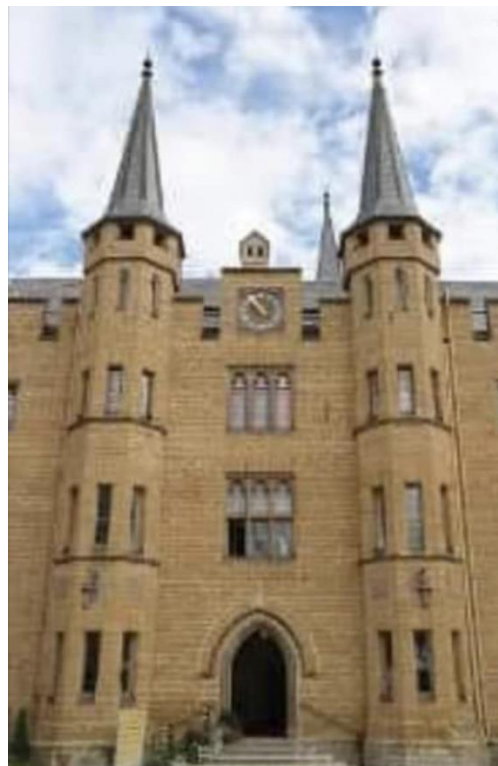
Hohenzollern Castle Facade
