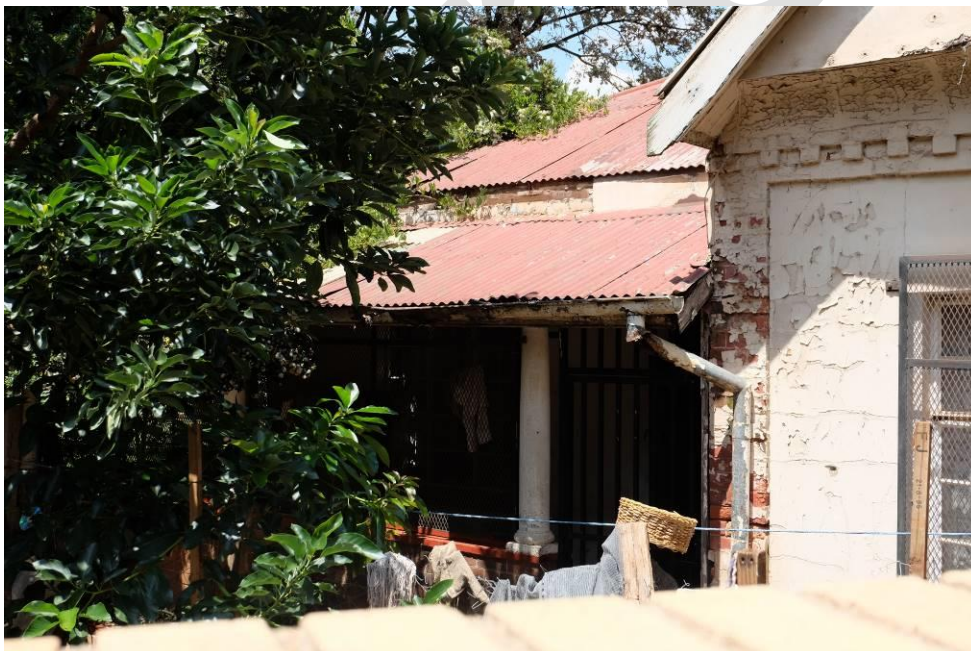
Fig. 39_Original park managers house along the eastern boundary line of Joubert Park next to the entrance gate, the building is in a very bad condition and is occupied by illegal residents
