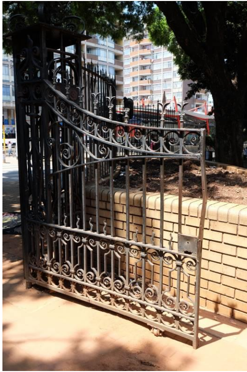
Fig. 71_Eastern entrance gate with decorative cast iron pillars and gates (Source: tsica heritage consultants, 2018)
