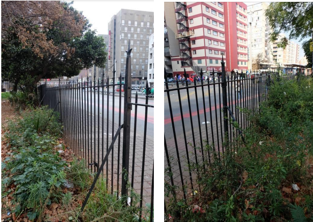
Fig. 74 & 75_Cast iron fencing all around Joubert Park_partly damaged or removed (Source: tsica heritage consultants, 2018)
