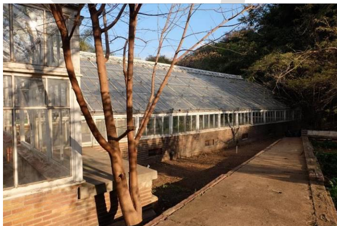
Fig. 41_Current state of Conservatory with partly broken glass and in urgent need of repair (Source: tsica heritage consultants, 2018)
