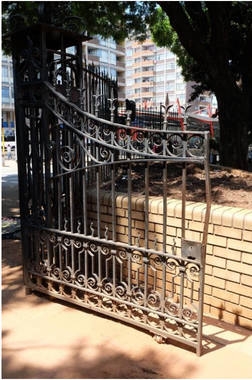
Fig. 24_Eastern entrance gate with decorative cast iron pillar and gates (Source: tsica heritage consultants, 2018)
