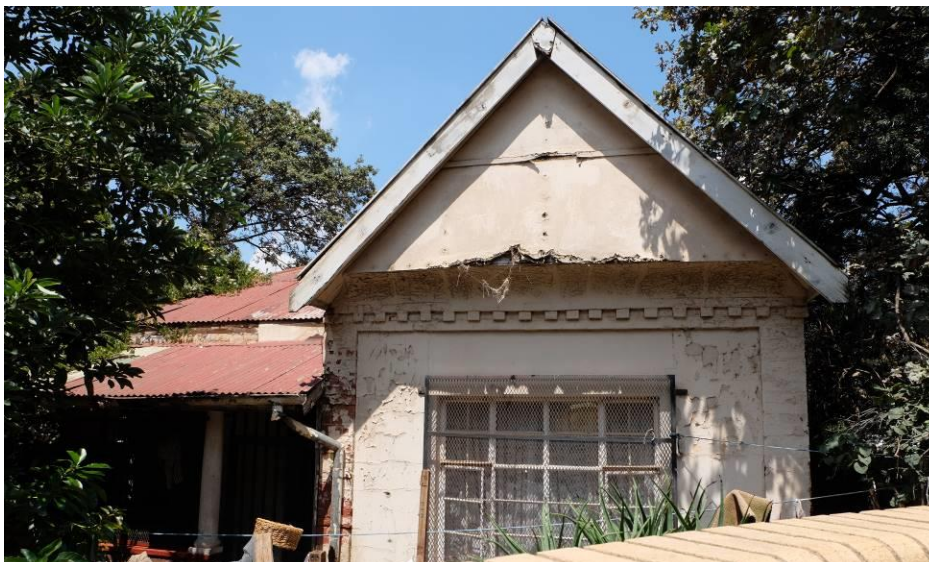
Fig. 53_Original Park Manager's house along the eastern boundary line of Joubert Park next to the western entrance gate, the building is in a very bad condition and is occupied by illegal residents
