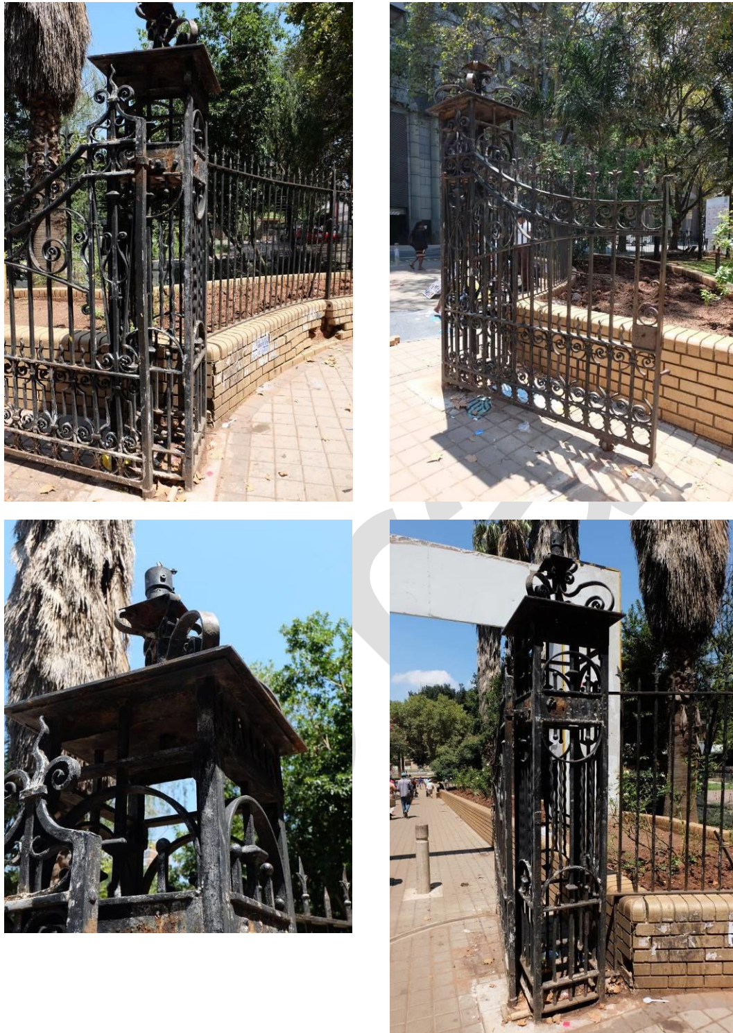
Fig. 20 to 23_Northern entrance gate with decorative cast iron pillar and gates (Source: tsica heritage consultants, 2018)
