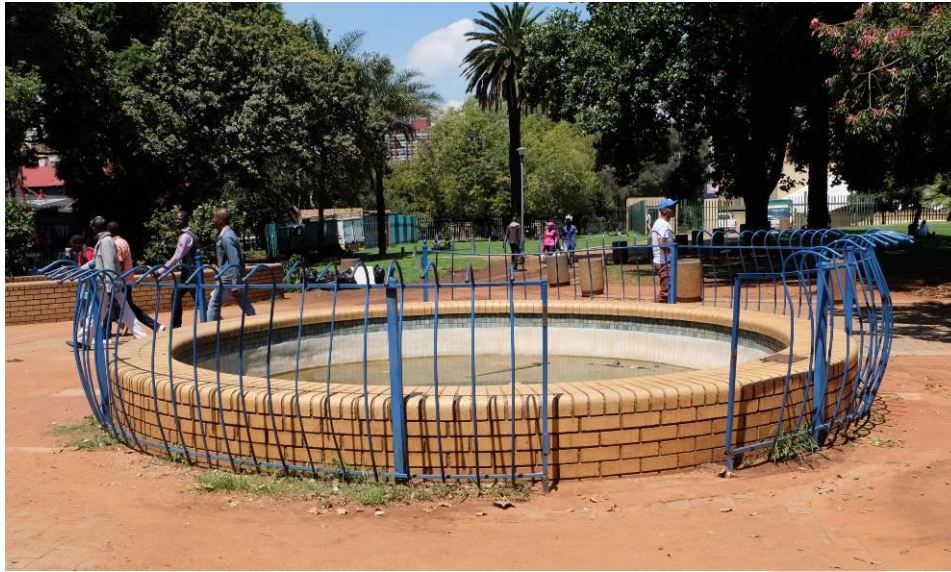
Fig. 36_One of the two fountains located along secondary axis in line with the main fountain, both fountains are in a very bad condition and not functional anymore (Source: tsica heritage consultants, 2018)
