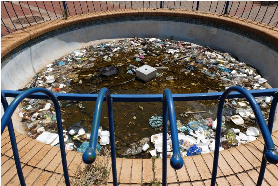
Fig. 37_One of the two fountains located along secondary axis in line with the main fountain, both fountains are in a very bad condition and not functional anymore (Source: tsica heritage consultants, 2018)
