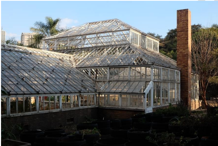
Fig. 40_Current state of Conservatory with partly broken glass and in urgent need of repair (Source: tsica heritage consultants, 2018)
