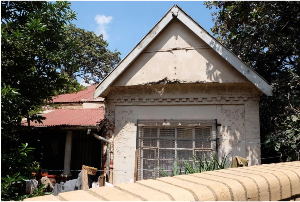
Fig. 38_Original park managers house along the eastern boundary line of Joubert Park next to the western entrance gate, the building is in a very bad condition and is occupied by illegal residents
