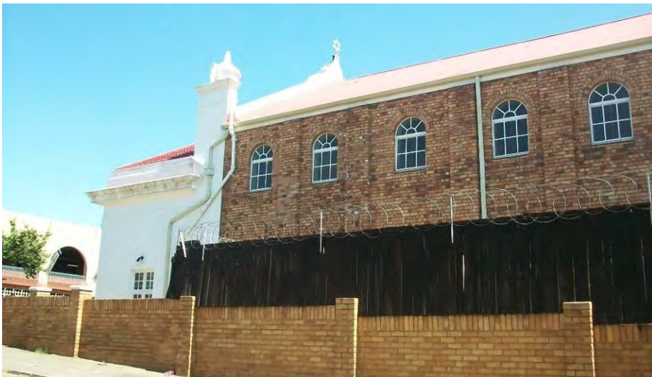
Fig. 92 Side elevation showing a combination of plastered front façade and a facebrick side elevation (Source: tsica heritage consultants, 2015)
