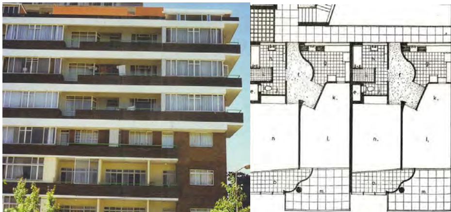
Fig. 13 (Left) University Gate, Braamfontein, 1961 by Clive Chipkin_large deep balconies with box food planting areas. Projections act as summer sun protection. (left)
