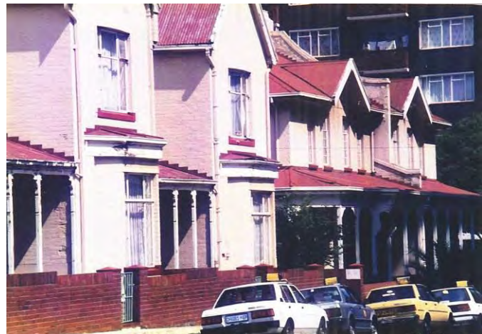
Fig. 25 & Fig. 26 Berea Fire Station 1910; adjacent architecture with reference to Victorian terraces of a decade earlier (Photographs: Clive Chipkin)
