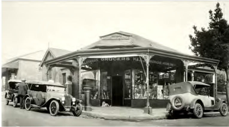
Fig. 5 Corner shop built in 1905 along 7th Street and 3rd Avenue in Melville, cast iron columns supporting the roof structure (Source: Museum Africa)
