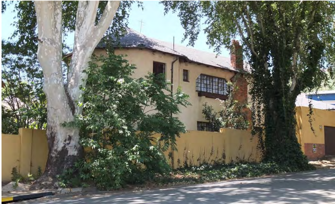
Fig. 186 Double storey slate tiled roofed residence in close proximity to Louis Botha Avenue in Fellside (Source: tsica heritage consultants, 2015)
