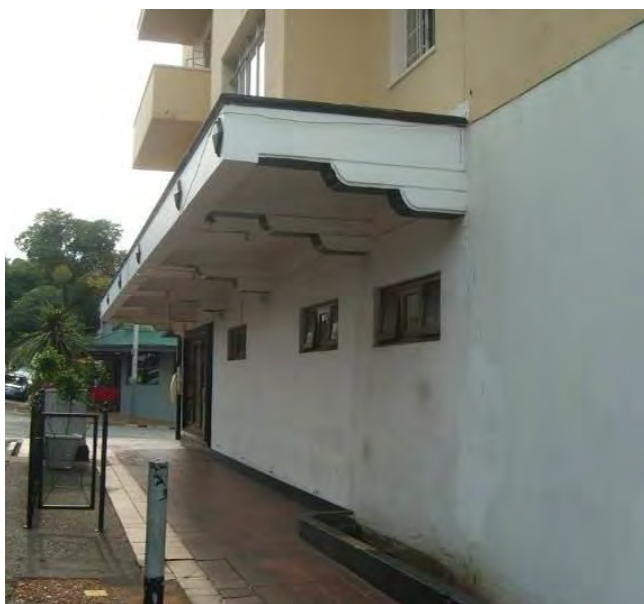
Fig. 6 Melville Mansions, 7 th Street in Melville_example for reinforced concrete cantilever, for Art Deco buildings slabs were supported on brackets with stepped or rounded edge forms. (Photograph: tsica heritage consultants, 2010)
