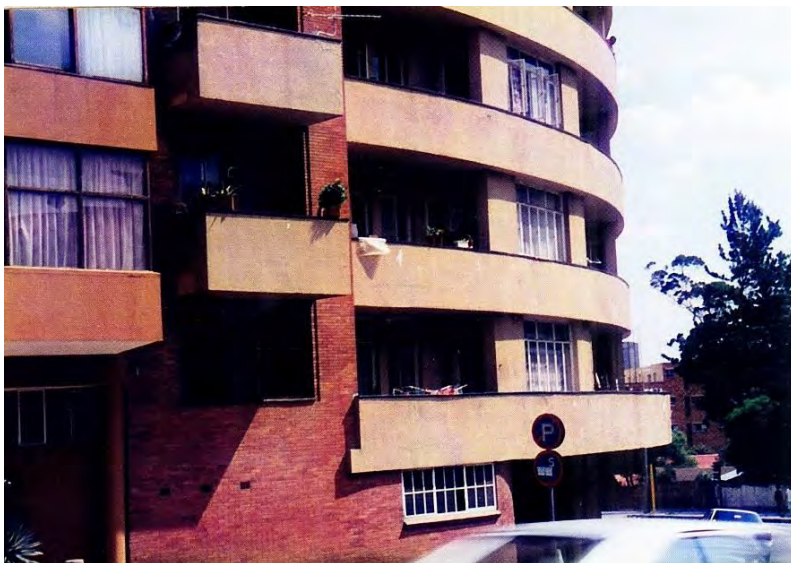
Fig. 29 Royal Crescent (right) on the curve; Reading Court (left) which is a major example of a Modern Movement building, restoration work is needed (Photograph: Clive Chipkin)
