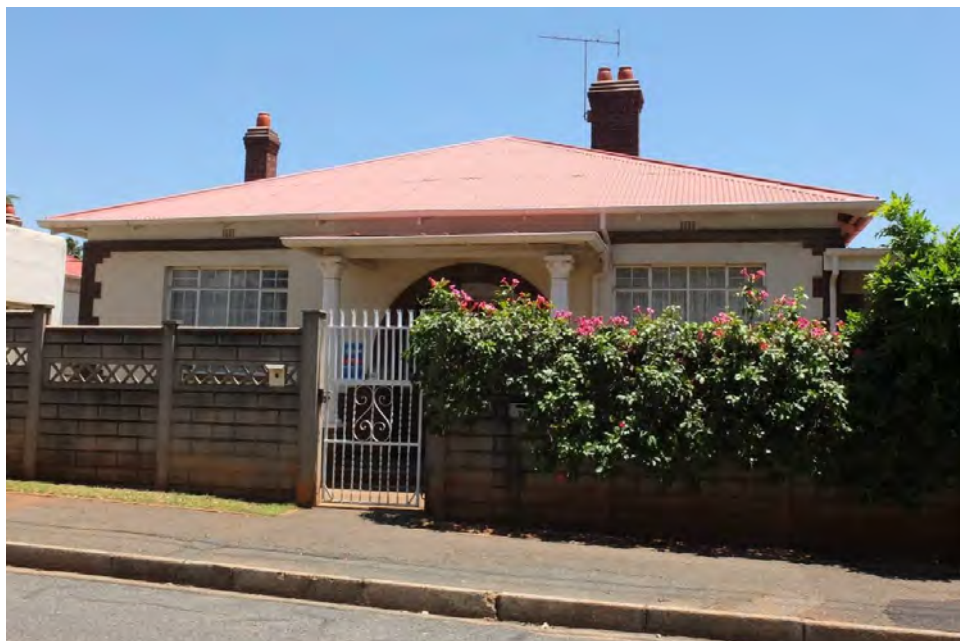
Fig. 183 Single storey residence with corrugated iron roofing and centrally located front stoep covering the arched main entrance, face brick detailing like building edges and arched entrance are still in very good condition (Source: tsica heritage consultants, 2015)
