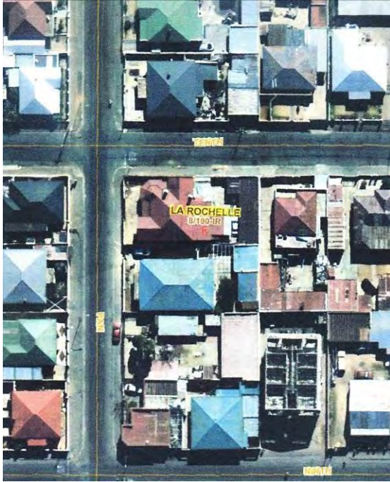
Fig. 43 La Rochelle_hipped roof houses with stoeps facing street, disregarding climate orientation. There is no tradition of atriums or courts_only small, separate rectangular houses placed in the middle of the stand
