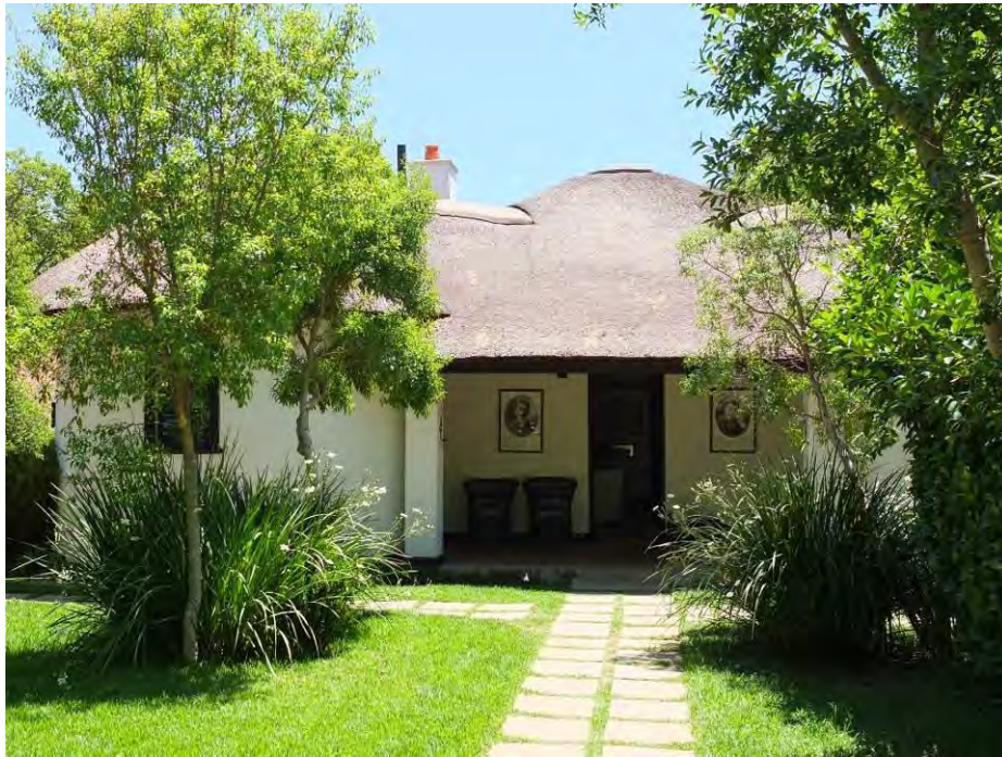
Fig. 213 View towards the main entrance of The Kraal building with the two rondavels used as bedrooms on either side (Source: tsica heritage consultants, 2015)
