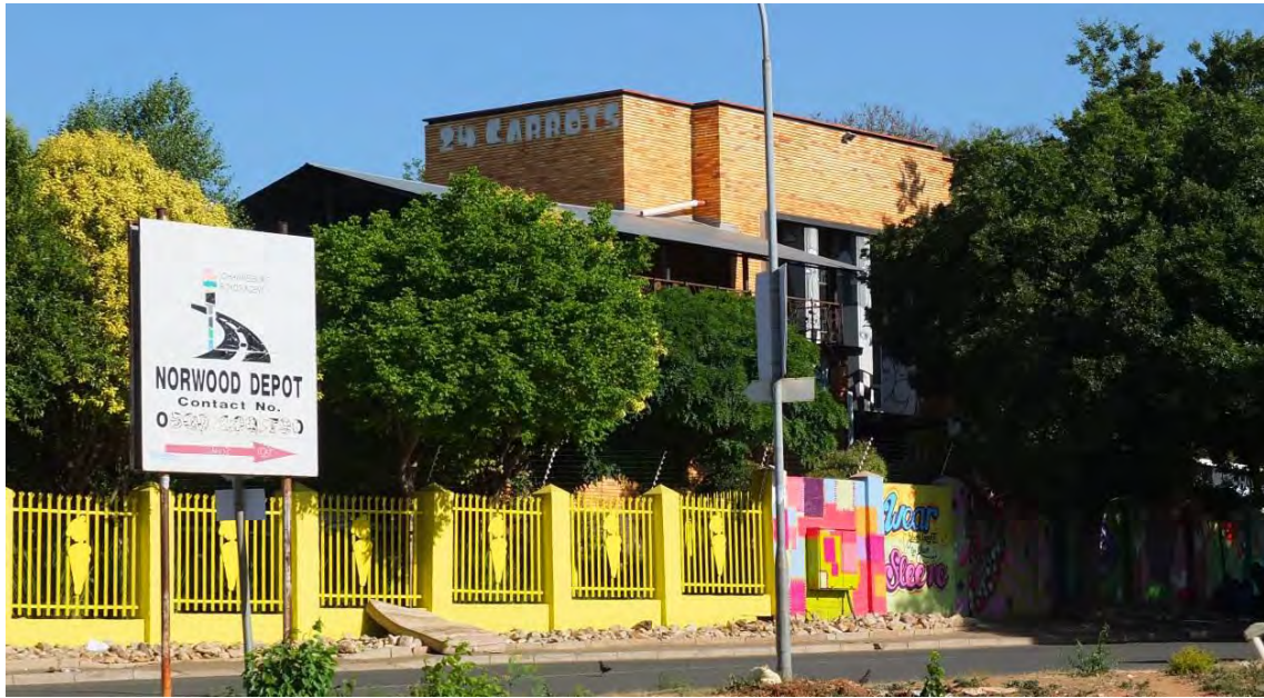
Fig. 223 View towards the main entrance of The Kraal building with the two rondavels used as bedrooms on either side (Source: tsica heritage consultants, 2015)
