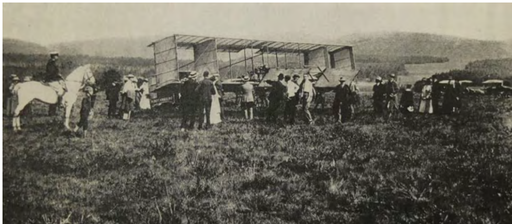
Fig. 197 Sydenham was home to an airfield in the 1910s from where Alfred Kimmerling made a number of notable flights
