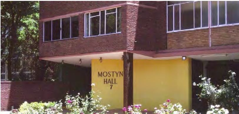
Fig. 34, Fig. 35 & Fig. 36 Generally 5 floors (including ground floor parking) with Princess Towers set back for eight floors (Photographs: Clive Chipkin)
