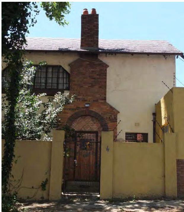
Fig. 187 Main entrance area with face brick decoration and chimney above along Unity Street (Source: tsica heritage consultants, 2015)
