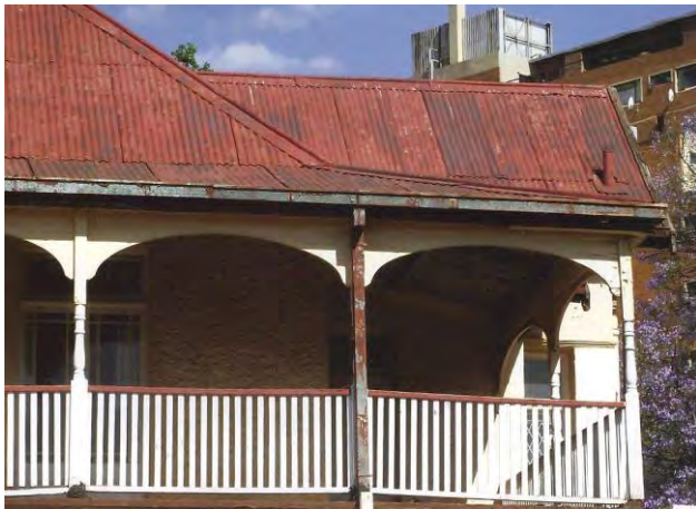
Fig. 23 Park Lane_Victorian colonial residence with perimeter verandah and steep corrugated iron roofing. Once a prominent double storey landmark off the old wagon road to Pretoria, via Halfway House (Photograph: Clive Chipkin)
