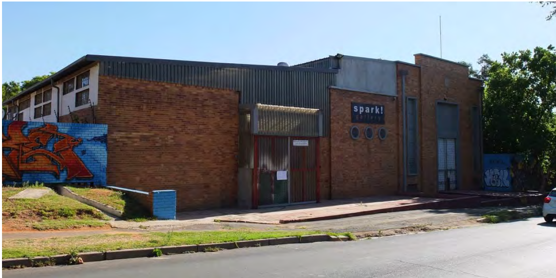
Fig. 234 Spark Gallery Originally used as the electrical substation of the City of Johannesburg along the southern side of Louis Road in Orchards (Source: tsica heritage consultants, 2015)
