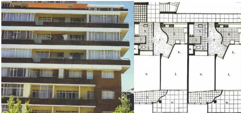
Fig. 180 (Left) University Gate, Braamfontein, 1961 by Clive Chipkin_large deep balconies with box food planting areas. Projections act as summer sun protection. (left)
