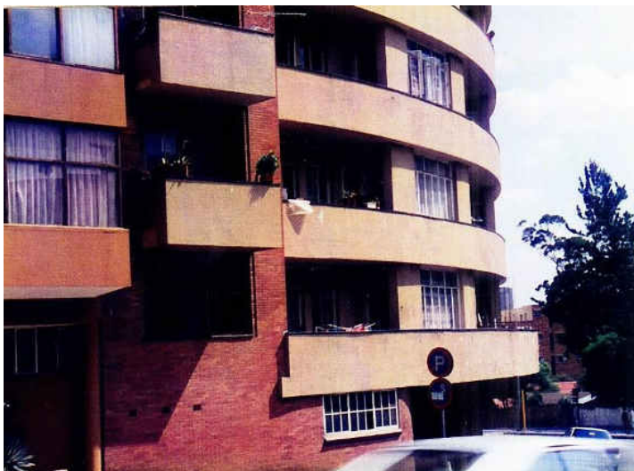
Fig. 196 Royal Crescent (right) on the curve; Reading Court (left) which is a major example of a Modern Movement building, restoration work is needed (Photograph: Clive Chipkin)
