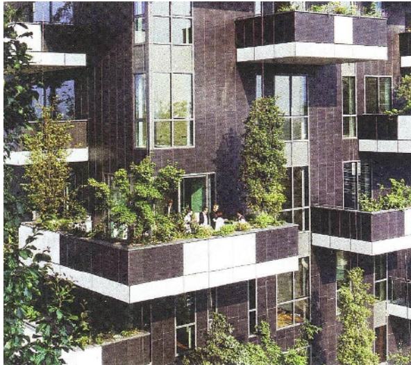
Fig. 179 Balconies as plant areas. Bosco Verticale, Milan. Architect: Boeri Studio. (Source: Earthworks journal, Issue 24/2015)
