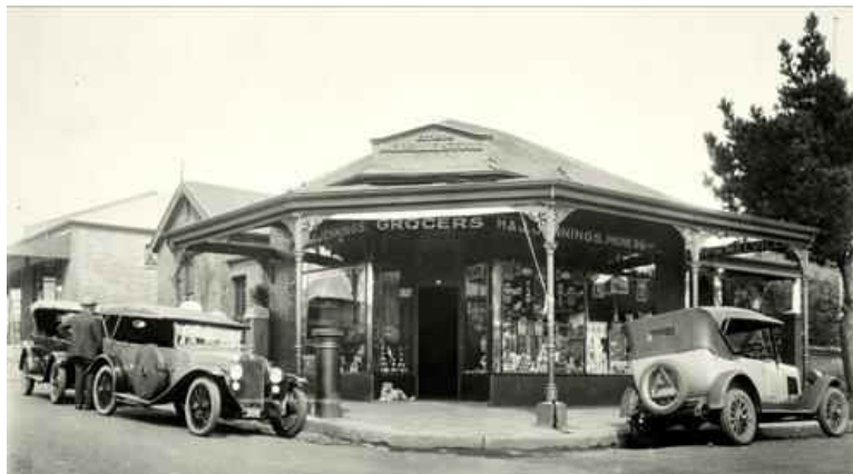
Fig. 172 Corner shop built in 1905 along 7th Street and 3rd Avenue in Melville, cast iron columns supporting the roof structure (Source: Museum Africa)
