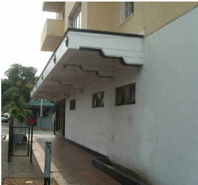
Fig. 323 Melville Mansions, 7 th Street in Melville_example for reinforced concrete cantilever, for Art Deco buildings slabs were supported on brackets with stepped or rounded edge forms. (Photograph: tsica heritage consultants, 2010)
