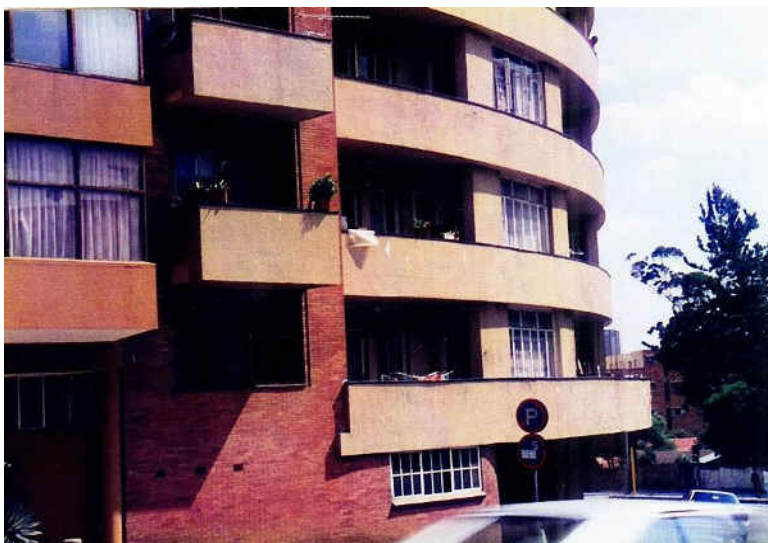
Fig. 346 Royal Crescent (right) on the curve; Reading Court (left) which is a major example of a Modern Movement building, restoration work is needed (Photograph: Clive Chipkin)
