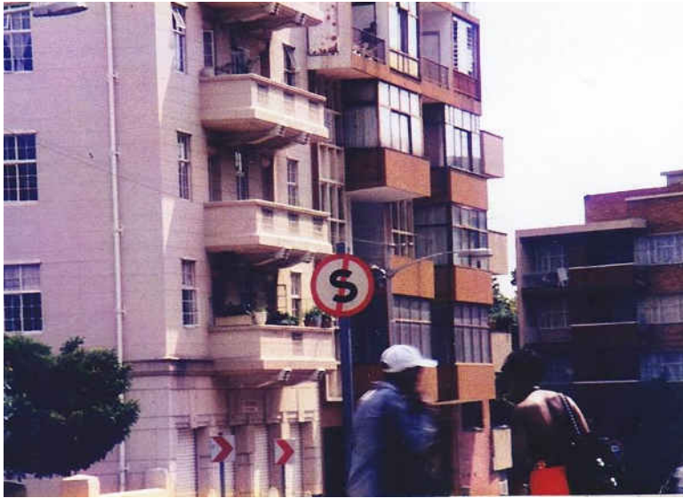
Fig. 345 Ridge View Corner Bantek Street (left); Reading Court (right), Ridge View is a setback flat block from the 1920's which creates a memorable urban space (Photograph: Clive Chipkin)
