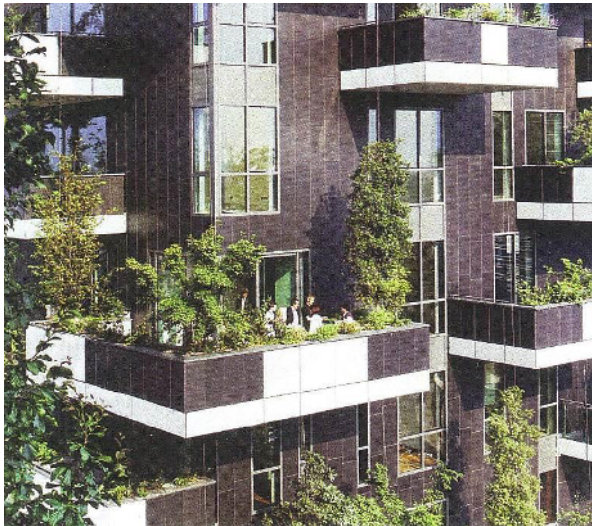
Fig. 329 Balconies as plant areas. Bosco Verticale, Milan. Architect: Boeri Studio. (Source: Earthworks journal, Issue 24/2015)
