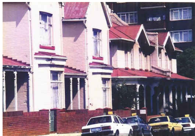
Fig. 342 & Fig. 343 Berea Fire Station 1910; adjacent architecture with reference to Victorian terraces of a decade earlier (Photographs: Clive Chipkin)
