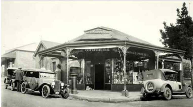
Fig. 322 Corner shop built in 1905 along 7th Street and 3rd Avenue in Melville, cast iron columns supporting the roof structure (Source: Museum Africa)
