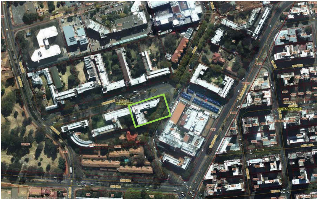
Fig. 349 Princess Place indicated in green_high density apartment block. Precinct with green-belt and private gardens (Source: GIS map, City of Johannesburg)
