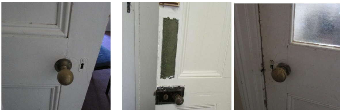
Images 24 – 26: Original door fittings: brass knobs, locks on rooms on right and brass knob on door to veranda.
