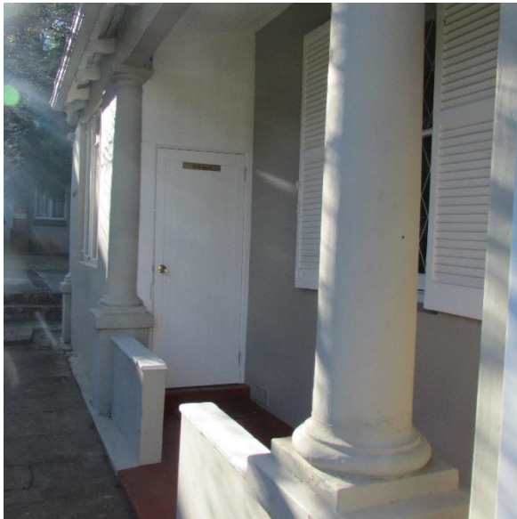
Image 11: portion of original veranda on east side with “Dr I Appelt” name plate on door. Two portions of the original veranda exists: on the south side (image 10) and on the east side (image 11)
